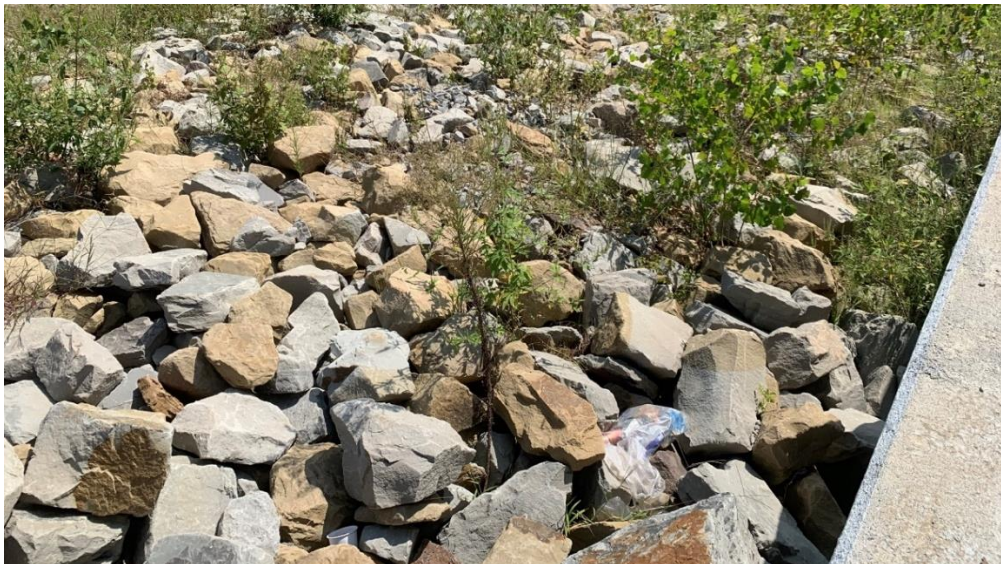
Figure 4: Rip rap along bridge abutment in good condition, taken near Laverne, Oklahoma, in 2020.
