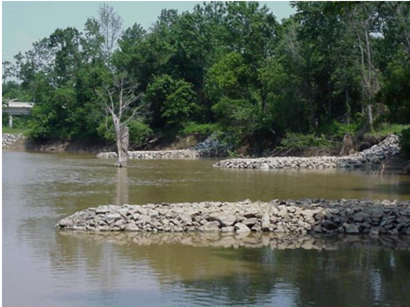
Figure 5: Image of bendway weirs (Thornton et al. 2007).
