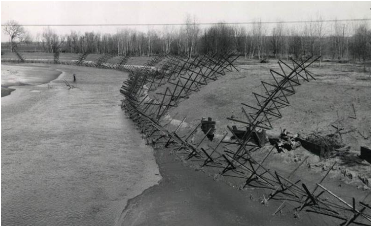
Figure 1. Example of a Kellner jetty field on the Washita River in Oklahoma, taken in 1950 (Lewis 2020).
