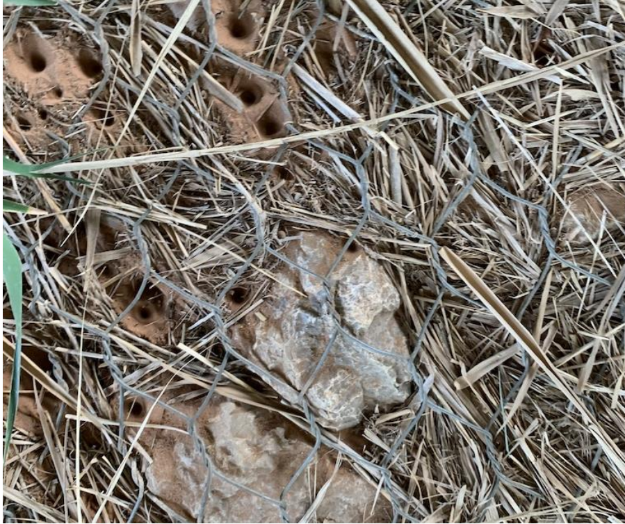
Figure 66: Sunken gabion baskets at site 26
