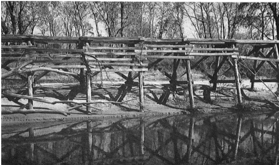
Figure 3. Image of pile diversion on the Arkansas River north of Bixby, Oklahoma, taken in 1988 (Harp and Thomas 1989).
