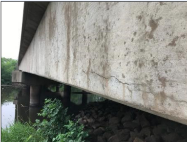
Cracks in concrete indicate potential corrosion in internal reinforcing rebars.
