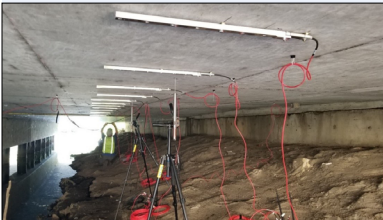
Strain gauges measure the load distribution across the width of the bridge.
