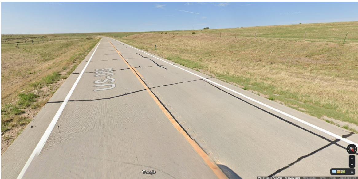
Figure 2.25 Current condition of US 385
