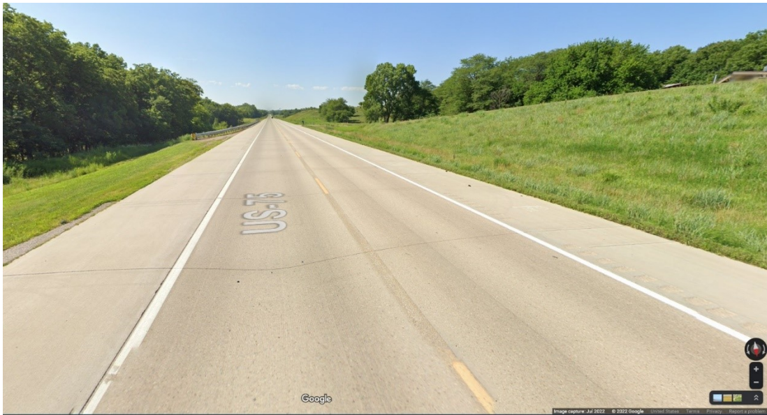
Figure 2.15 Current condition of US 75
