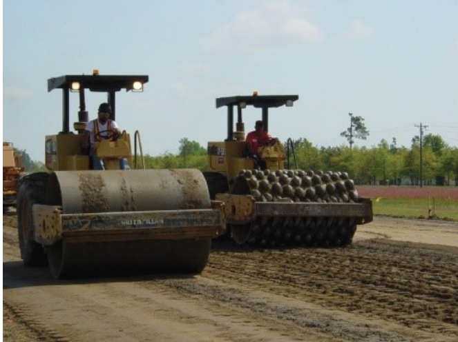
Figure 1.6 Final compaction (4)
