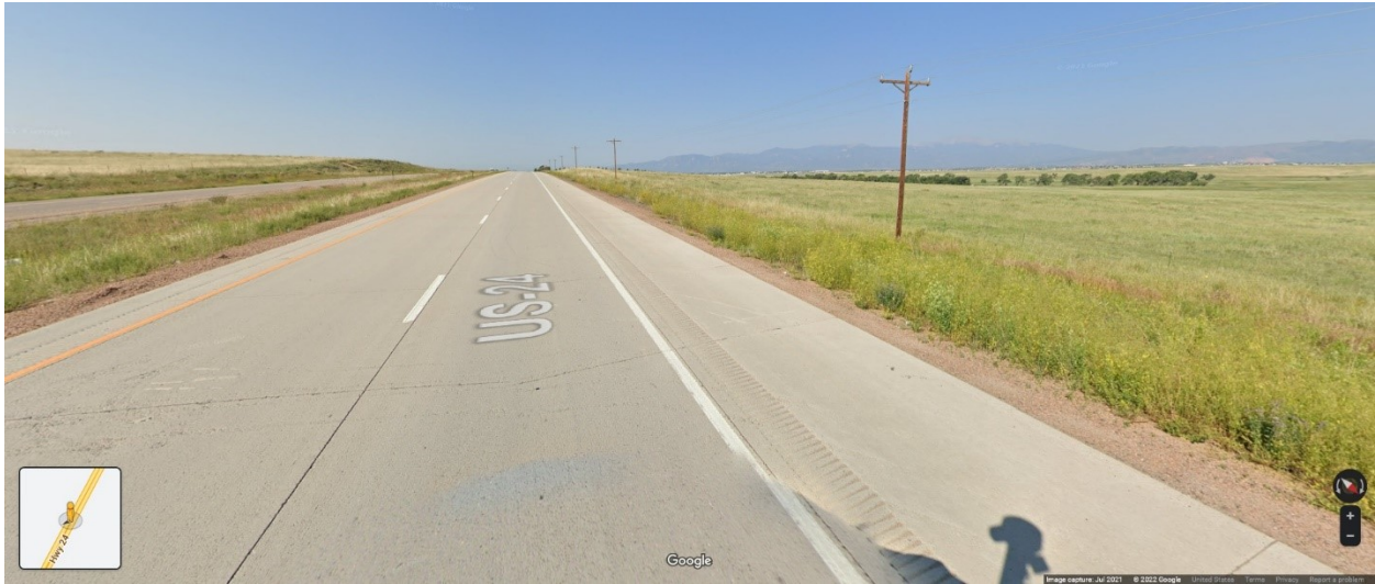
Figure 2.29 Current condition of US 24
