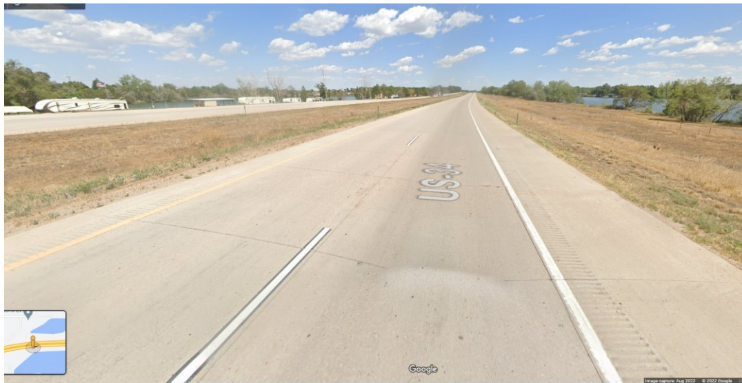
Figure 2.27 Current condition of US 34
