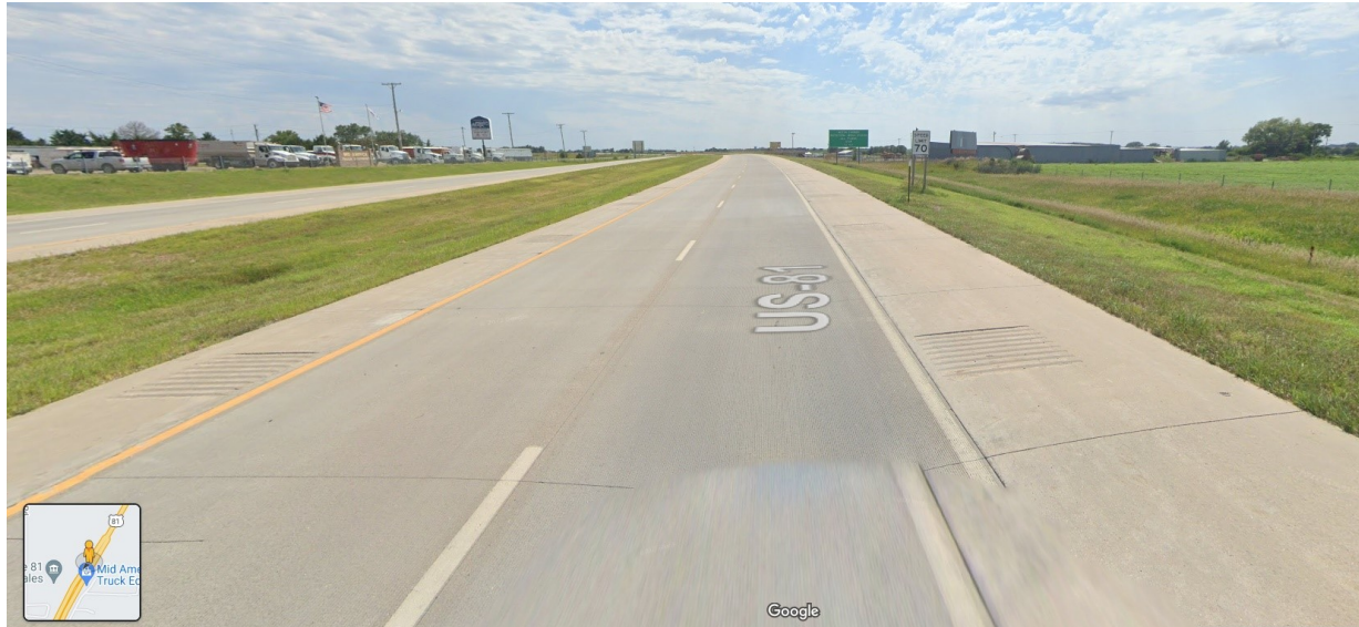
Figure 2.20 Current condition of US 81
