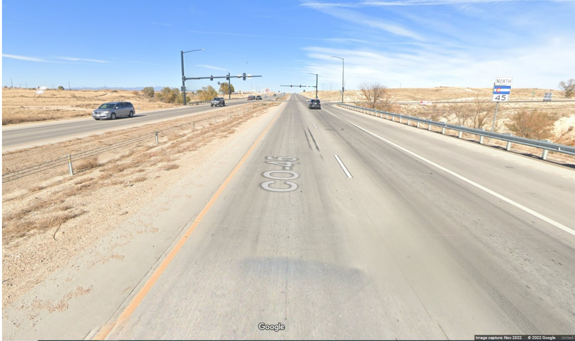
Figure 2.31 Current condition of SH 45
