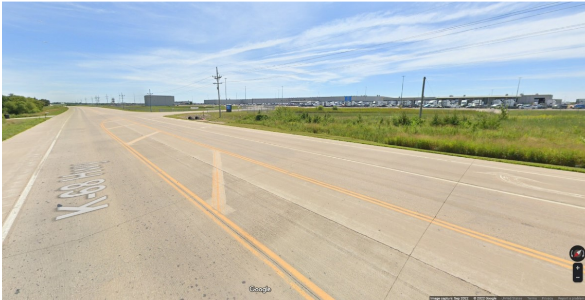
Figure 2.18 Current condition of K-68
