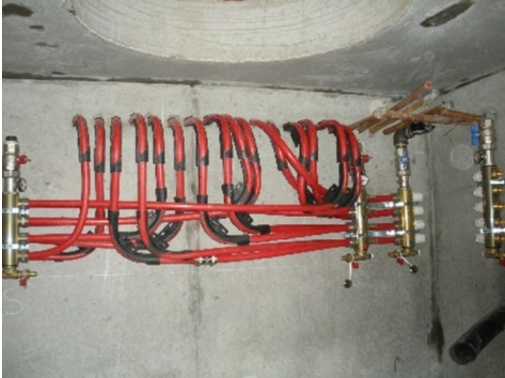
Figure 2. Control Center Interior
