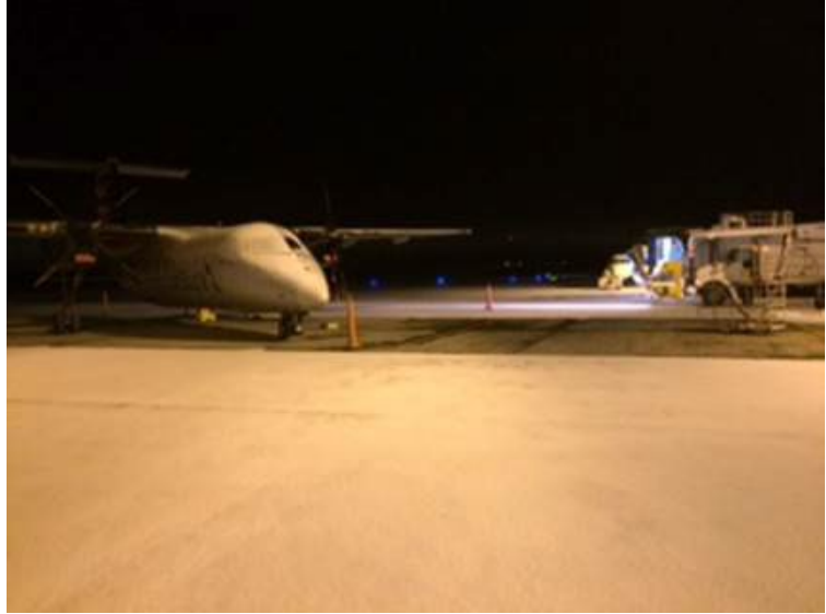
Figure D-3. System in operation following a snow event: Heated pedestrian walkway in the foreground; heated slab to the right; unheated area in the background (left photo); Heated slab under and to the right of the aircraft; unheated apron is in the foreground (right photo)
