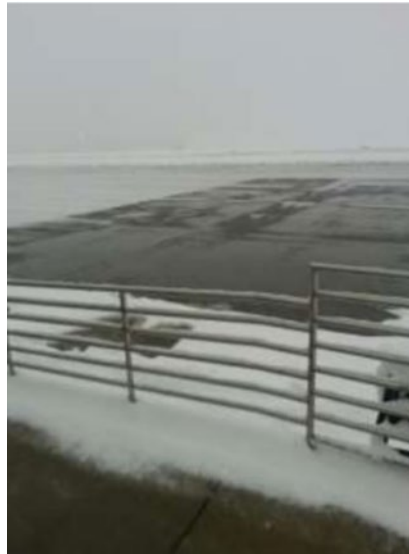
Figure 10. Walkway and Apron Pavement in Test Area—Ice and Snow Free
