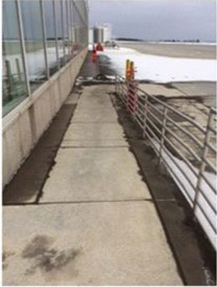
Figure D-3. System in operation following a snow event: Heated pedestrian walkway in the foreground; heated slab to the right; unheated area in the background (left photo); Heated slab under and to the right of the aircraft; unheated apron is in the foreground (right photo)
