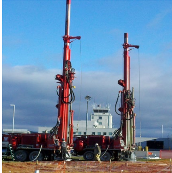
Figure 5. Geothermal Well Drilling
