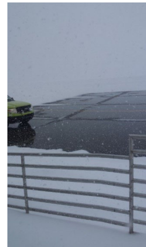
Figure D-5. System in Operation During a Snow Event Falling at the Unusually High Rate of 4–6 inches per hour (Note the system is slightly behind, as expected in such a rare event. However, the slush as seen by the footprints shows the system is operating and will, in fact, clear the area as soon as the downfall lets up.)
