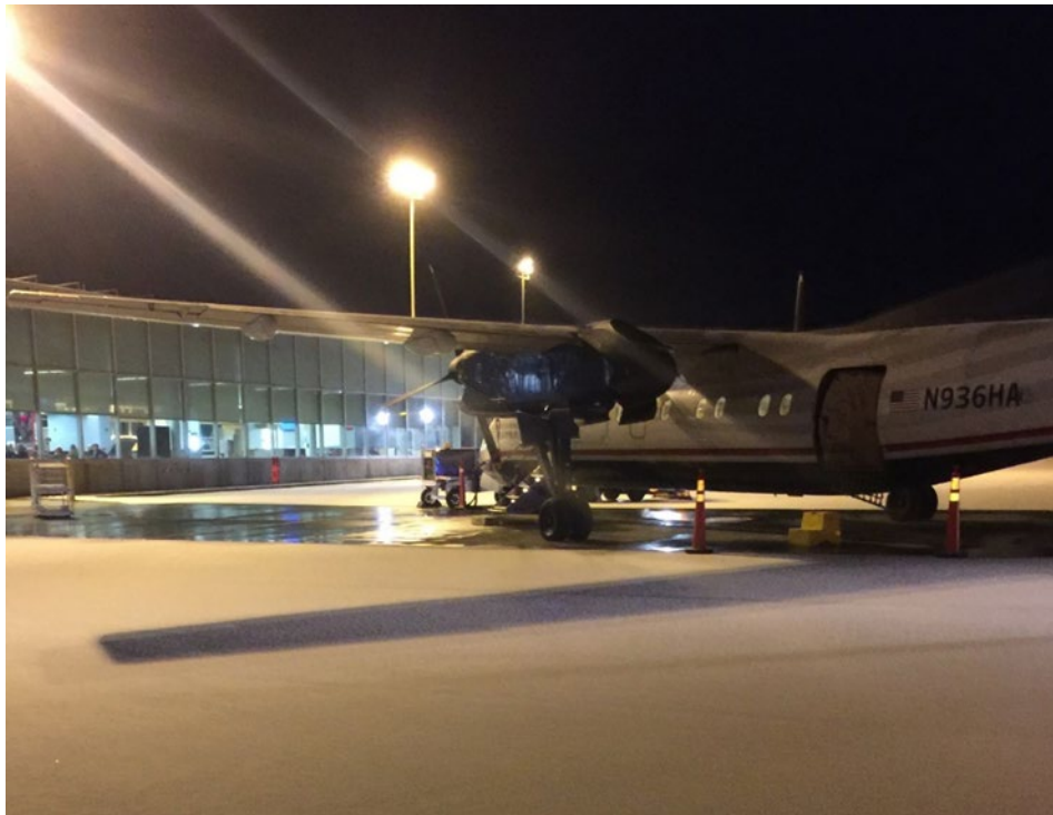
Figure D-4. System in Operation Following a Snow Event 12/29/2016 (Heated slab can be seen under and to the left of the aircraft. Unheated apron is in the foreground.)
