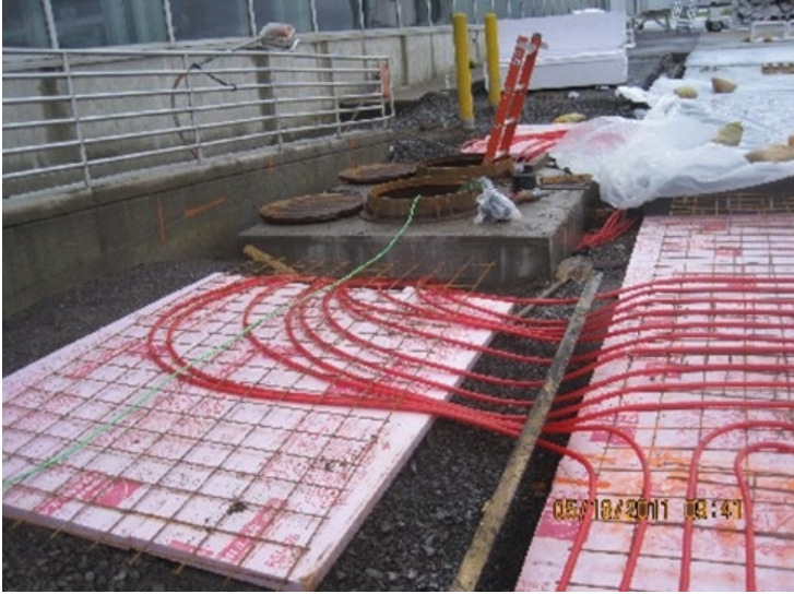
Figure 1. Control Center Exterior
