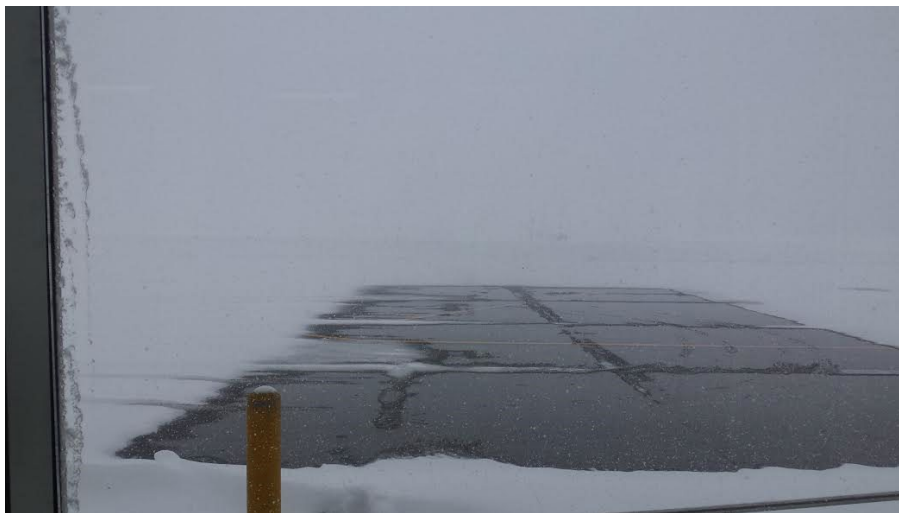
Figure D-5. System in Operation During a Snow Event Falling at the Unusually High Rate of 4–6 inches per hour (Note the system is slightly behind, as expected in such a rare event. However, the slush as seen by the footprints shows the system is operating and will, in fact, clear the area as soon as the downfall lets up.)
