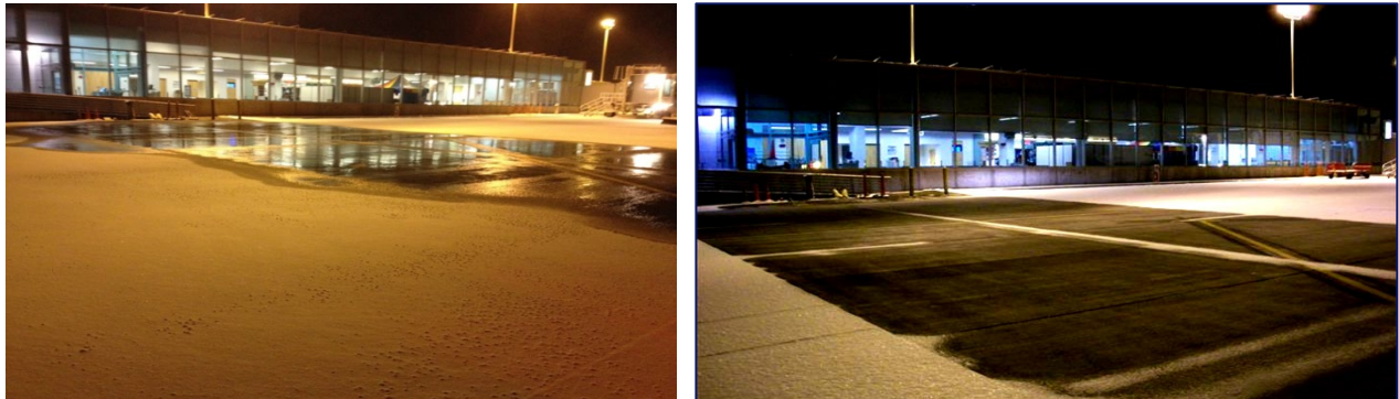
Figure D-2. A preliminary test of just the radiant heating portion of the system was conducted near the end of the winter of 2011–12 and proved successful in all aspects of the system. (Note the cleared area of the tarmac). At that time, since the geothermal field had not yet been installed, heat to the system was provided by a temporary gas boiler.
