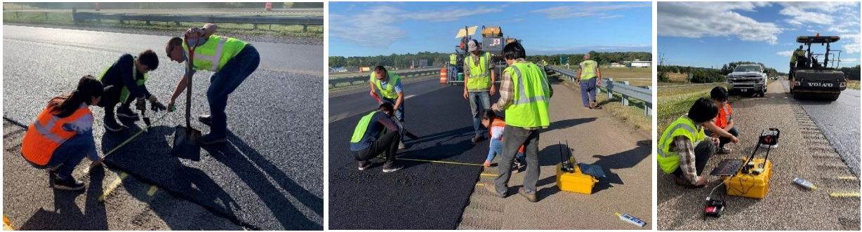
Figure 8. SmartRock installation and data collection in the Indiana project.
