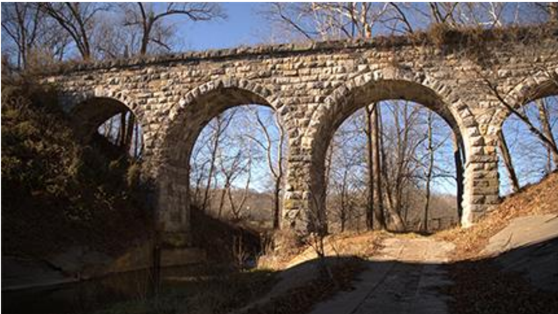
Figure 3. Stone Masonry Arch, Built as a Railroad Bridge, 1874 (Augusta County Structure No. 6997)
