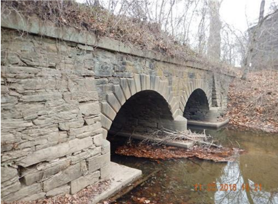
Figure 4. Stone Masonry Arch, Originally Built as a Canal Viaduct, 1835 (Nelson County Structure No. 6070). Note the particularly fine finishing of the voussoirs.
