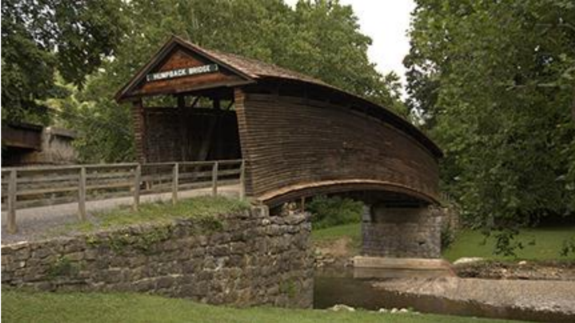
Figure 2. Stone Masonry Abutments and Stone Masonry Approaches on Humpback Bridge, 1857 (Alleghany County Structure No. 9007)
