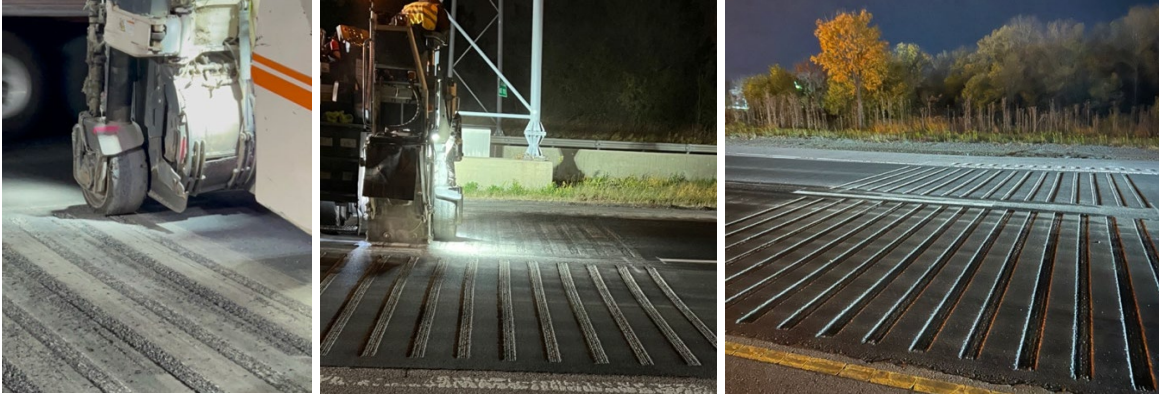
Figure 2. Photo. Construction of 2022 rumble strips.
