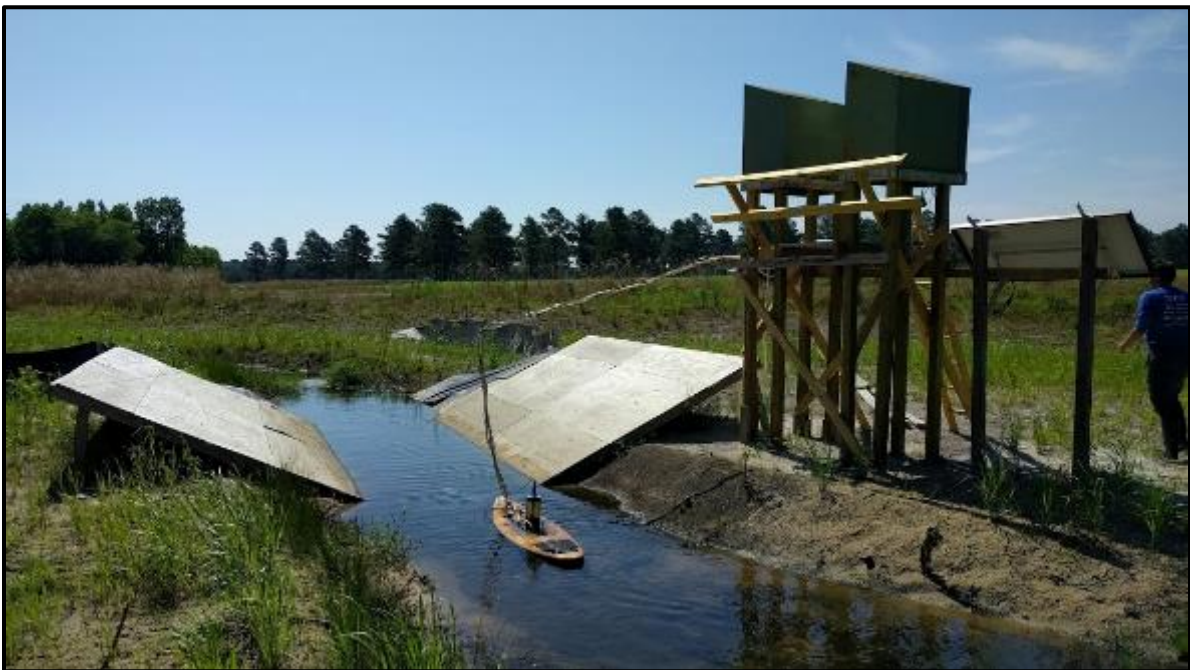
Figure 6. CLMD station with raised platform
