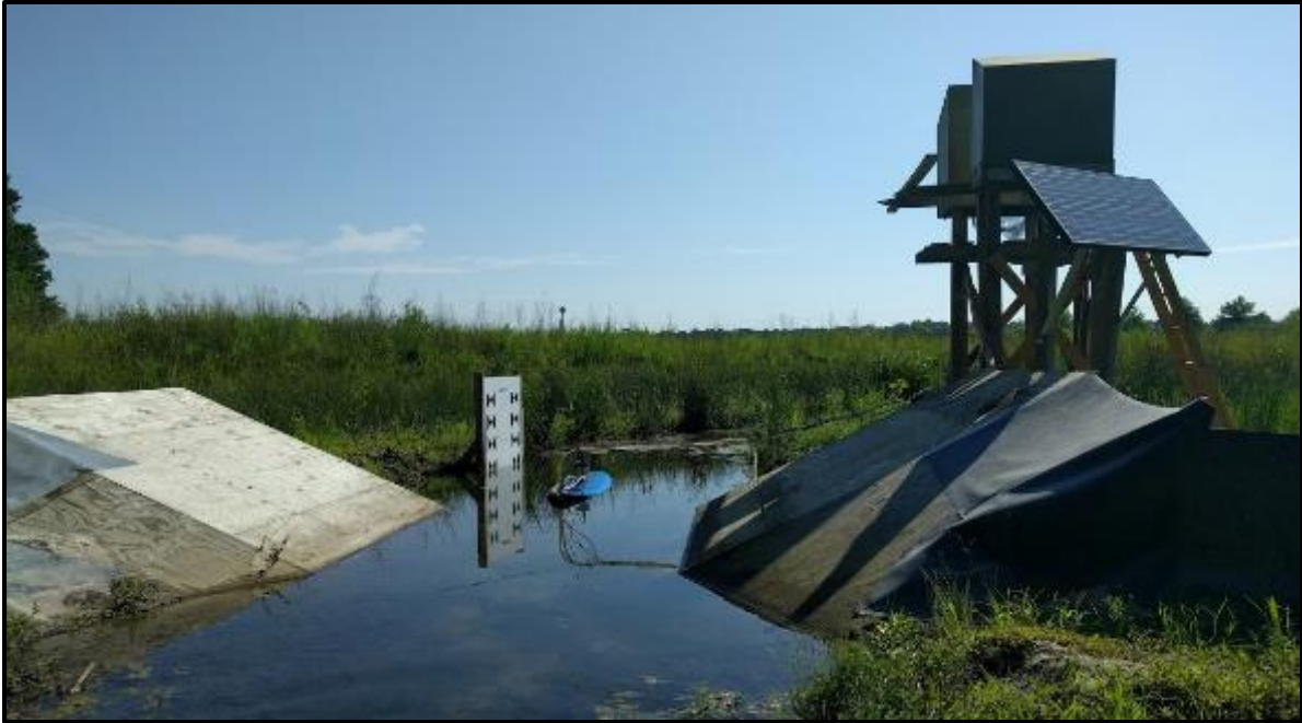
Figure 5. CLUP station with raised platform
