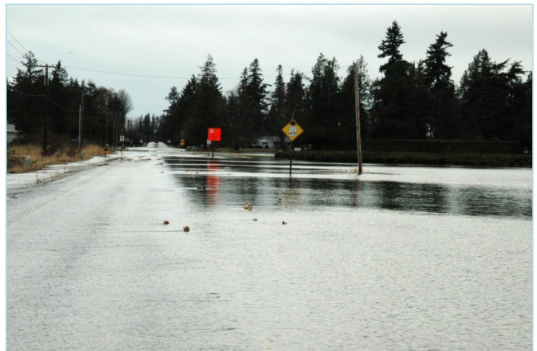
SR 11 during the 2009 Flood Event
