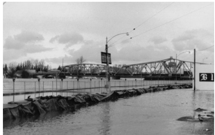
Sandbag Revetment during the 1980 flood event
