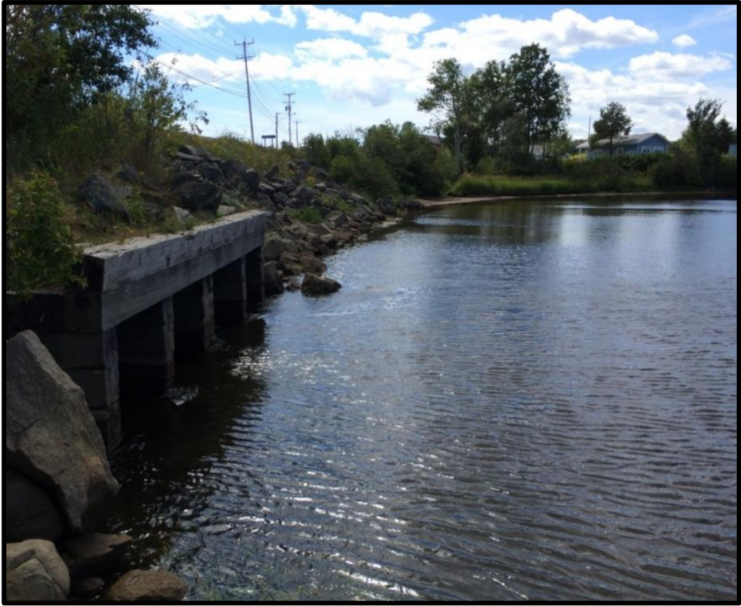
Figure 4: Photo of Dyke Bridge, Upstream Side. 8
