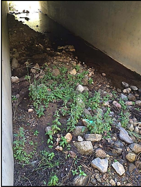
Figure 6: Sediment Deposition Inside the US 34 Culvert, October 2015 (left) and View of Culvert Inlet Showing Wingwall (right). Photograph provided courtesy of FHWA.
