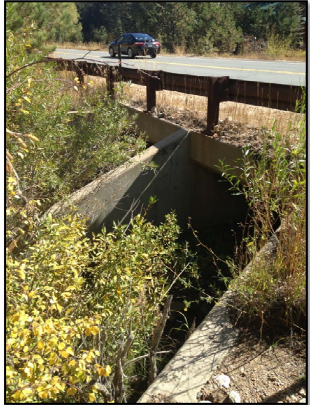
Figure 6: Sediment Deposition Inside the US 34 Culvert, October 2015 (left) and View of Culvert Inlet Showing Wingwall (right). Photograph provided courtesy of FHWA.
