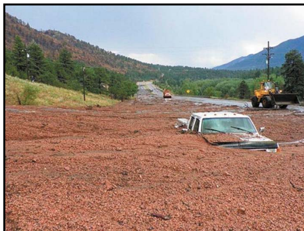
Figure 5: Post-wildfire debris flows on US 24 near Waldo Canyon (2013). Photograph courtesy of the Colorado Department of Transportation.
