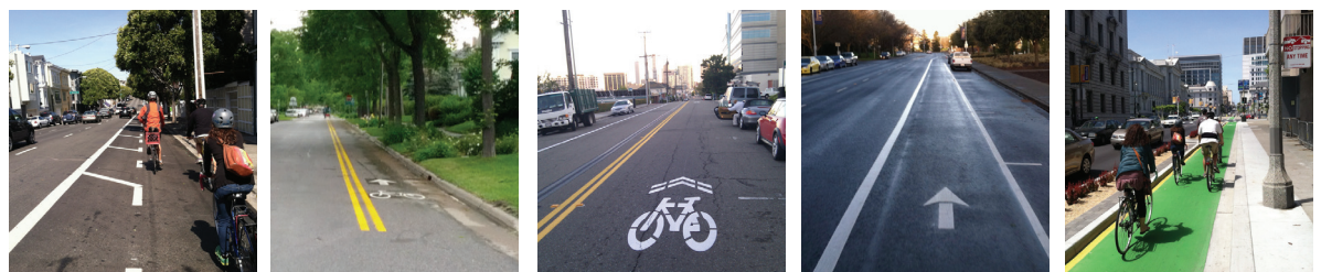
Figure 1. Examples of bicycle infrastructure. From left to right: buffered bicycle lane, contraflow bicycle lane, bicycle route marked by a sharrow, conventional bicycle lane, and a physically separated bicycle lane.
