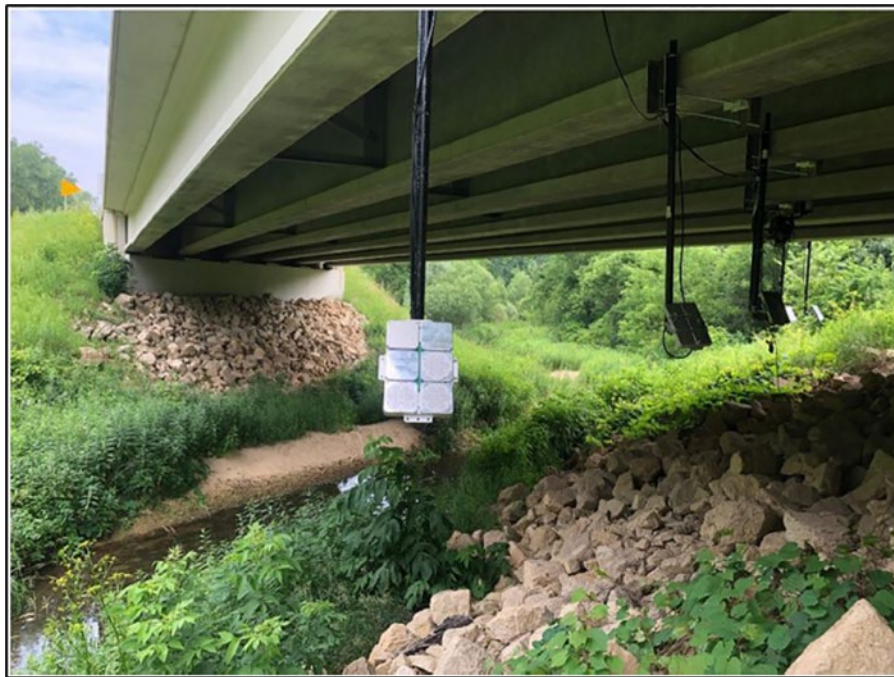
Figure 5. NRG Bat Deterrent System arrangement at bridge. (Photo by Justin Dahlberg used with permission from Bektas et al. 2021)
