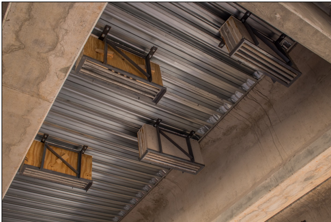
Figure 8. Bat roosts installed on a bridge in Arizona as an example of those installed on a bridge in NC for gray bats. (Photo taken by Melina Zuniga and used with permission from Cronkite News)
