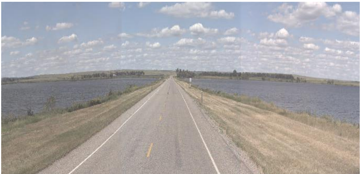
Figure 10: LEFT, CENTER, AND RIGHT IMAGE ROADWAY EVALUATION SYSTEM JCT US 83 NORTH OF HERREID
