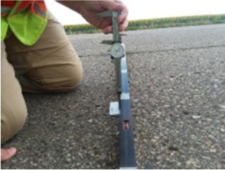
Figure 5: RUT MEASUREMENTS WITH LEVEL AND CALIPER
