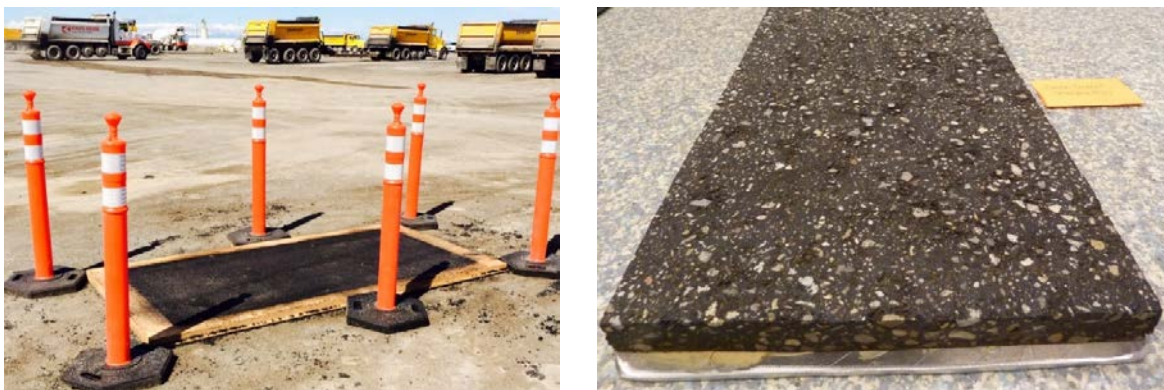
Figure 2.1 Pavement sample during construction (left) and after preparation (right)
