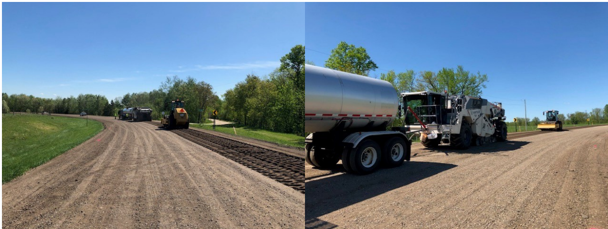
Figure 2-1 SFDR Construction on Beltrami CSAH 4.
