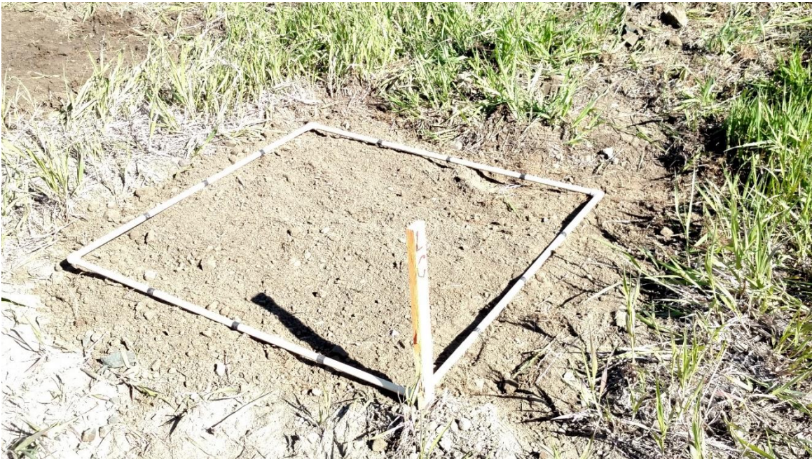
Figure 13. Preparation of 1 m 2 experimental plot, simulating post-construction revegetation. This plot was hand dug, and the soil was mixed to a depth of 15–20 cm (6–8 in) and smoothed level. A perennial seed mix was broadcast over the soil and gently tamped by hand to give seeds good soil contact. This test plot was located at the Bozeman Pass test site.
