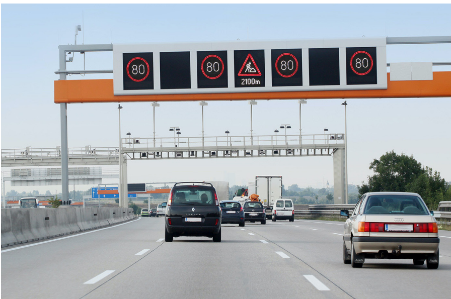
Figure 2. An overhead sign communicating variable speed limits on an Austrian highway ( www.asfinag.at )
