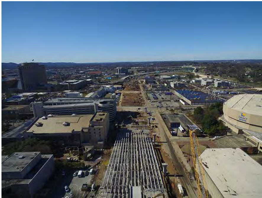
Figure 2. Interstate reconstruction in February 2019 (source: ALDOT)
