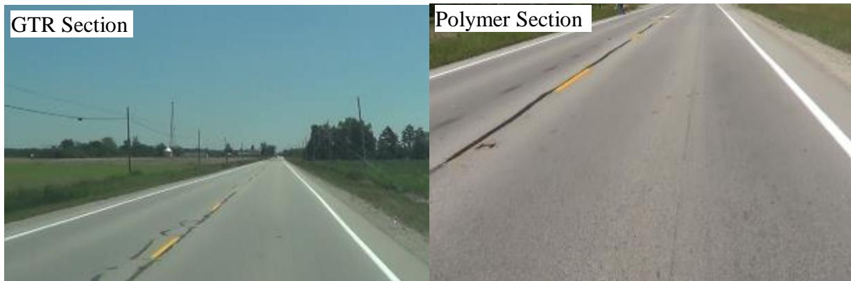
Figure 3.6 Pictures of GTR and Polymer Modified Pavement Sections at US 6 After 6 Years of Service
