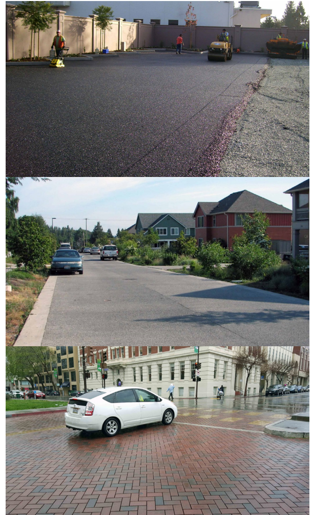
Figure 1. Three examples of permeable pavements, from top to bottom: porous asphalt, pervious concrete, and permeable interlocking concrete pavement
