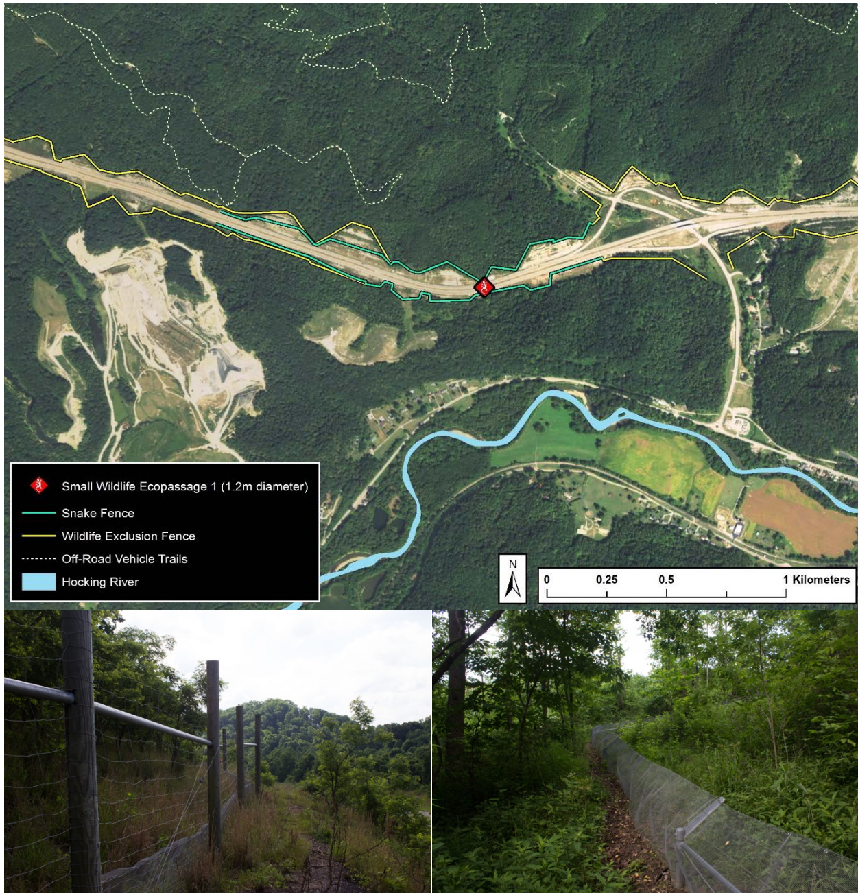
Figure 7-2. Snake exclusion fence along the U.S. 33 Nelsonville Bypass, Hocking County, Ohio. Top: map showing extent of snake exclusion fence, Bottom Left: snake fence attached to the 8-ft. tall wildlife exclusion fence, Bottom Right: snake fence installed independently from the 8-ft. tall wildlife exclusion fence.
