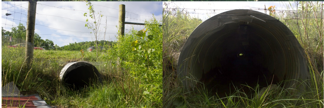
Figure 7-3. Ecopassages (i.e. wildlife crossing structures) along the U.S. 33 segment of the Nelsonville Bypass. Top: ecopassages locations along the U.S. 33 Nelsonville Bypass, Bottom Left: Small Wildlife Ecopassage 1 entrance integrated into snake fence, Bottom Right: a look inside the ecopassages reveals a long, dark tunnel.
