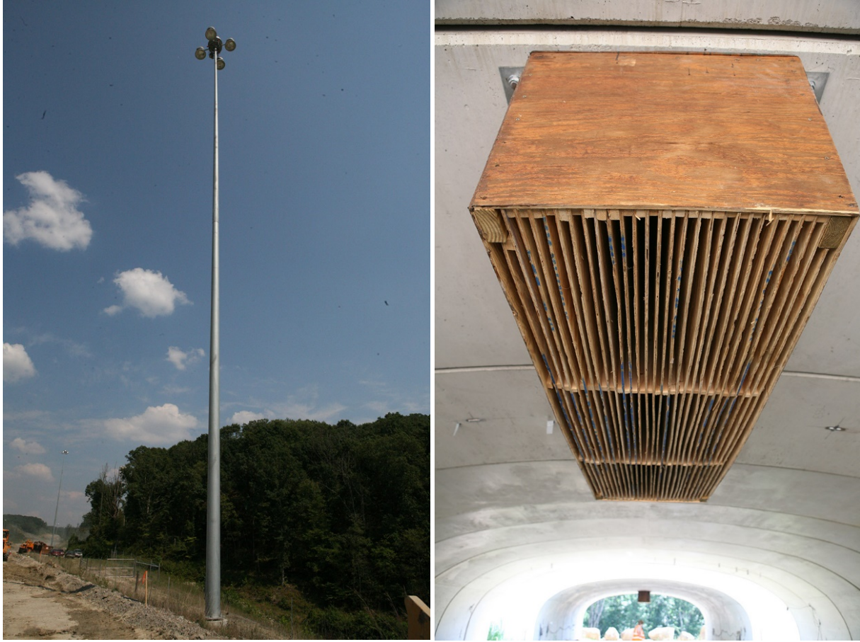
Figure 6-1. Image of high-mast lighting (left) and lattice style bat roosting boxes (right) employed along the U.S. 33 Nelsonville Bypass, Athens and Hocking Counties, Ohio. High-mast lighting is designed to lure bats away from the flow of traffic and bat roosting boxes are intended to replace habitats removed during construction.
