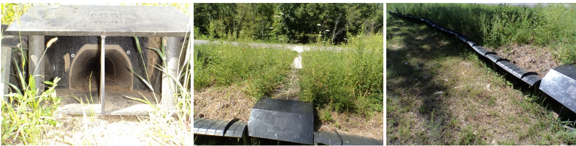
Figure 5-4. Images of the ecopassage opening (left), ecopassage crossing under the road, perforations in the top can be seen (middle), and curved plastic fencing (right) in place along State Route 78, Athens County, Ohio.
