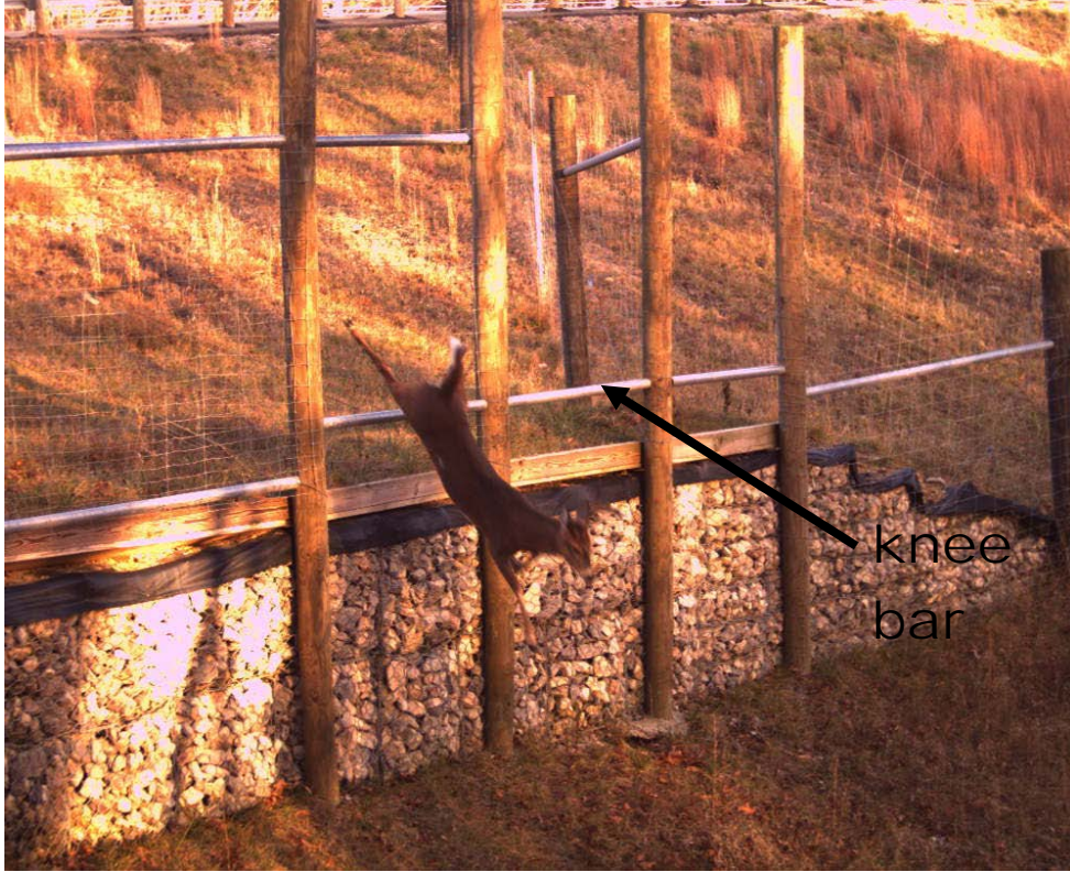
Figure 2-16. White-tailed Deer exiting the U.S. 33 Nelsonville Bypass right-of-way through a one-way jump out. This jump out does have a knee bar. This jump out has no apparent landing pad.
