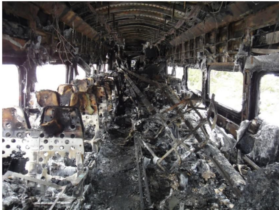
Figure 1. Interior of Valhalla, NY, passenger car after fire event (National Transportation Safety Board, 2017)
