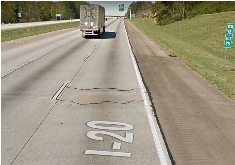
Figure 49 – A Patched Area of the Outside Lane at S3-b (Google Maps, 2017)
