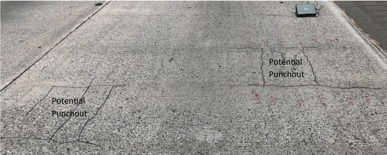
Figure 71 –Potential Punchout Sections at S5-c
