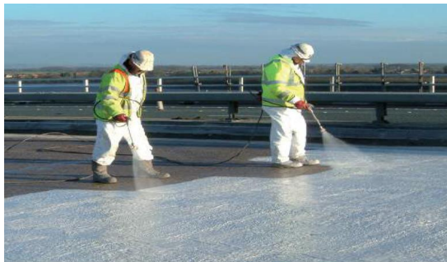
Fig. A.39 Applied-in-Place System (Strandquist, 2012)
