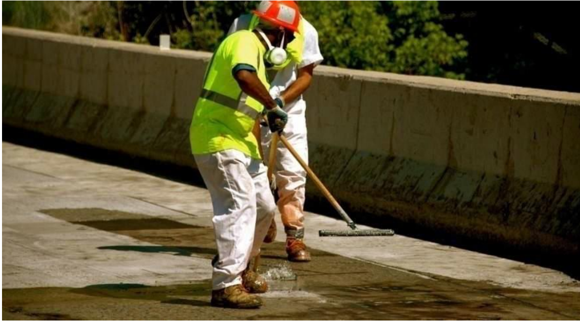
Fig. A.37 Application of Primer by Squeegeeing (Strandquist, 2012)
