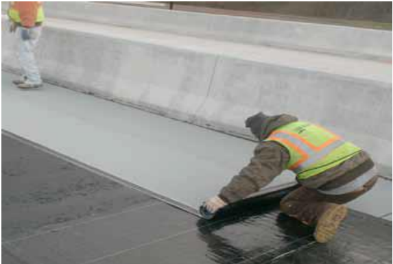
b) Laying out the Sheet Membrane
