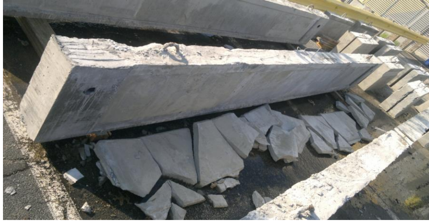
Fig. F.20 Set#4 Removed Grout After Testing for Re-Grouting
