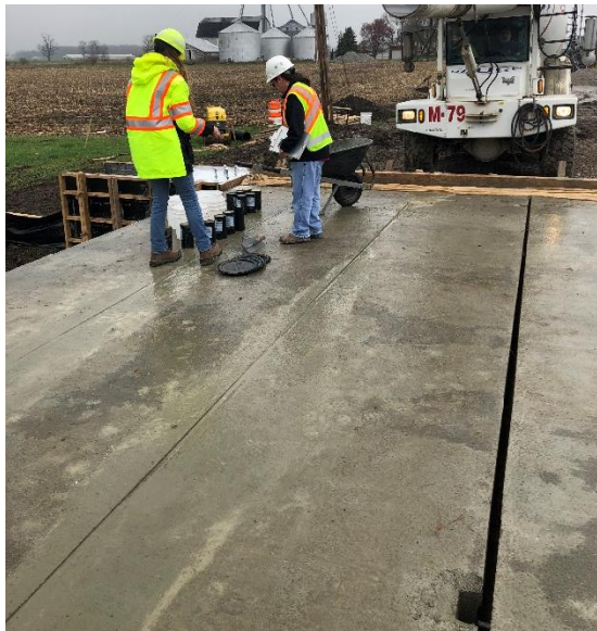
Fig. J.4 Joint Opening on Top Surface (Left); Key way Surface and Level Difference (Right)
