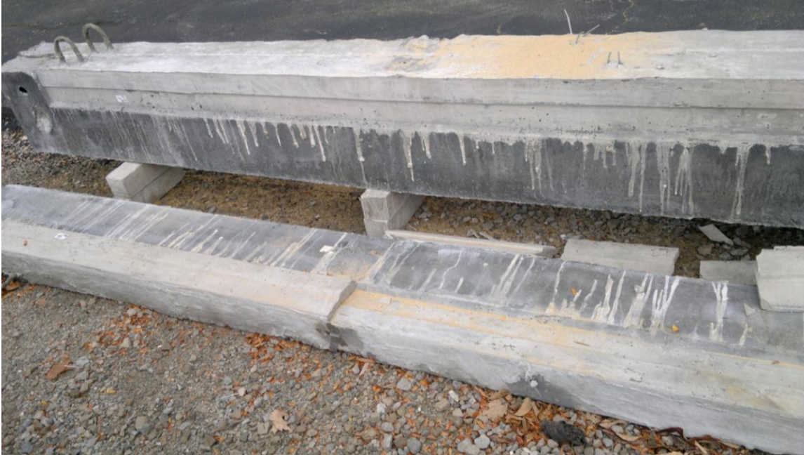
Fig. F.16 Set# 1 - Failed Joint After Testing
