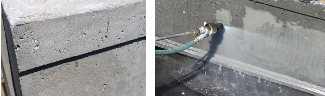
Fig. H.7 Sandblasted Surface Preparation for Eccentric Load Tests
