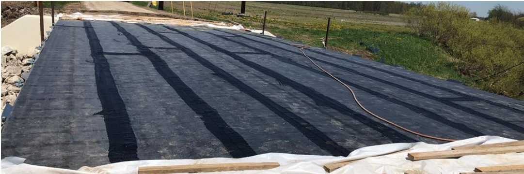
Fig. J.9 Deck Top Surface after Membrane Installation
