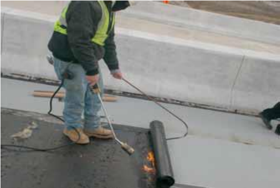
c) Heating the Sheet Membrane with a Torch
