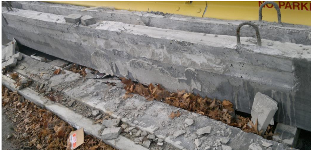
Fig. F.17 Set # 2 Failed Joint After Testing
