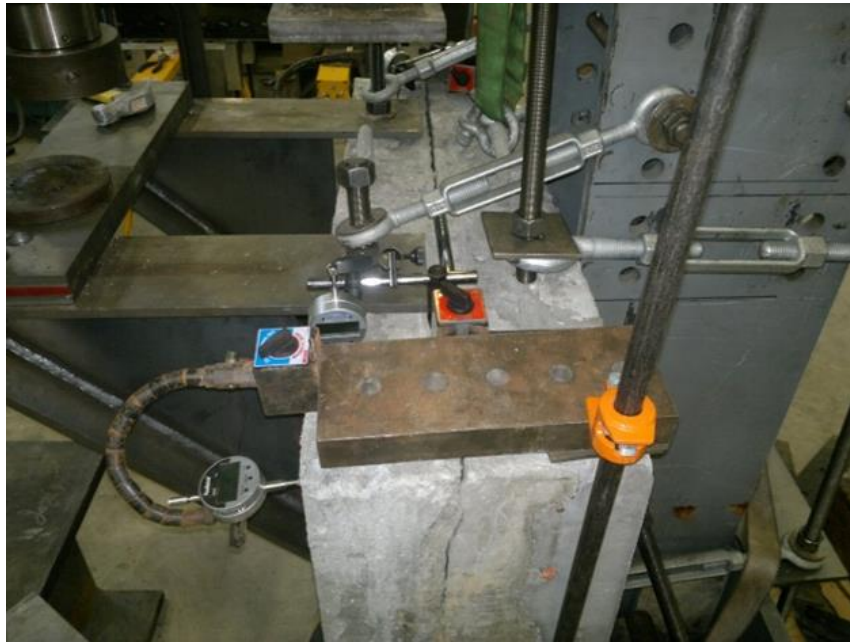
Fig. H.9 Failure of the Test Specimen with Kuhlman Grout under Self-Weight
