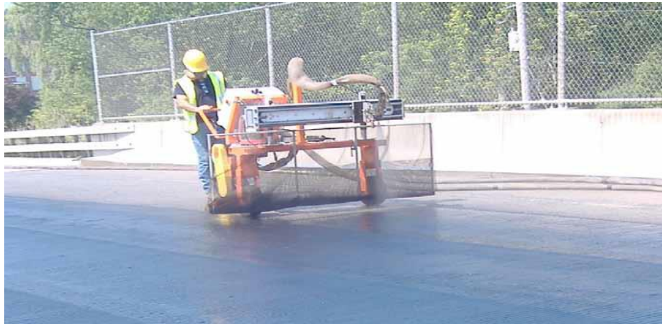
(b) Machine Spraying
