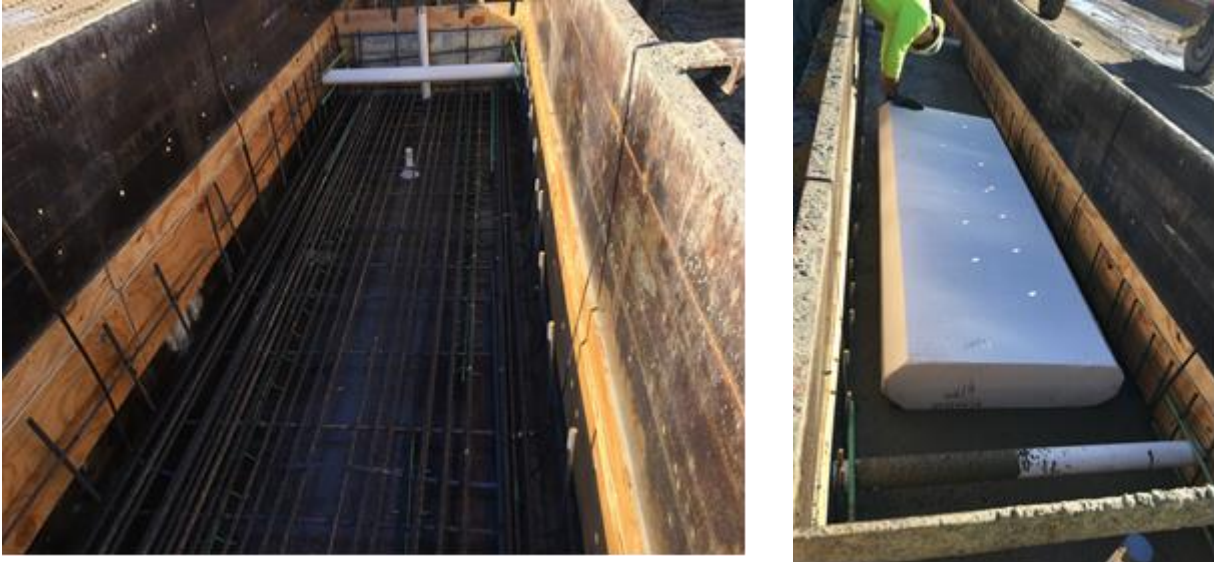
Fig. J.2 Key Way Profile Using Plywood (Left); Styrofoam Block for Creating a Void (Right)
