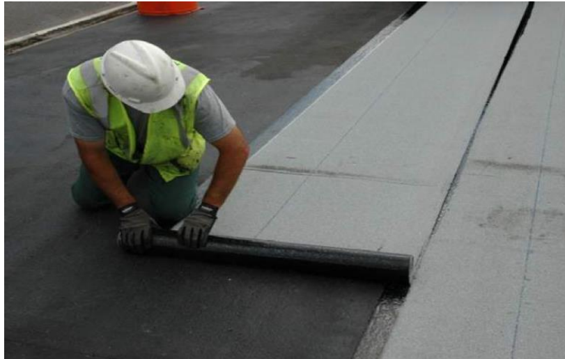
Fig. A.38 Preformed System Installation (Strandquist, 2012)
