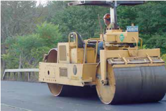
(f) Compacting the Hot Mix Asphalt
