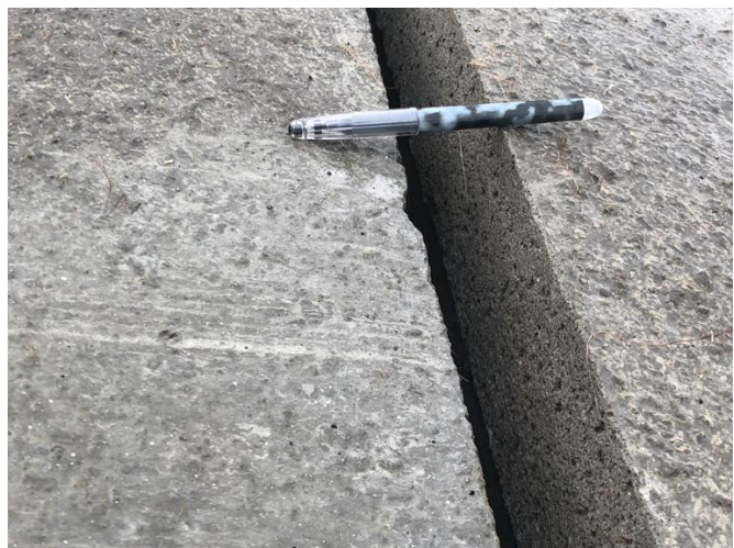
Fig. J.4 Joint Opening on Top Surface (Left); Key way Surface and Level Difference (Right)
