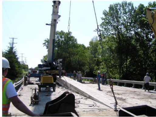
Fig. A.20 Removing the Deteriorated Beam
