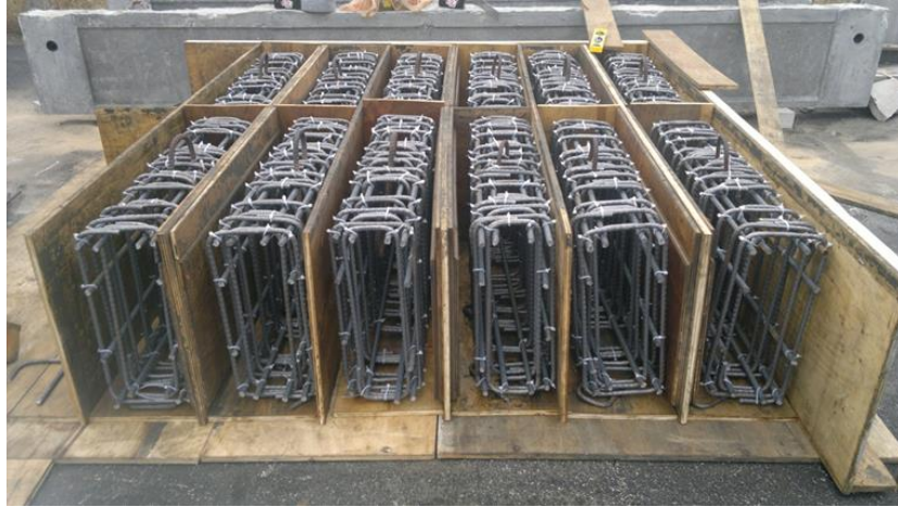
Fig. H.14 Formwork and Rebar for Set#2
