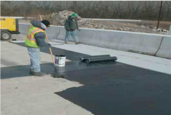
a) Application of Primer to the Concrete
