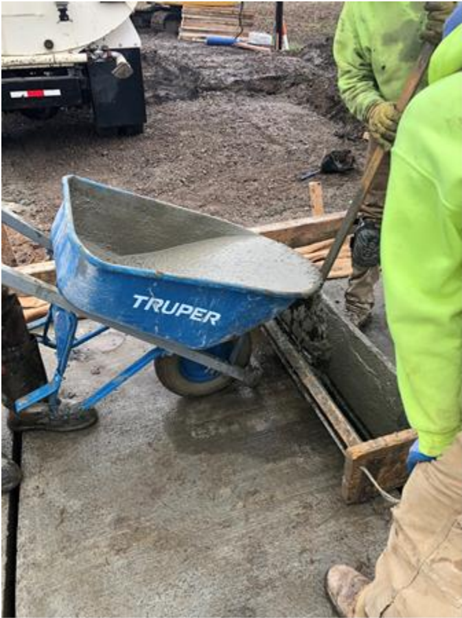
Fig. J.6 Grout Placement Through the Opening of the Key Way
