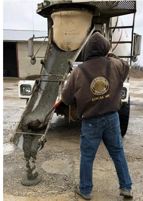
Fig. J.3 Trial Grout – Note the Spread of the Grout (Left); the Grout Consistency (Right)
