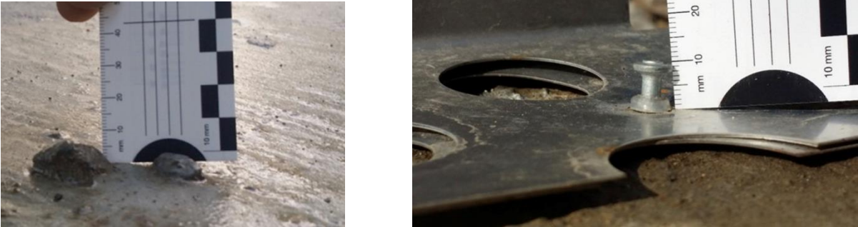
Fig. C.6 Protrusions Documented Just Prior to Laying the Waterproofing Membrane
