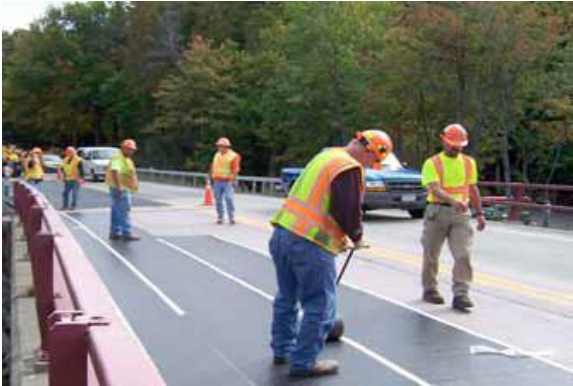
d) Sealing the Overlap Seams by a Hand Roller
