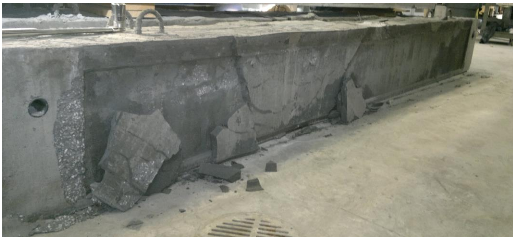
Fig. F.19 Set # 6 External Concrete Unit After Failure
