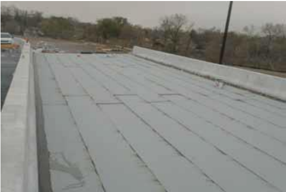
(e) Completed Membrane
