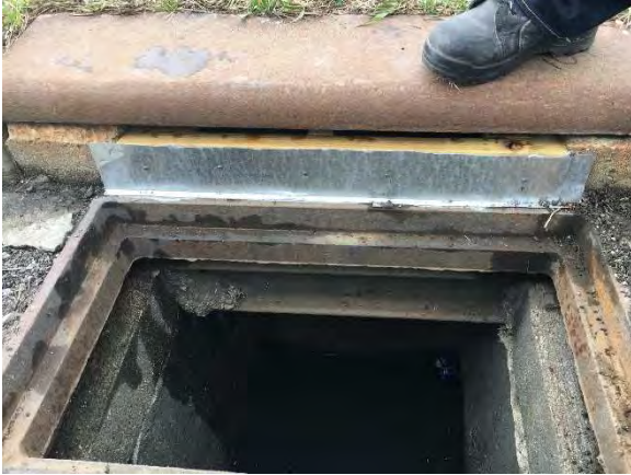
Catch basin in good condition
