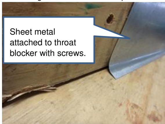
Figure 4-4: Throat block top view
