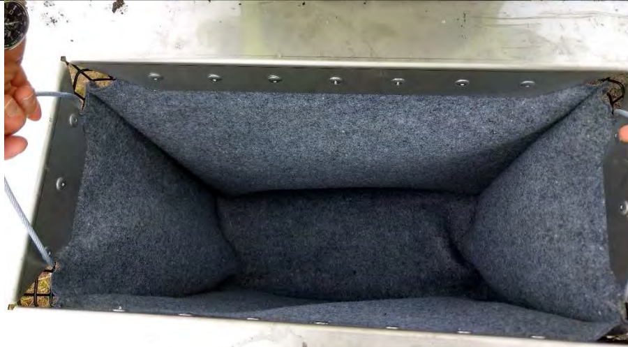
Basket was modified to fit within the catchbasin
