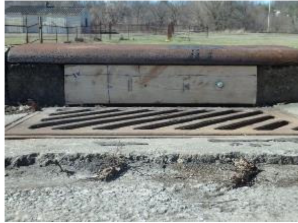
Figure 4-5: Throat block front view
