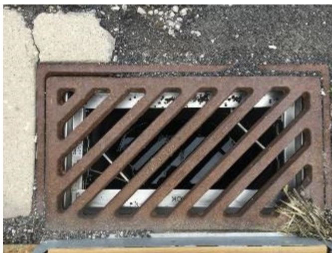
Figure 4-12: Typical Visual Inspection
