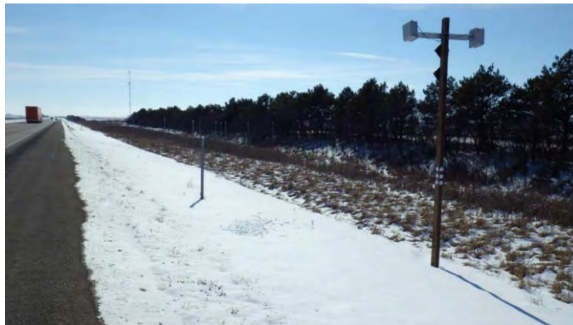
Figure 84. View of the I-35 site with the living snow fence protecting it
