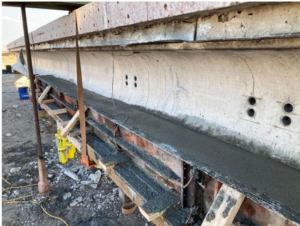
Figure 78. Placement of the SCC mix around the bottom flange
