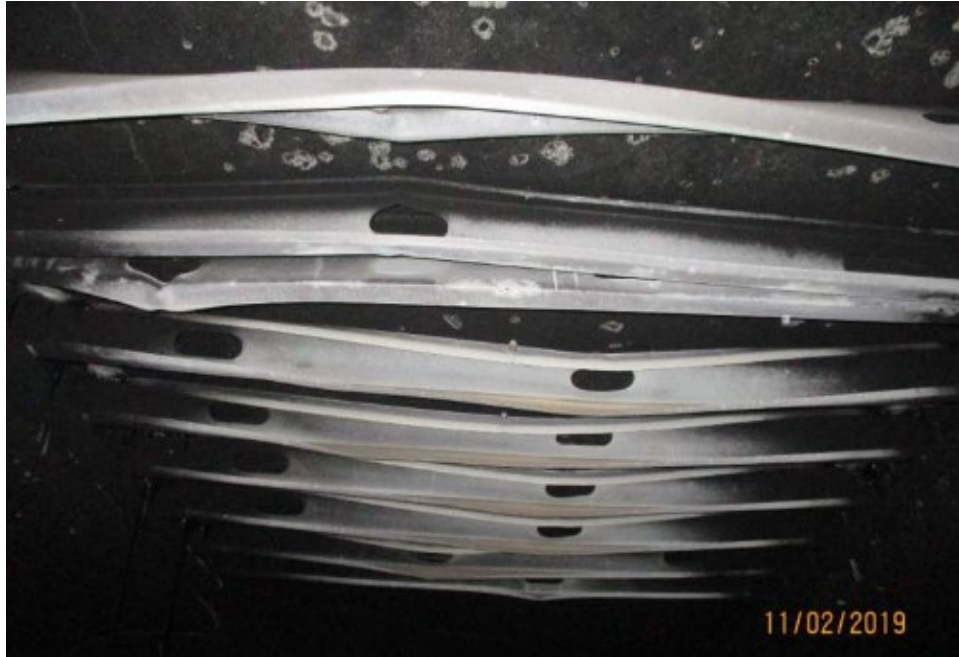
Figure 5. Melted polycarbonate formwork between Girders G and F
