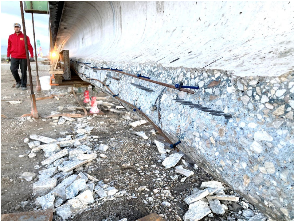
Figure 76. Tapcon concrete anchors and #3 rebar
