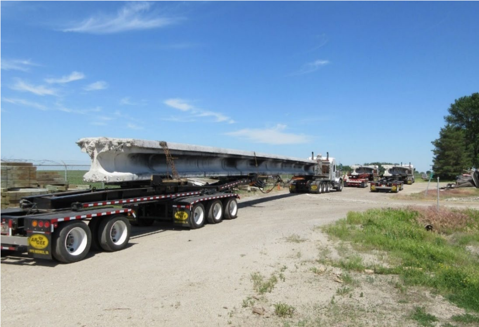
Figure 7. Girder transport from bridge site to Iowa DOT maintenance yard
