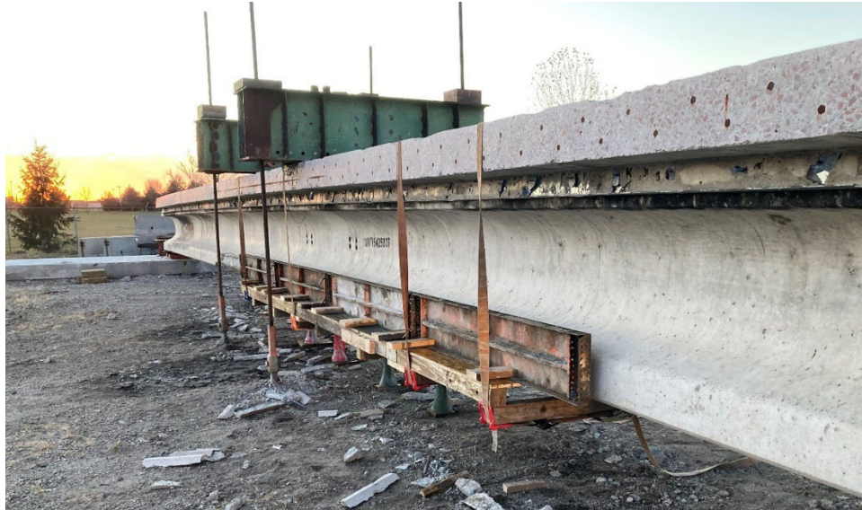
Figure 77. Steel and plywood formwork
