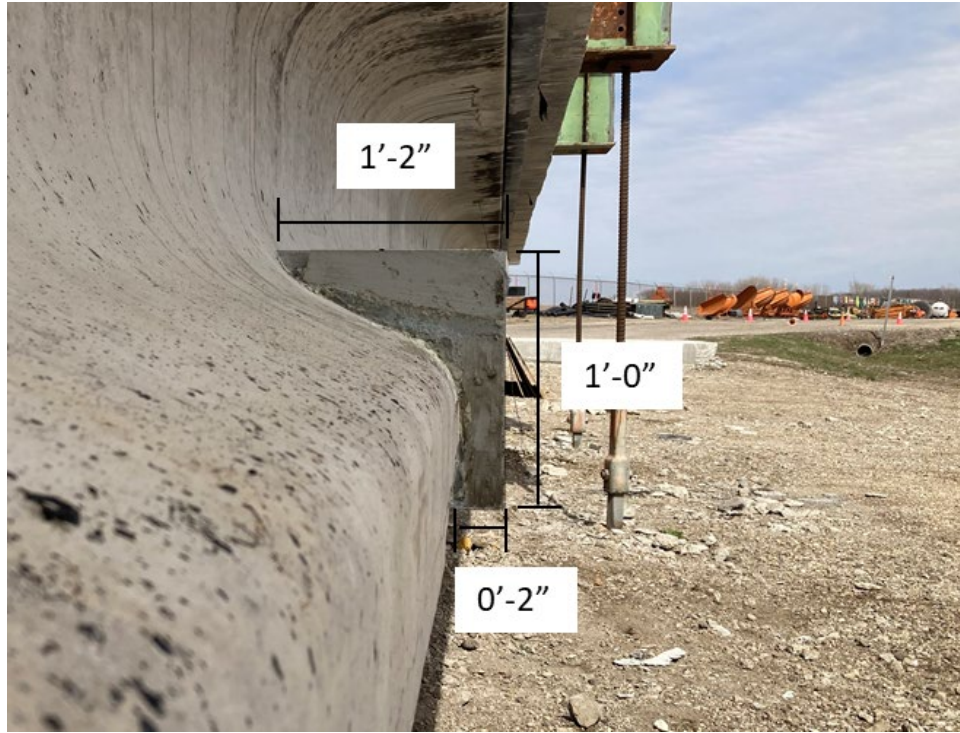
Figure 82. Dimensions of SCC and UHPC bottom flange repair
