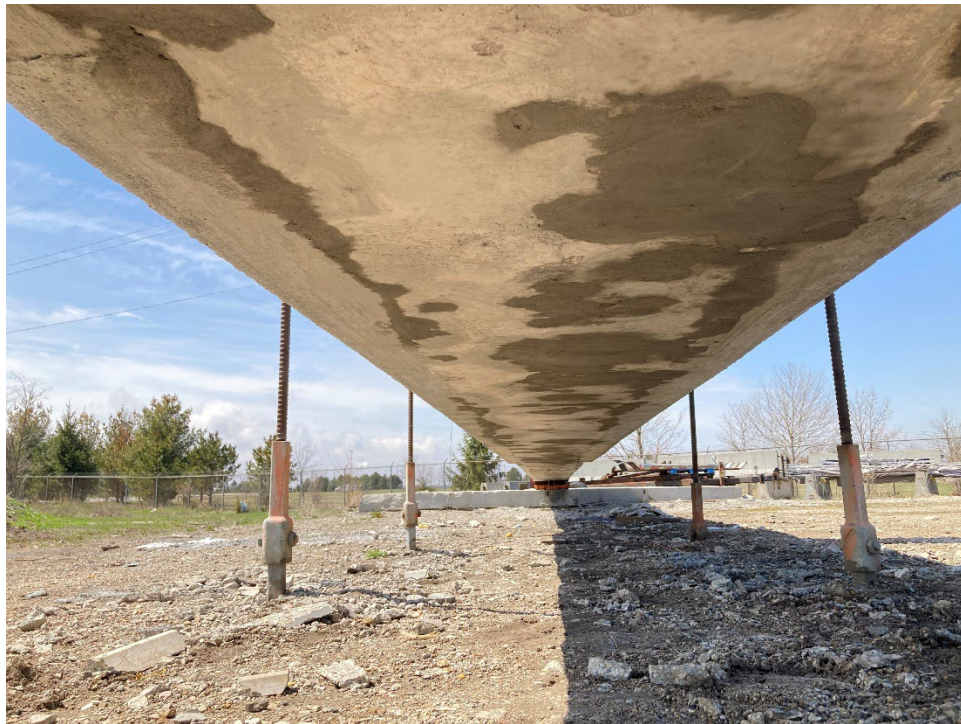
Figure 84. Bottom of girder spalls after repair mortar application
