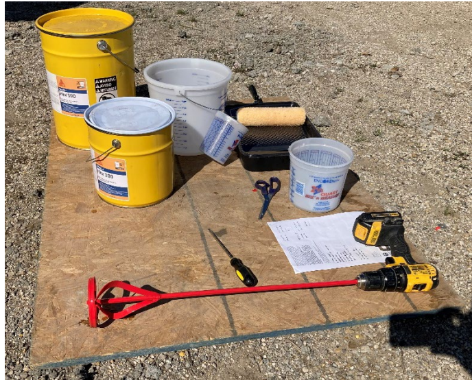
Figure 85. Preparation for mixing the FRP resin
