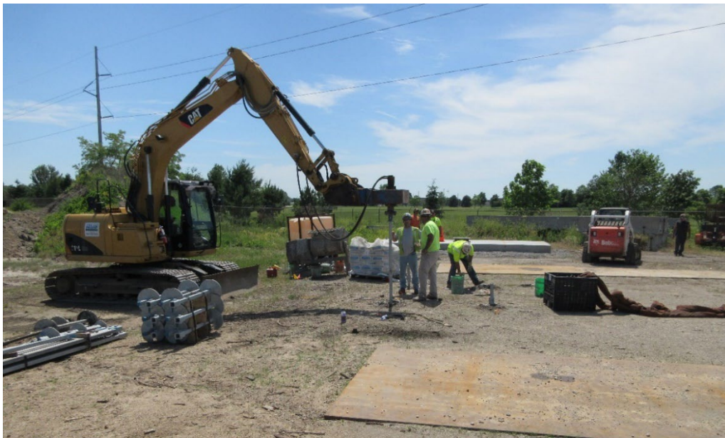
Figure 37. Installation of helical piles
