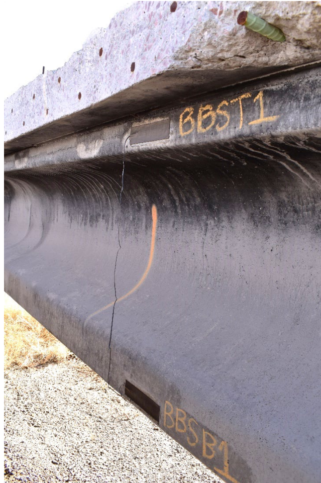
Figure 35. Girder B – Strain gauges at Section B bottom on south side
