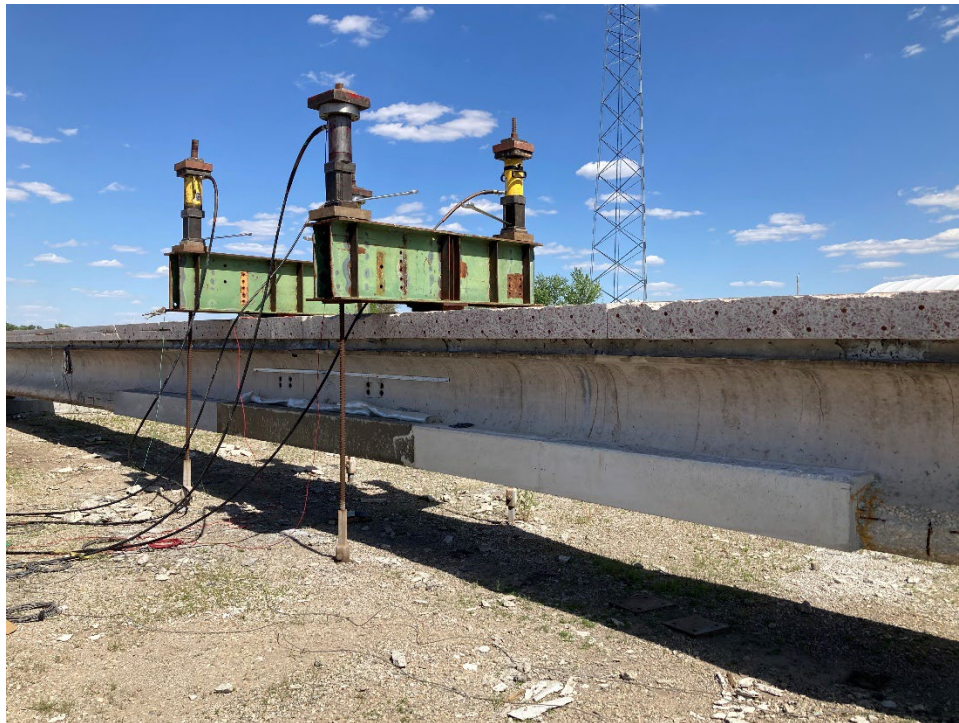
Figure 88. Load test of repaired girder
