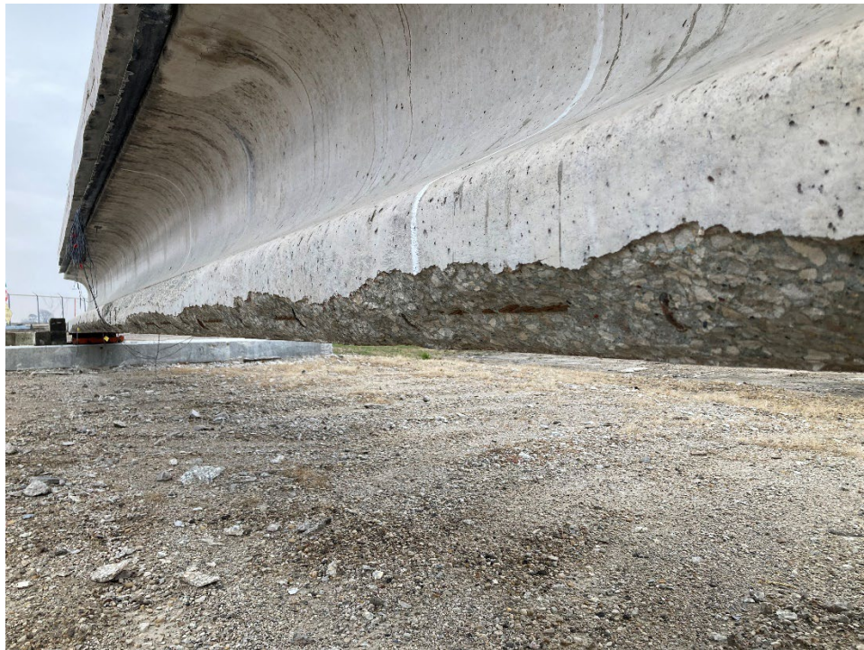
Figure 73. Removal of loose bottom flange concrete
