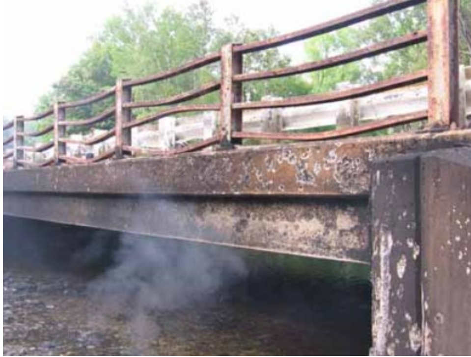
Figure 17. US 7 Bridge fascia after fire
