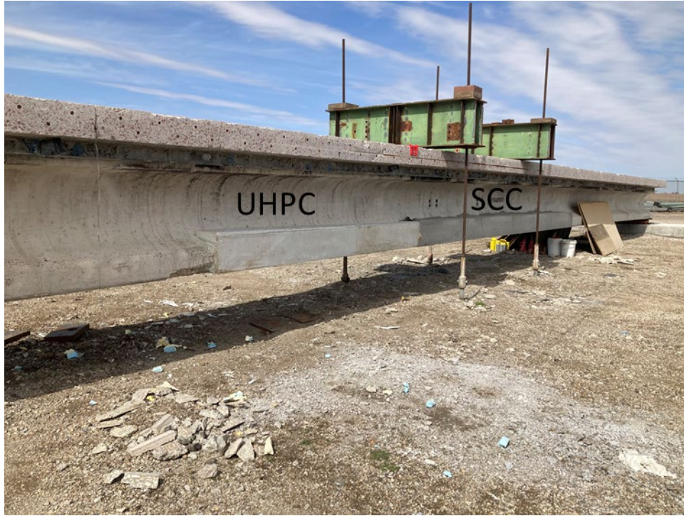
Figure 81. UHPC and SCC repair sections fully cast
