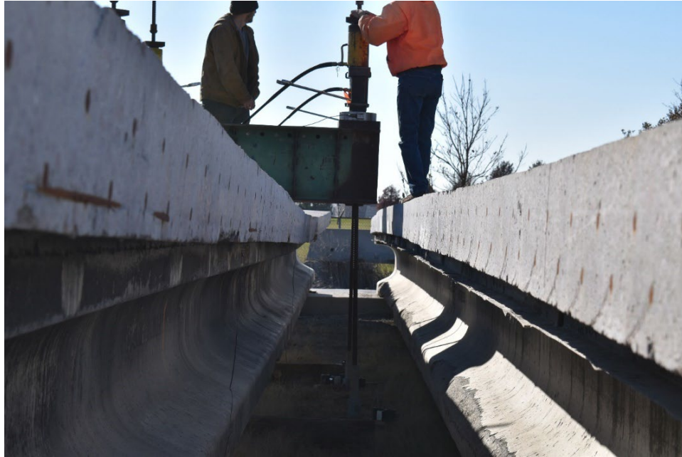
Figure 56. Deflected shape of Girder B at max loading
