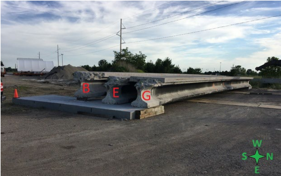
Figure 8. Girders B, E, and G at Iowa DOT maintenance yard
