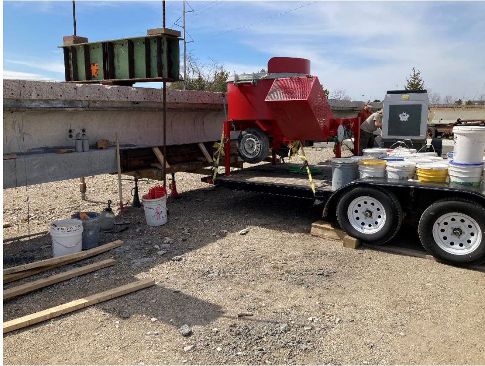
Figure 79. UHPC materials and mixer
