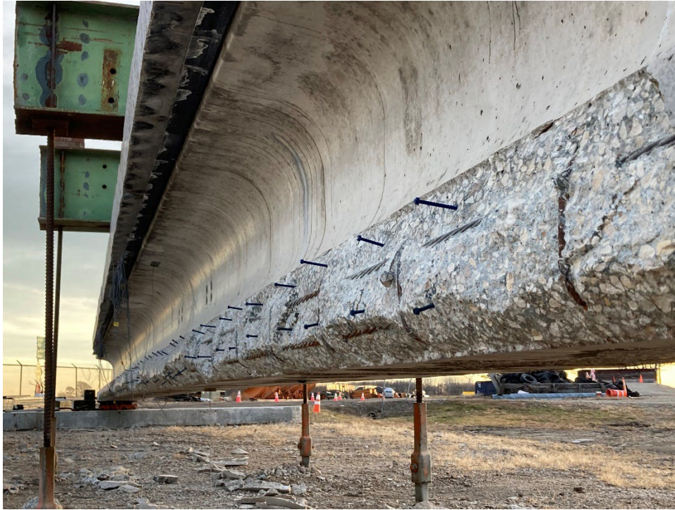
Figure 75. Concrete anchors into bottom flange
