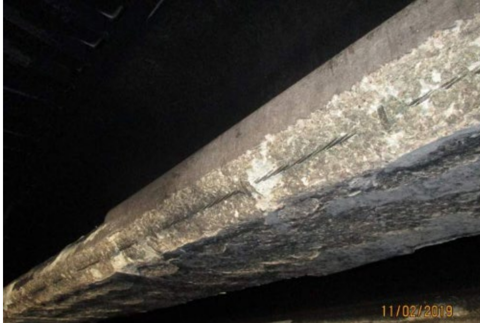
Figure 3. Exposed steel reinforcement strands and stirrups on Beam E
