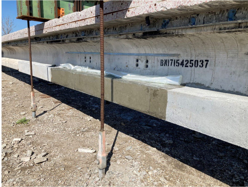
Figure 86. FRP wrap application on bottom flange repair
