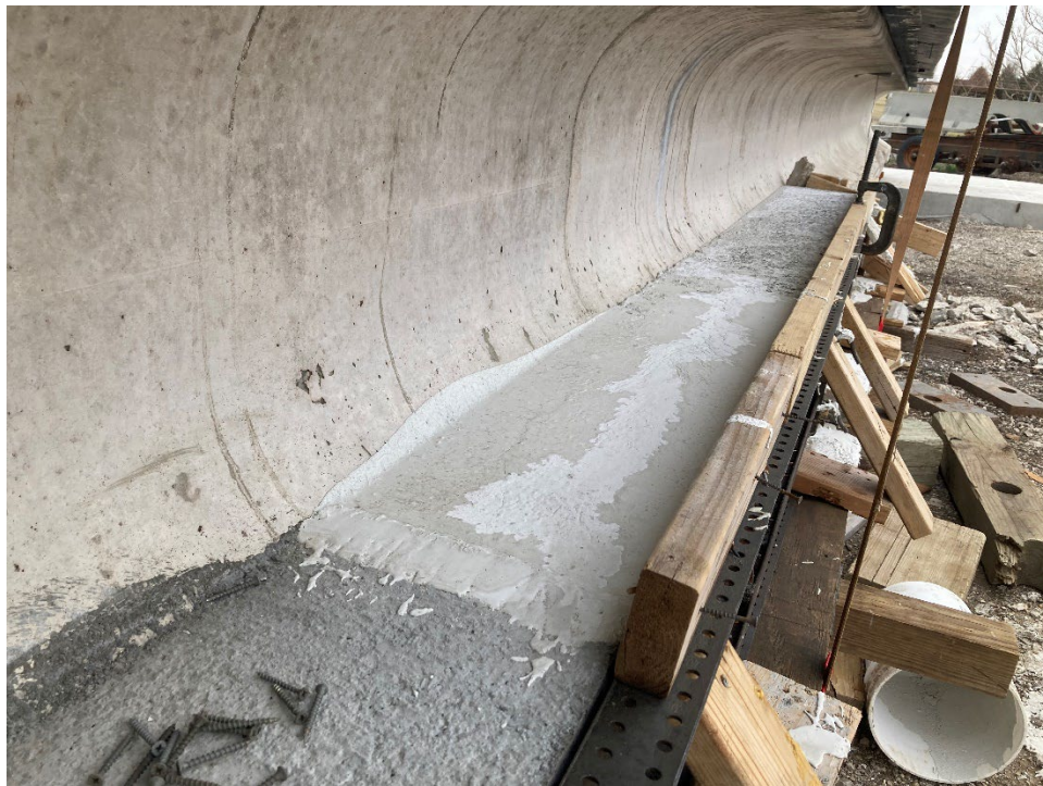
Figure 80. Placement of the UHPC section of repair
