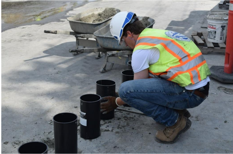
Figure 3-5. Making Concrete Test Specimens in the Field
