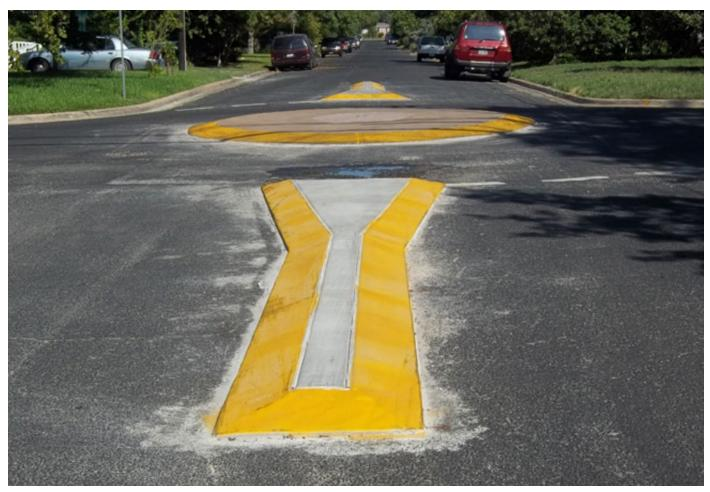
Images of several physical engineering countermeasures used are shown above: Rain Garden Bulb Out (top left), Median and Speed Cushions (top right), and Mountable Traffic Circles (bottom). Source: City of Austin
