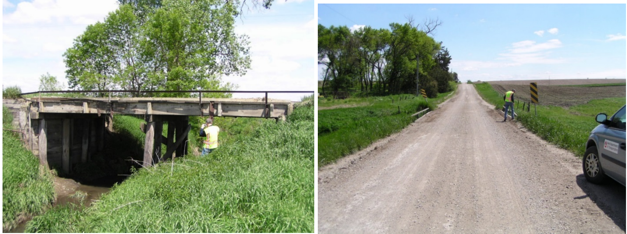
Figure C-2. Timber-Timber Bridge 1: West elevation view (left) and north end view (right)
