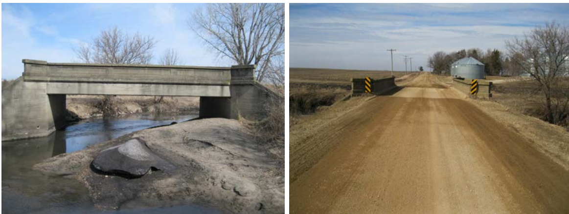
Figure A-26. Steel-Concrete Bridge 4: Elevation view (left) and end view (right)
