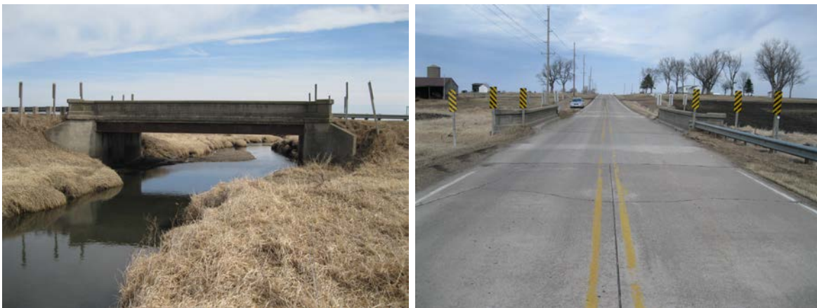
Figure A-33. Steel-Concrete Bridge 5: Elevation view (left) and end view (right)
