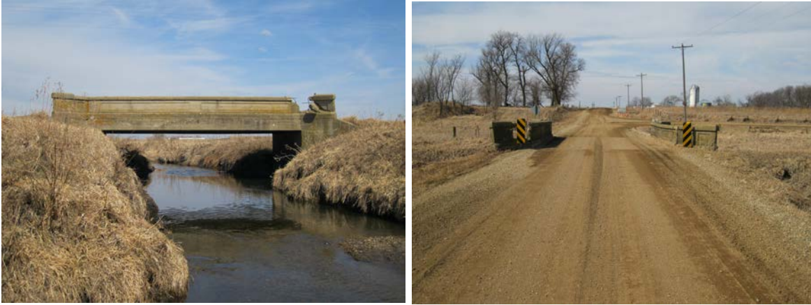
Figure A-2. Steel-Concrete Bridge 1: Elevation view (left) and end view (right)
