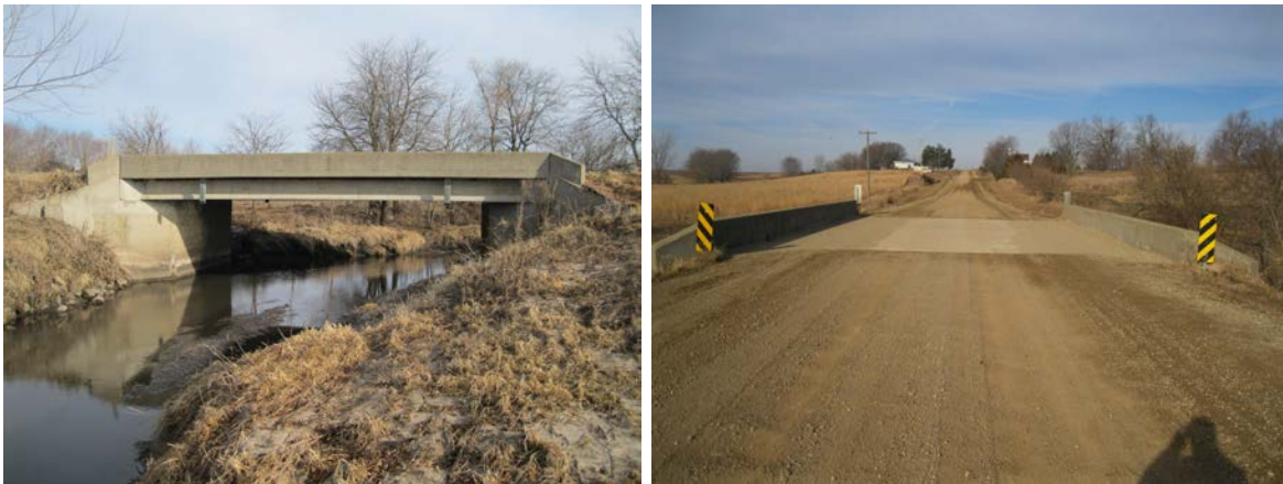
Figure A-10. Steel-Concrete Bridge 2: Elevation view (left) and end view (right)
