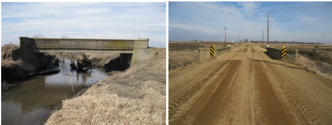
Figure A-18. Steel-Concrete Bridge 3: Elevation view (left) and end view (right)
