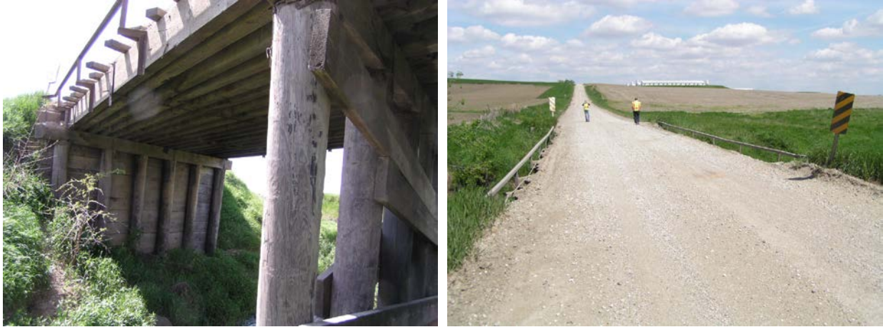
Figure C-18. Timber-Timber Bridge 3: Elevation view (left) and east end view (right)
