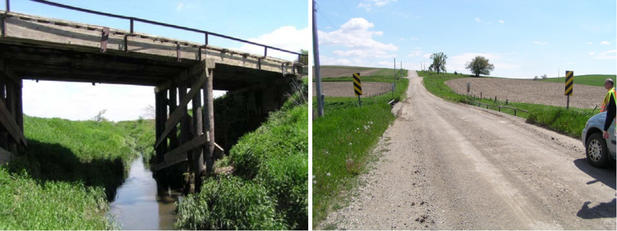
Figure C-10. Timber-Timber Bridge 2: West elevation view (left) and south end view (right)
