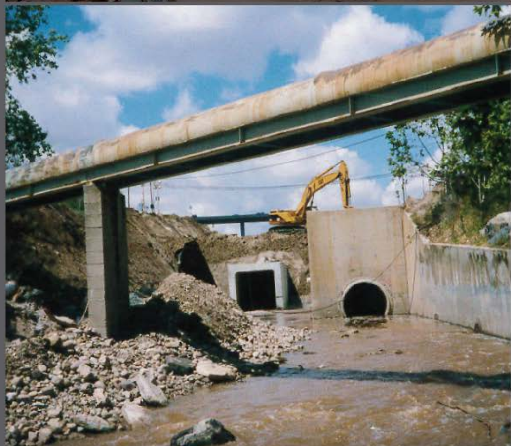
CULVERT | BALBOA AVENUE AND I-15 RECONSTRUCTION
