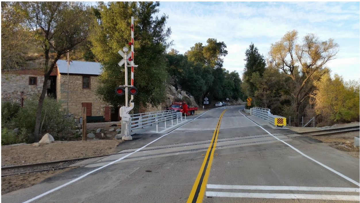
After Bridge Replacement
