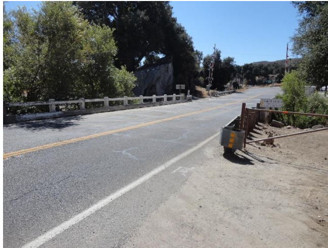
Before Bridge Replacement
