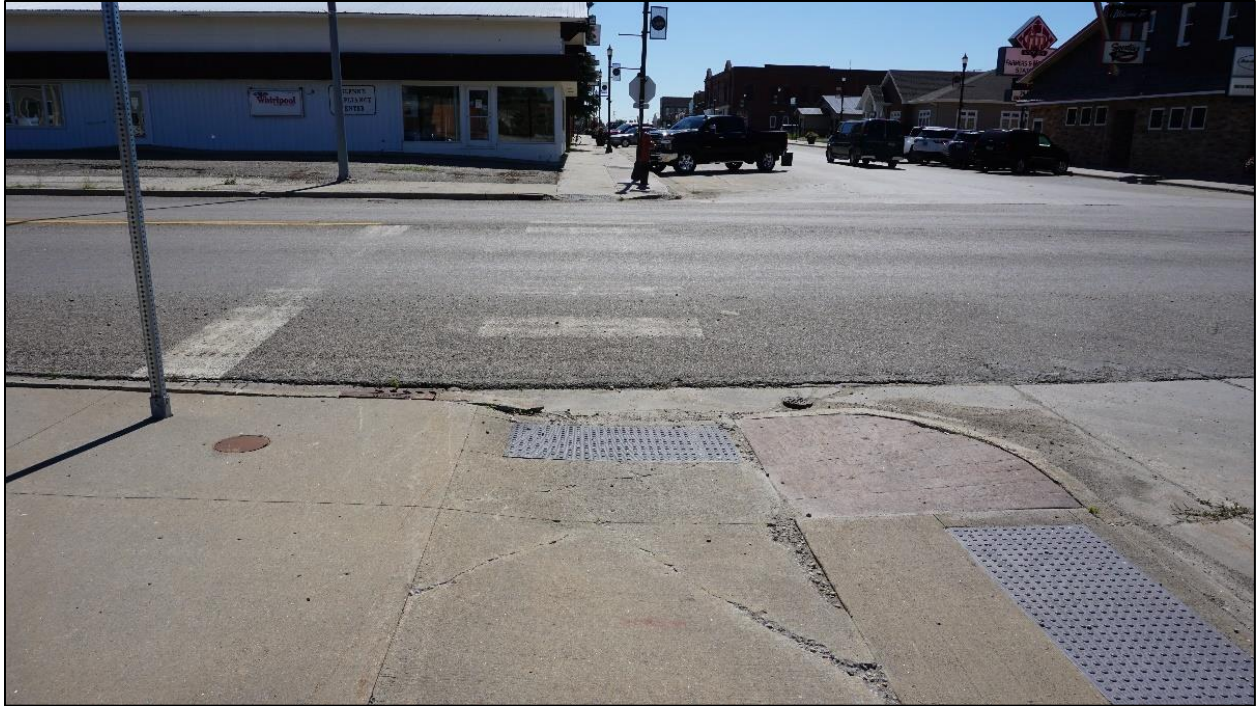
Figure 4. Ramps, sidewalk and crosswalk at Third Street across ND Highway 5
