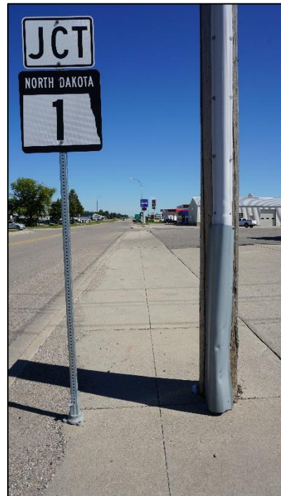
Figure 17. Route sign and utility pole obstructing sidewalk
