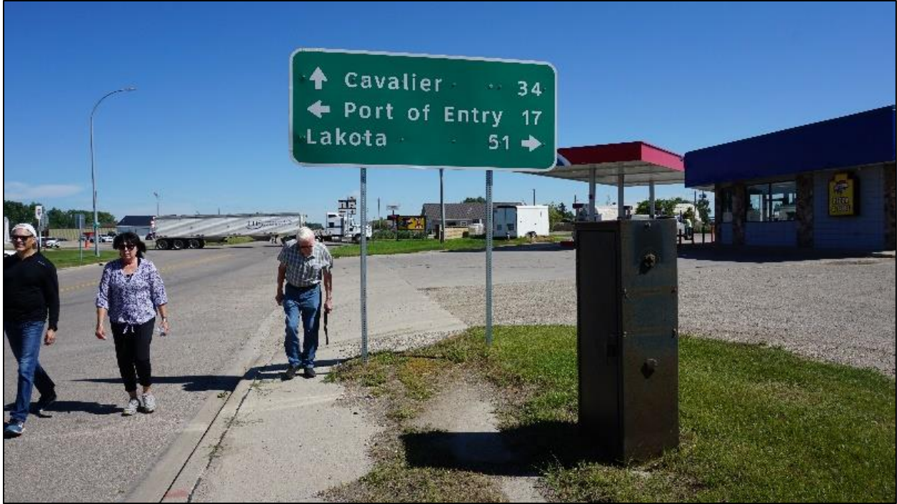
Figure 16. Guide sign obstructing the sidewalk
