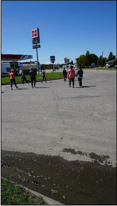
Figure 14. Lack of crosswalk/sidewalk on the south side of ND Highway 5 at ND Highway 1
