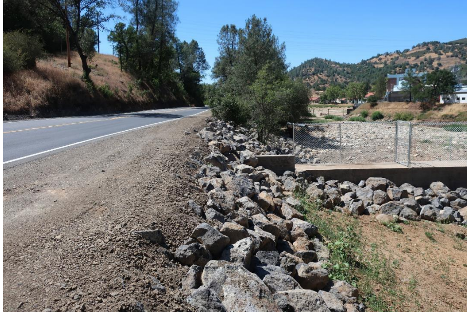
FIGURE 27: REPAIRED ROADWAY SR 49 IN TUOLUMNE COUNTY, MAY 2018
