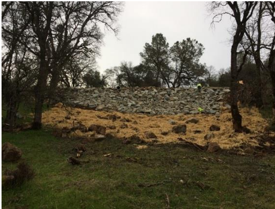
FIGURE 3: EXAMPLE OF LANDSLIDE REPAIR WORK ON SR 26
