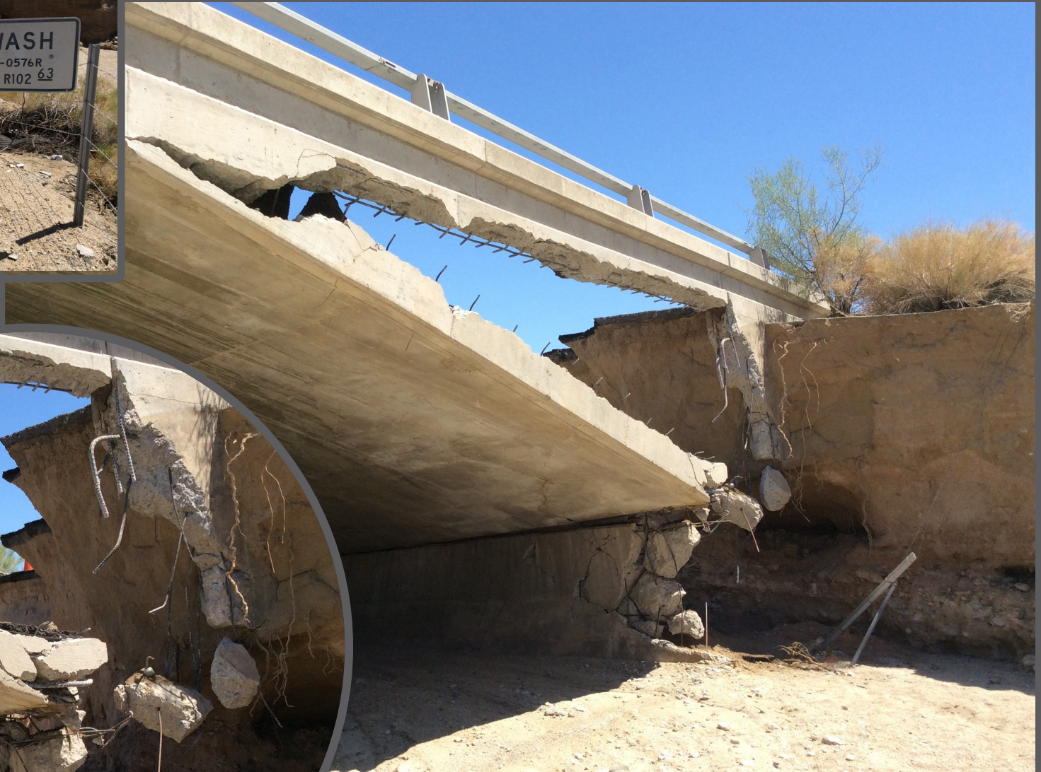
HEAVY WATER FLOW THROUGH TEX WASH CAUSED EAST BOUND COLLAPSE AND ABUTMENT, WING WALL, AND FOOTING DAMAGE
