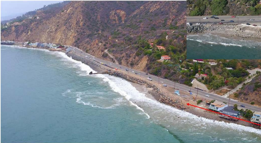
6/15/2016 Aerial of completed project looking north.
