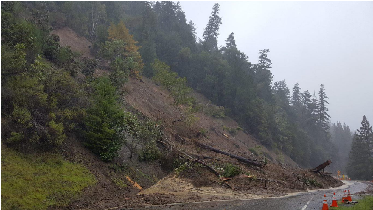
FIGURE 10-2: SR 1 NEAR LEGGETT MUDSLIDE
