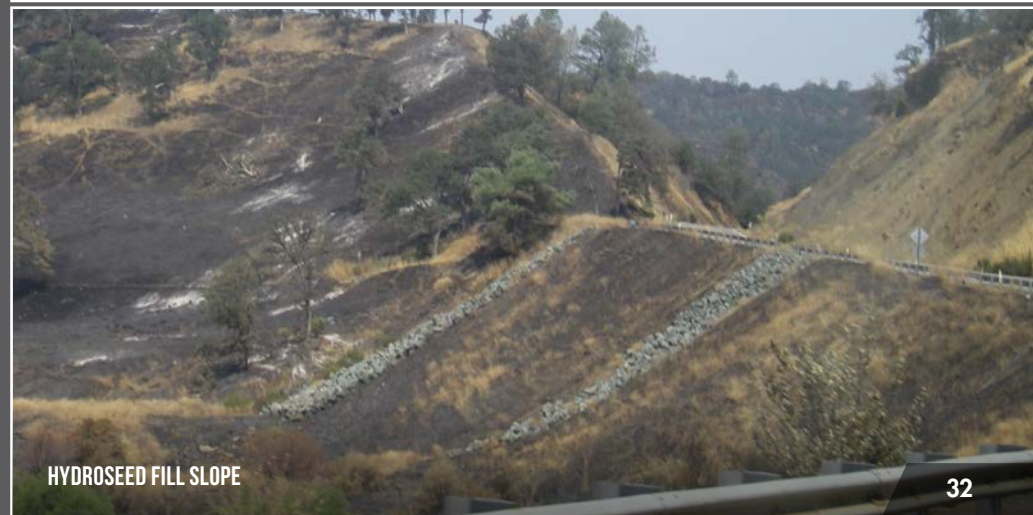
ARMOR RILL IN CUT SLOPE WITH RSP
