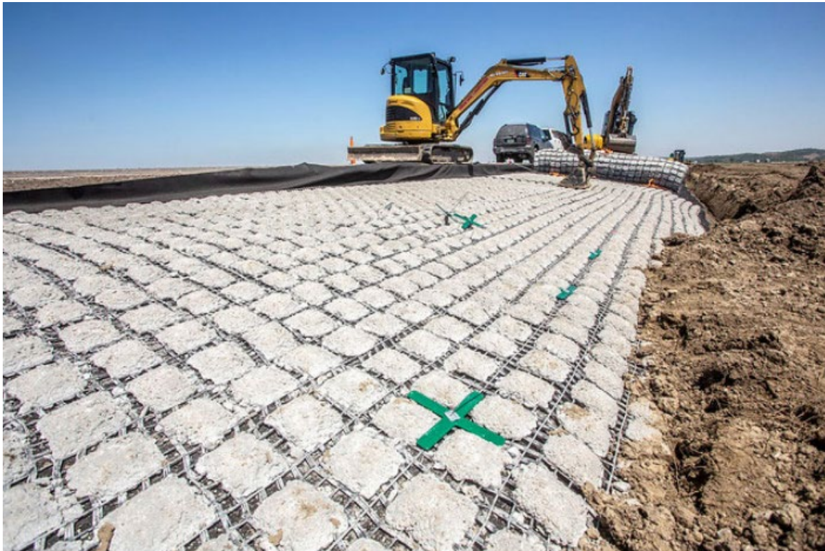
Figure 3 Example of tied concrete block mats in use in western Iowa to protect roadway shoulders from erosion caused by flooding. Source: Iowa Department of Transportation.
