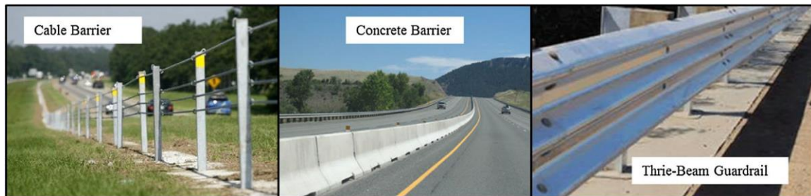
Figure 1. Photos. Standard roadside barriers deployed in Georgia in addition to the W-beam system.
