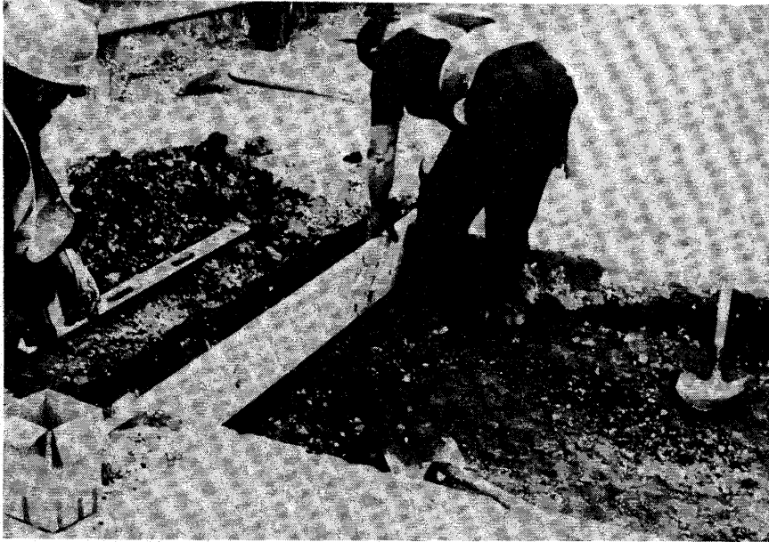
FIGURE 13 – PLACE FORM A removable wood form is being installed.
