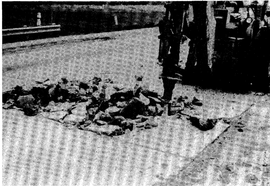
FIGURE 7 – BREAK CONCRETE Breaking concrete with pavement breaker.
