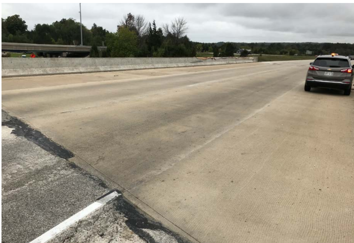
Figure C-4. I-43 bridge deck over Beloit Rd. (Site #4, I-43, New Berlin).
