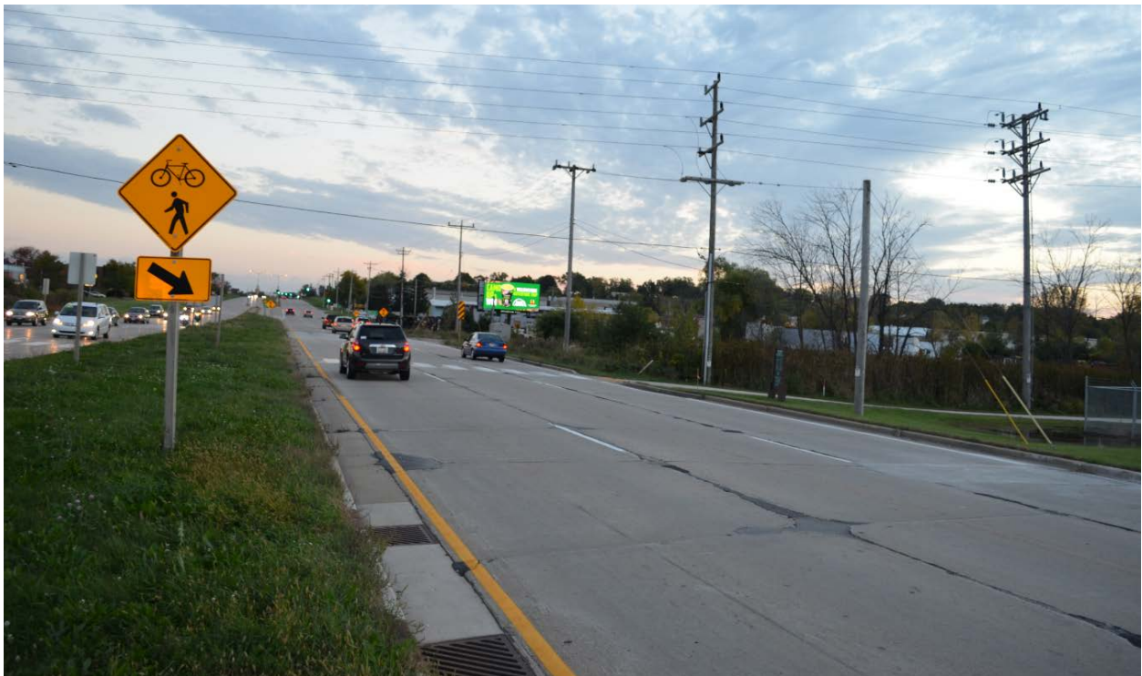
Figure F-5. Overview of existing concrete pavement (Site #21, State Road 59, Waukesha).
