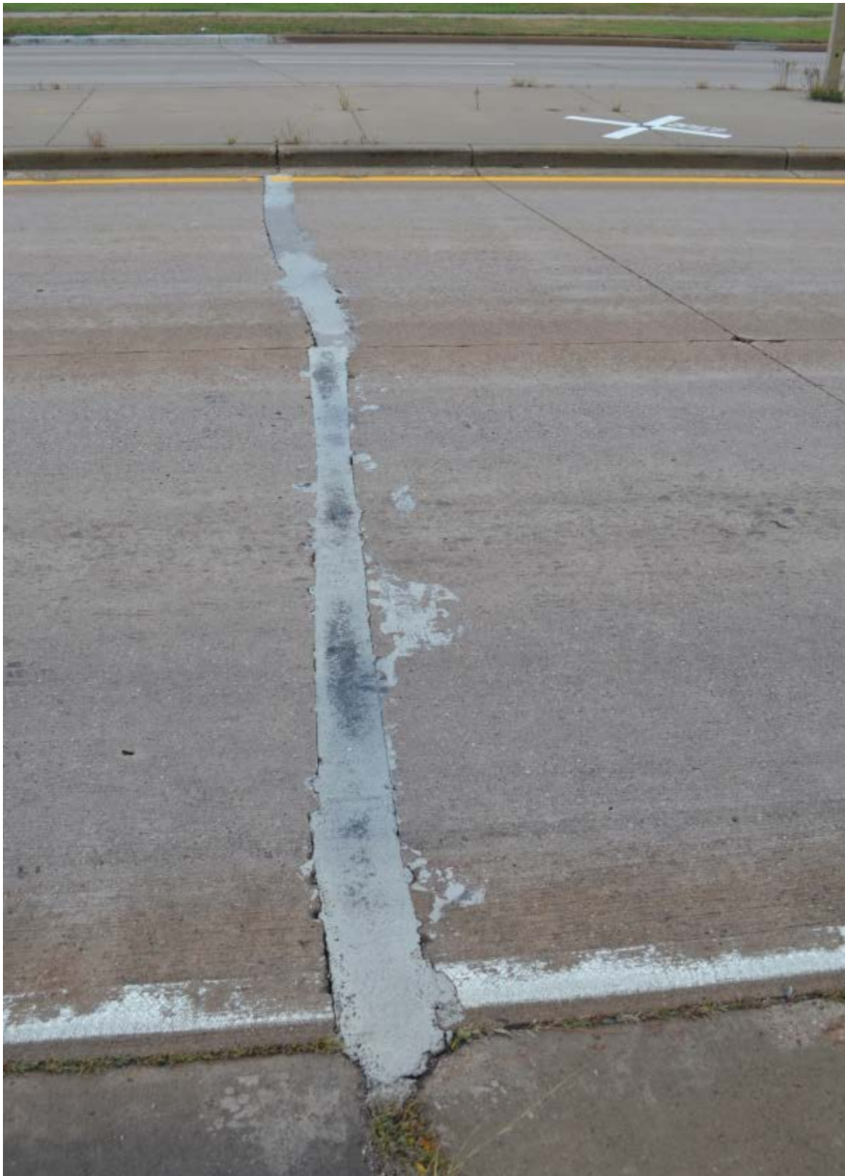
Figure E-9. PDR used to address transverse cracking (Site #11, US 10, Stevens Point).
