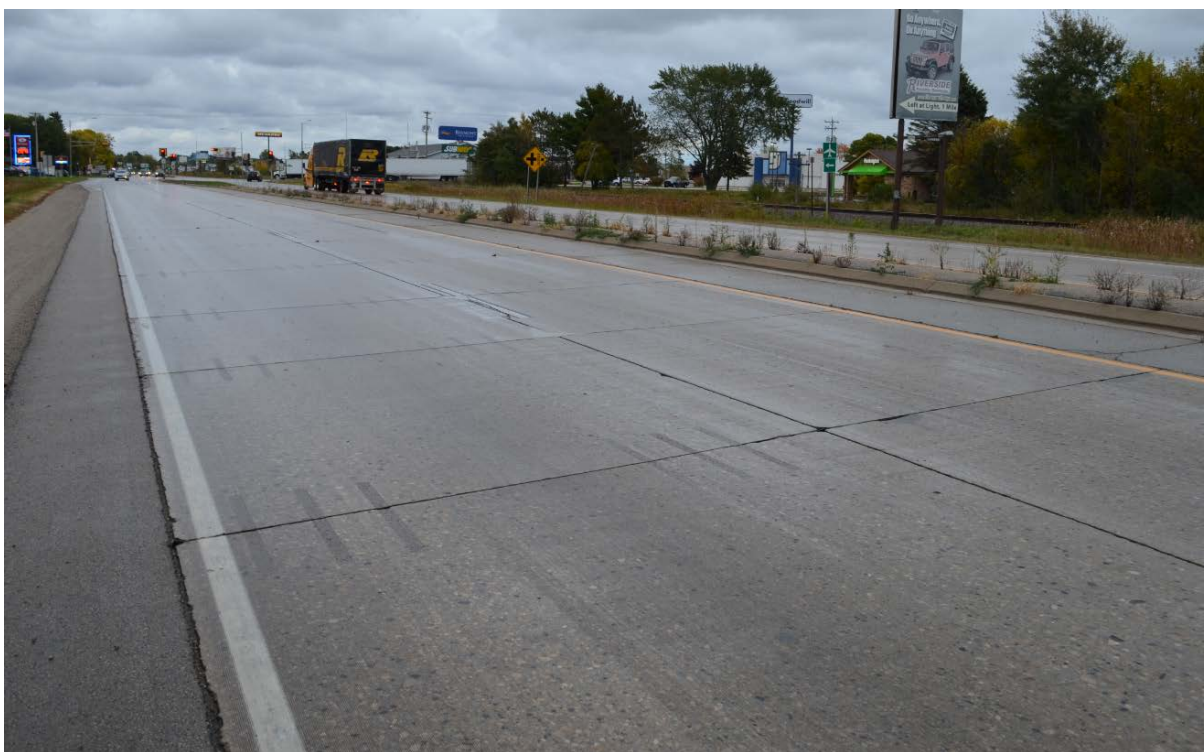
Figure E-14. Overview of existing concrete pavement (Site #12, US 41, Marinette).
