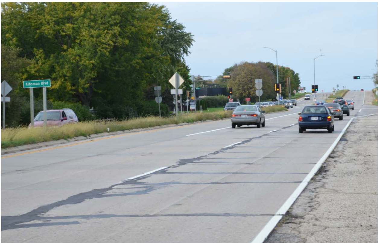
Figure F-3. Overview of existing concrete pavement (Site #20, N. Stoughton Rd., Madison).
