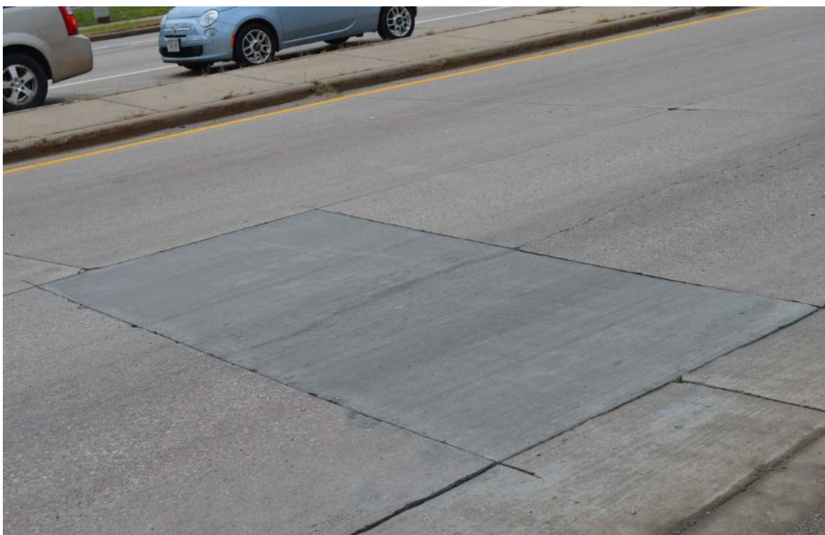
Figure E-11. Full depth repairs in existing concrete pavement (Site #11, US 10, Stevens Point).
