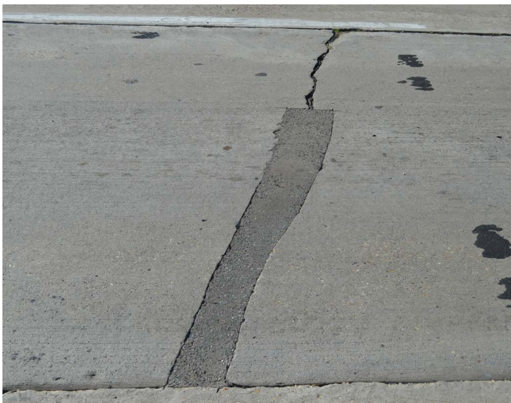
Figure E-3. PDR over a transverse crack (Site #9, State Road 66, Stevens Point).
