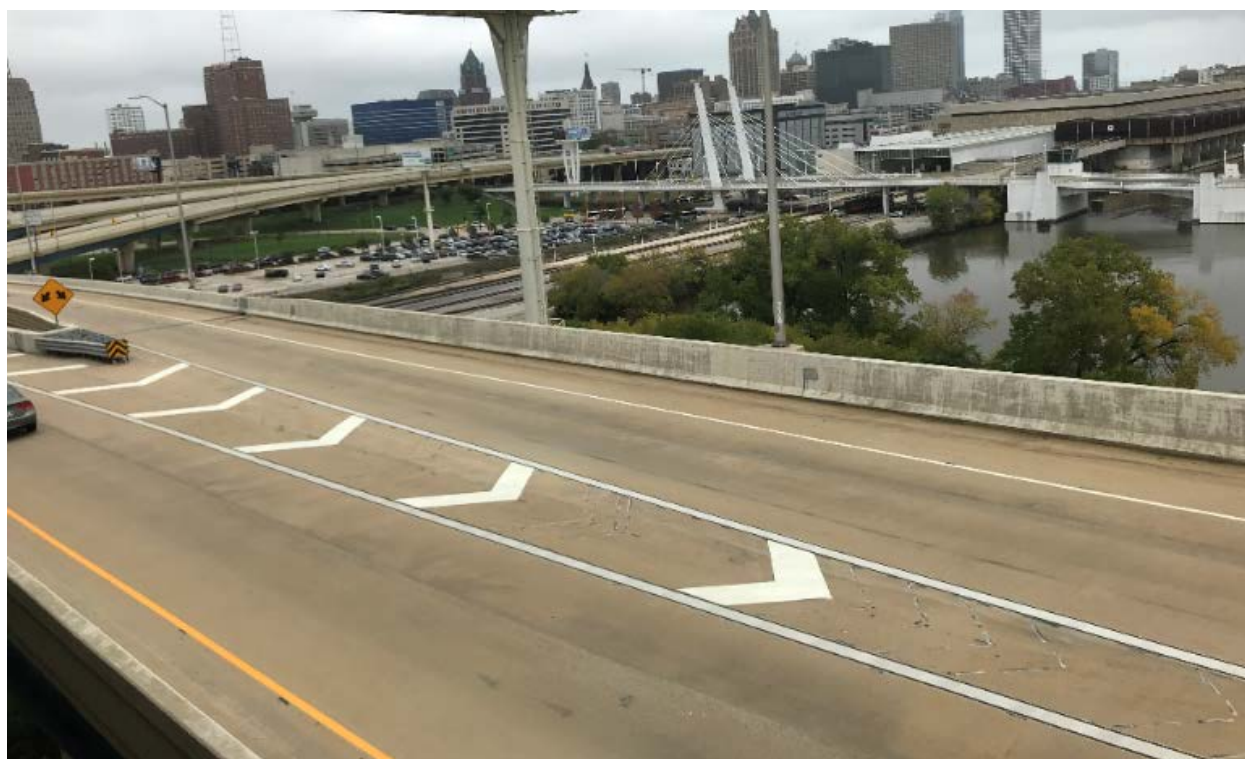
Figure C-2. Marquette Interchange bridge deck overview (2) (Site #2, I-43, Milwaukee).
