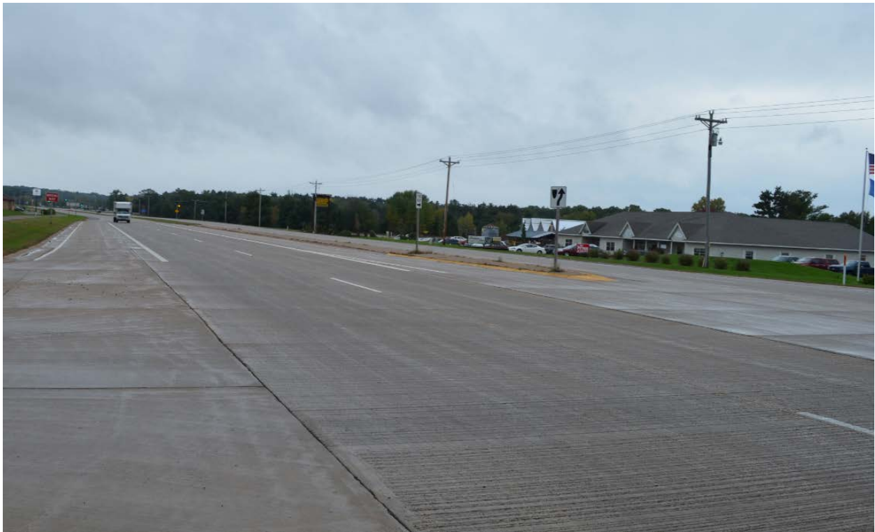
Figure F-2. Overview of generally distress-free surrounding concrete pavement (Site #19, State Road 93, Eau Claire).
