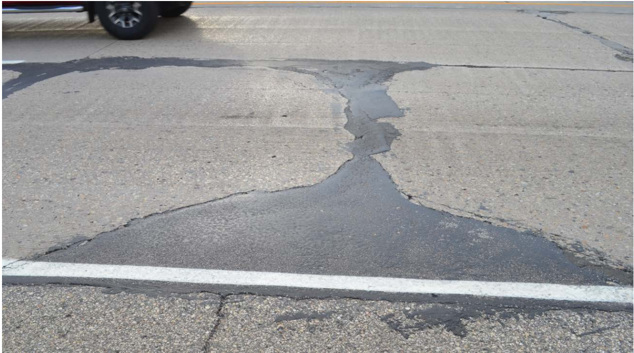
Figure F-4. PDR used to address a severely distressed area (Site #20, N. Stoughton Rd., Madison).
