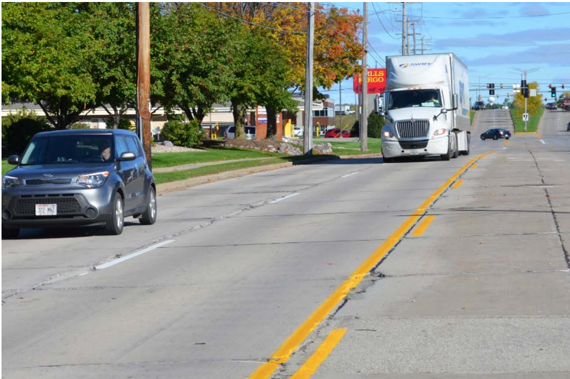
Figure F-8. Overview of existing concrete pavement (Site #22, N. Ballard Rd., Appleton).
