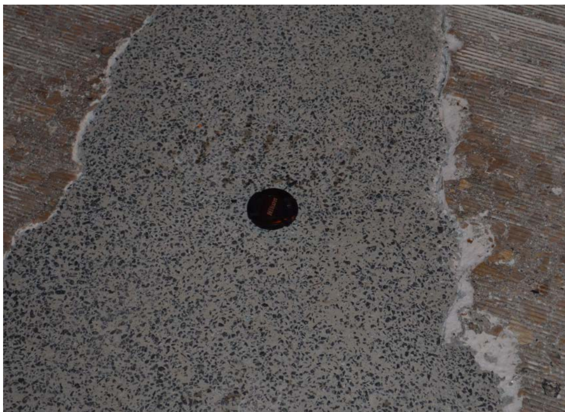
Figure B-8. RM-1 PDR (7)—close-up of repair surface (Site #1, US 12/18, Madison Beltline).
