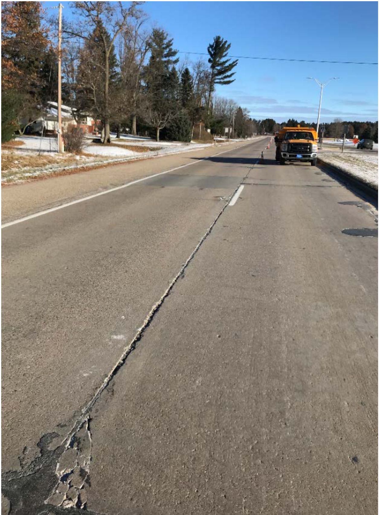
Figure D-7. Overview of existing concrete pavement (Site #8, State Road 66, Stevens Point).
