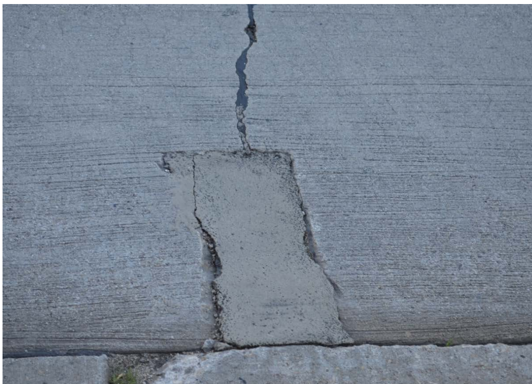
Figure E-4. Material loss along edges of a small PDR (Site #9, State Road 66, Stevens Point).
