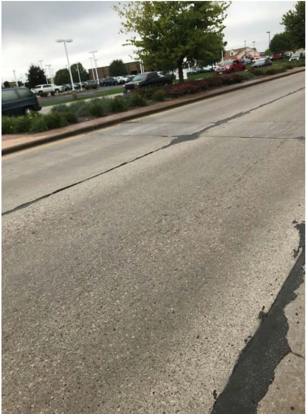
Figure D-4. Overview of existing concrete pavement (Site #6, Plover Rd., Plover).
