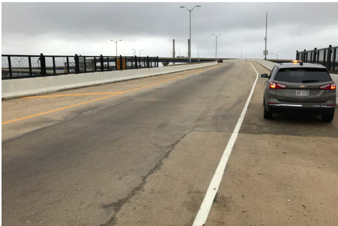
Figure C-1. Marquette Interchange bridge deck overview (Site #2, I-43, Milwaukee).
