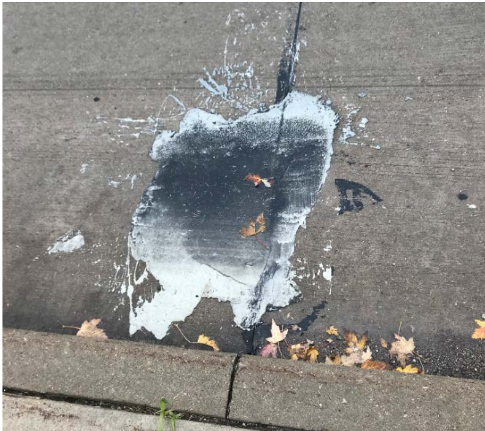
Figure E-22. PDR to address joint spalling (Site #15, Calumet St., Appleton).
