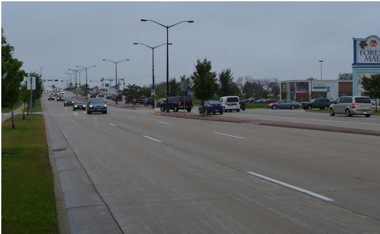
Figure E-26. Overview of existing concrete pavement in very good condition (Site #17, W. Johnson St., Fond du Lac).
