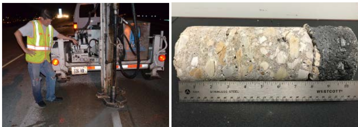
Figure 3-5. Coring operation in progress for core #2 (left) and the extracted core #2 (right).
