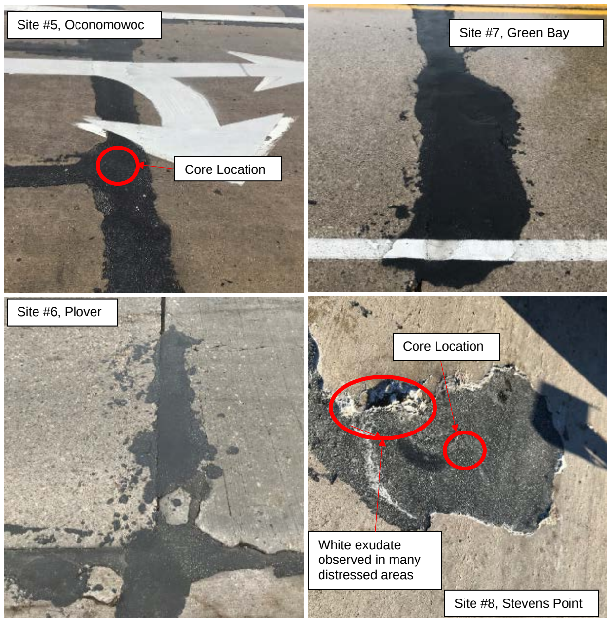
Figure 3-13. RM-3 used in concrete pavement PDR applications.
