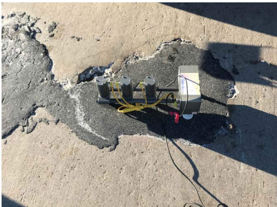
Figure D-10. PSPA testing in progress on PDR in slab interior (Site #8, State Road 66, Stevens Point).
