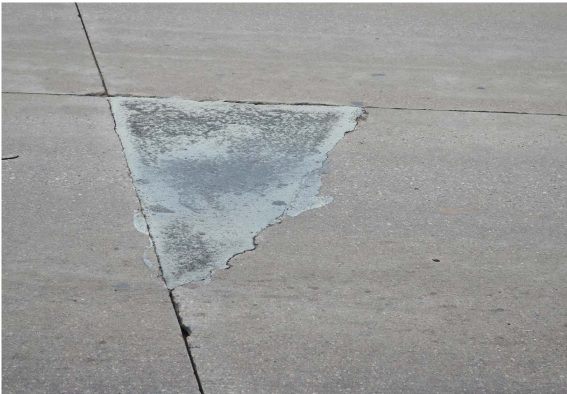
Figure E-13. PDR to address corner break (Site #11, US 10, Stevens Point).
