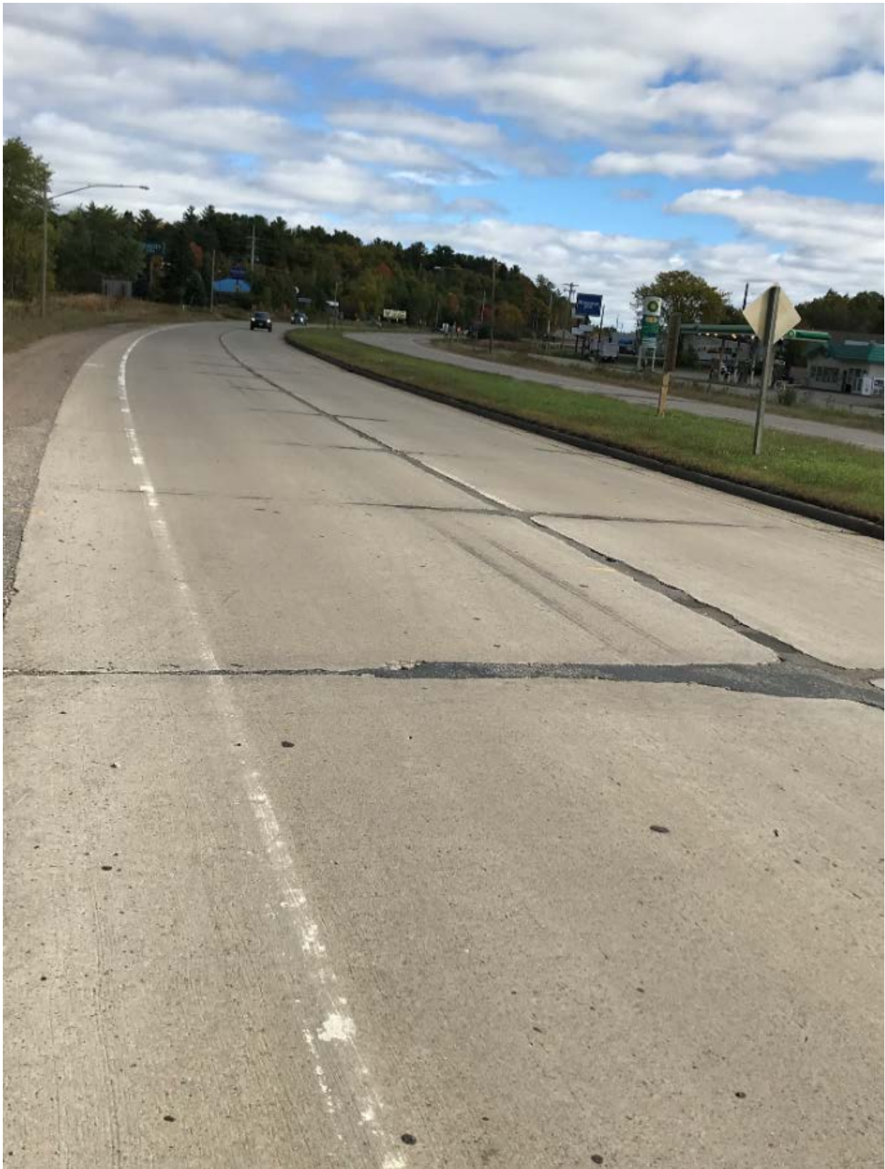
Figure F-11. Overview of existing concrete pavement (Site #23, W. Kemp St., Rhineland).
