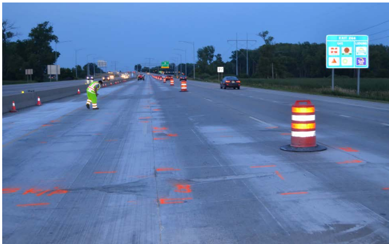
Figure B-11. Workzone—areas being marked for full-depth repairs (Site #1, US 12/18, Madison Beltline).
