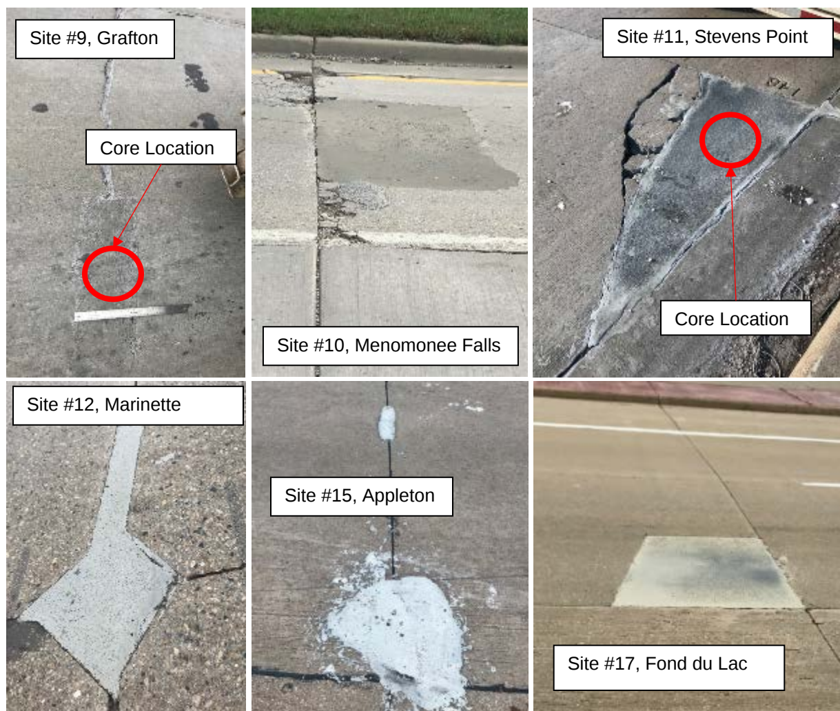
Figure 3-16. RM-4 used in concrete pavement PDR applications.
