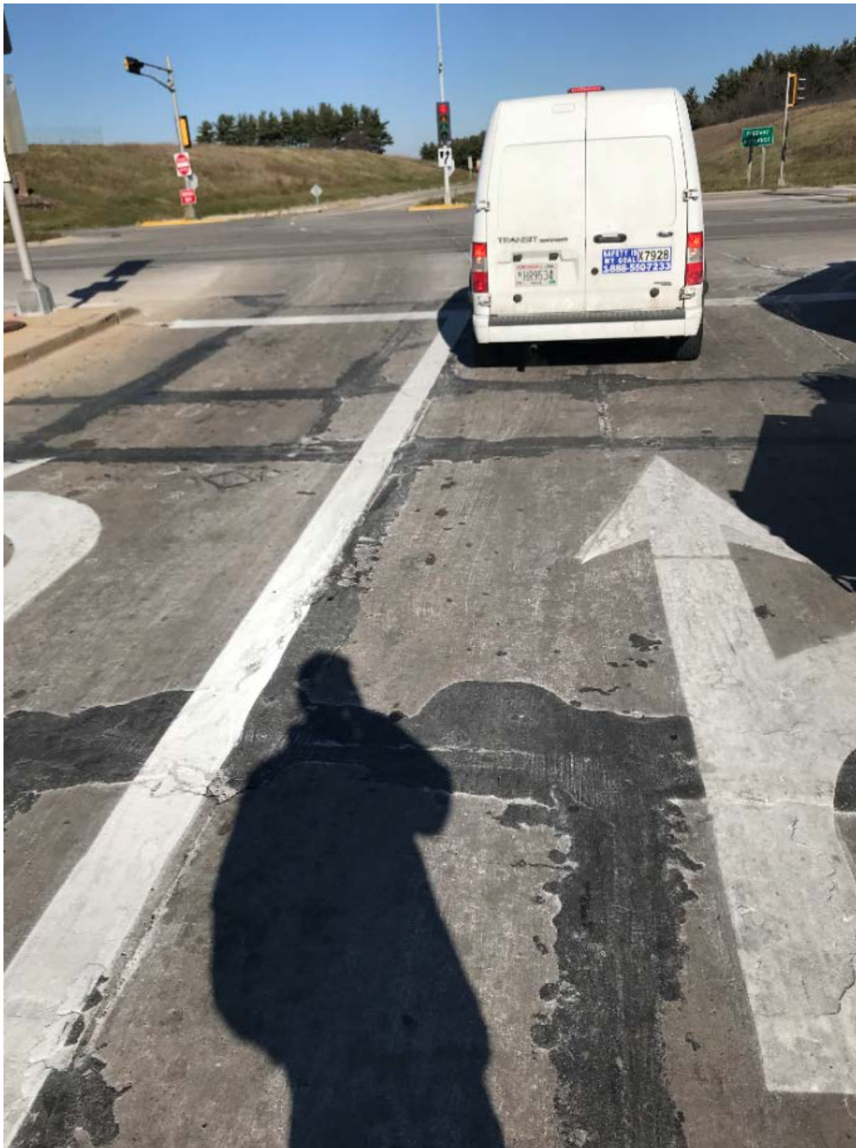
Figure D-1. RM-3 used to repair spalls, deteriorated joints and traffic loops (Site #5, W. Wisconsin Ave, Oconomowoc).
