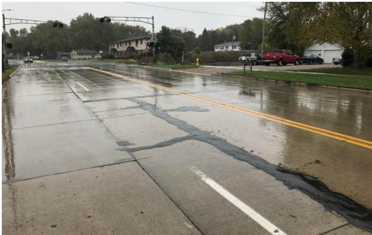
Figure D-5. Overview of RM-3 repairs (Site #7, S. Taylor St., Green Bay).
