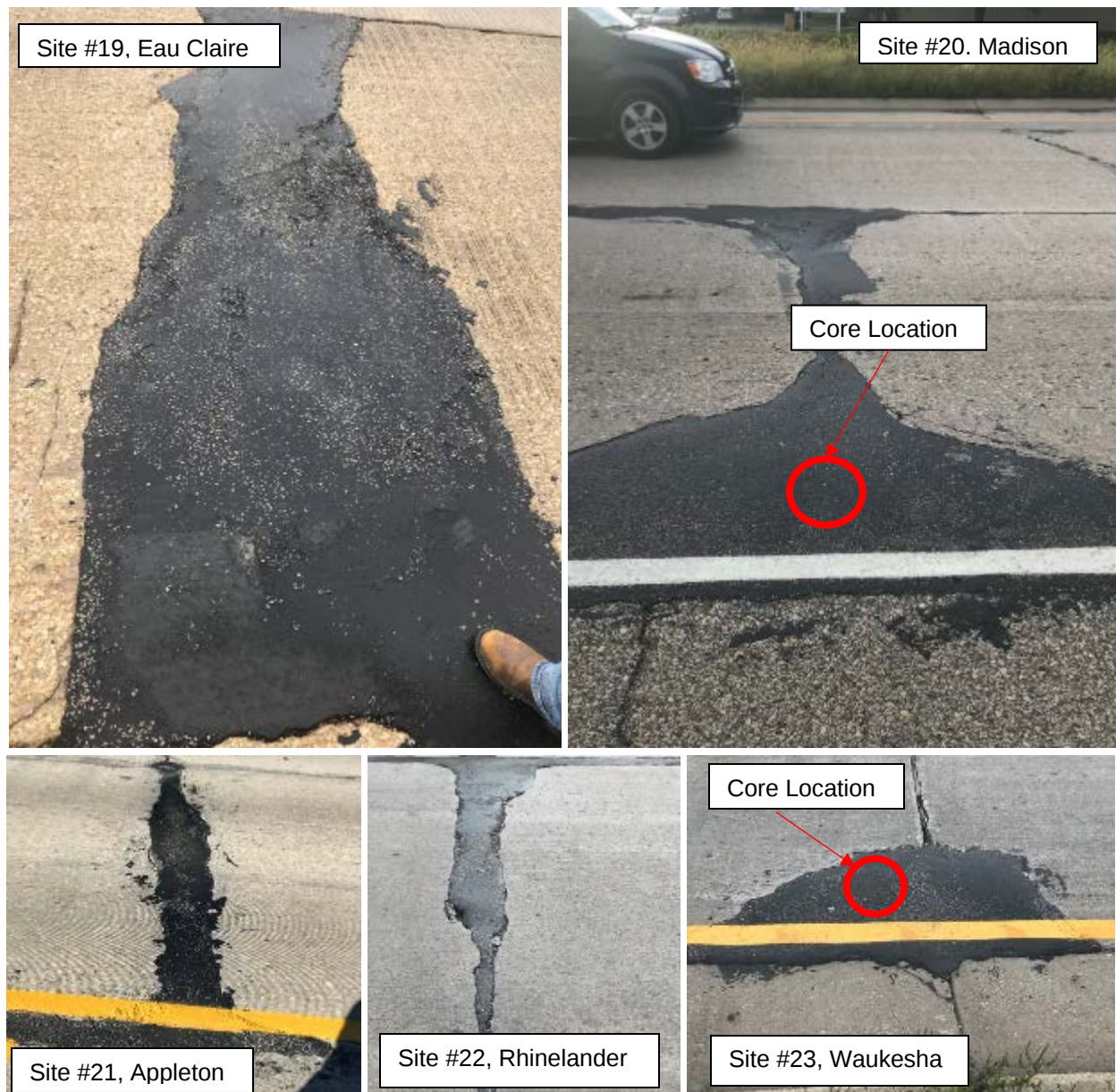
Figure 3-22. RM-5 used in concrete pavement PDR applications.
