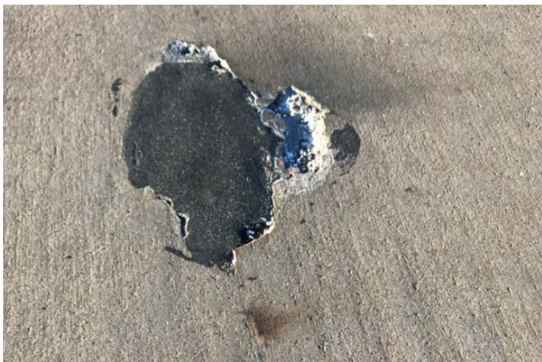
Figure D-9. Small spot repairs in slab interior (Site #8, State Road 66, Stevens Point).
