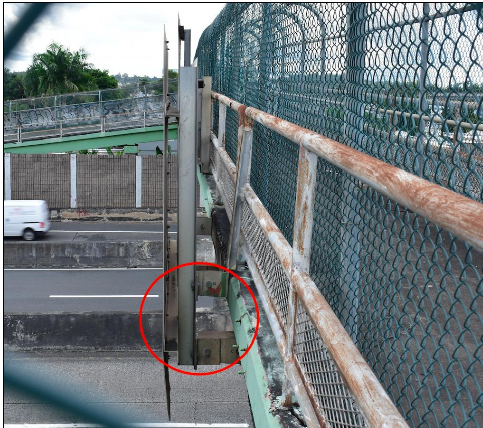
Figure 5.16: Traffic Signs partially detached from support
