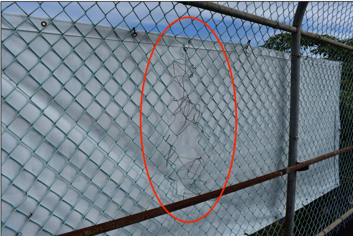
Figure 6.11: Hole in safety fence on PB 1095
