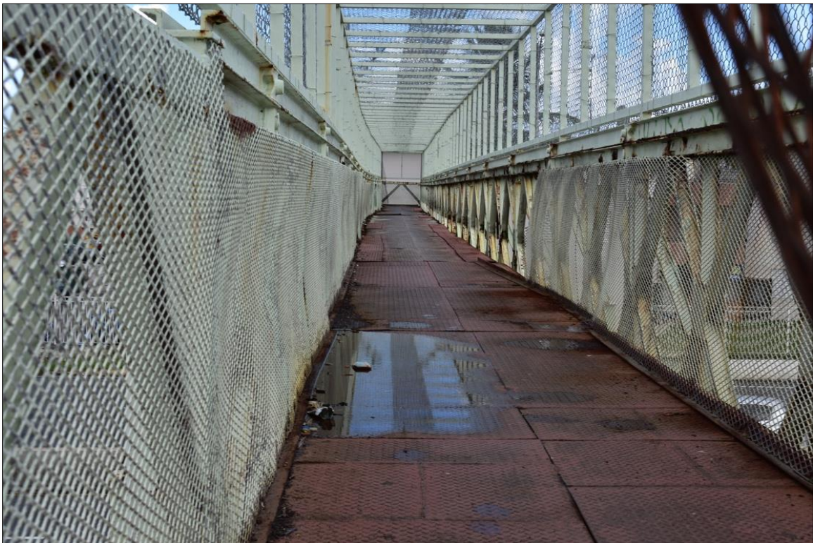
Figure 5.62: Corrosion on deck and section of guardrail without security meshing
