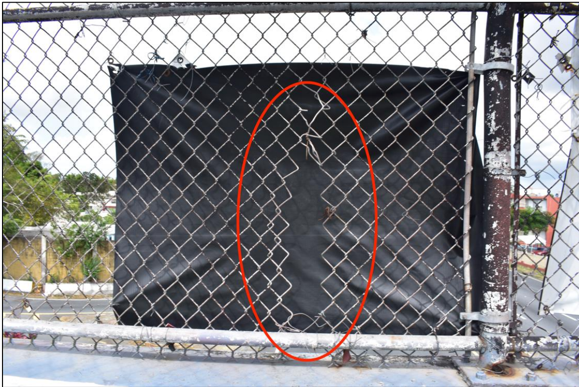
Figure 6.34: Security Fence with holes, Pedestrian Bridge 2355
