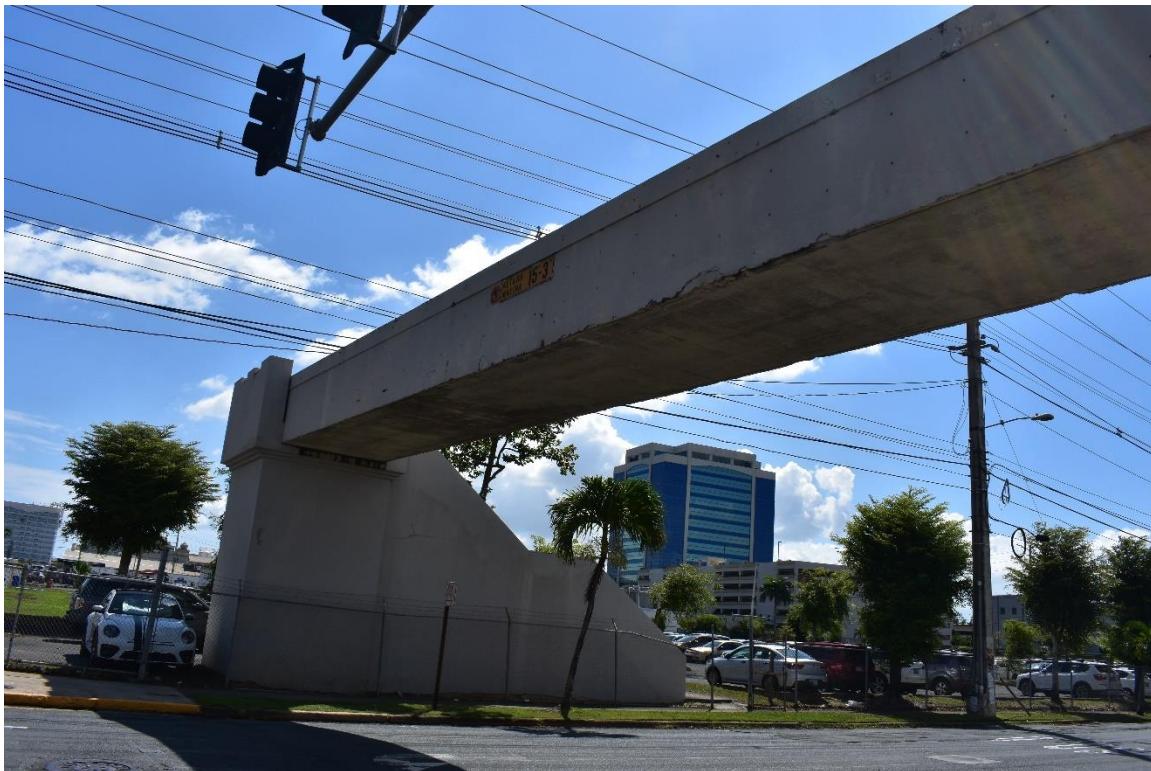
Figure 6.28: Electrical cables passing closely over PB 1926
