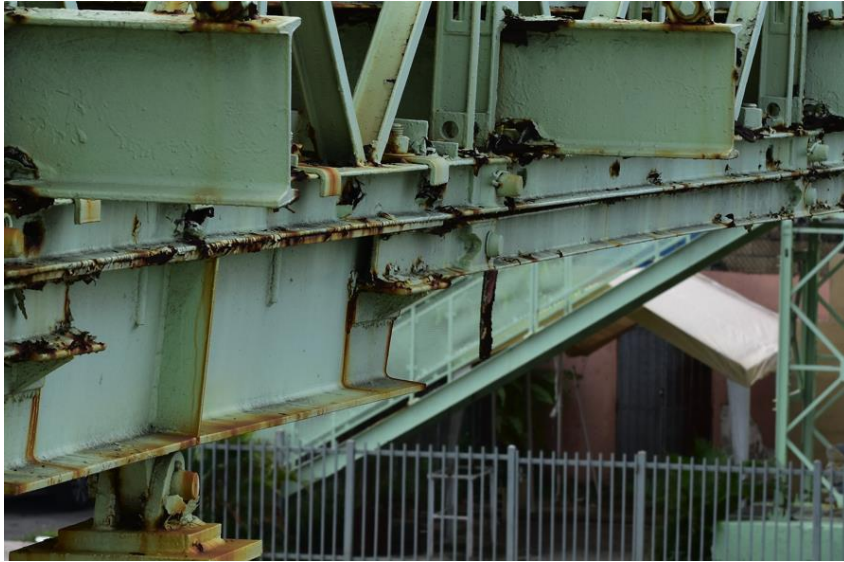
Figure 5.14: Corrosion in Floor Beams (Example 2)
