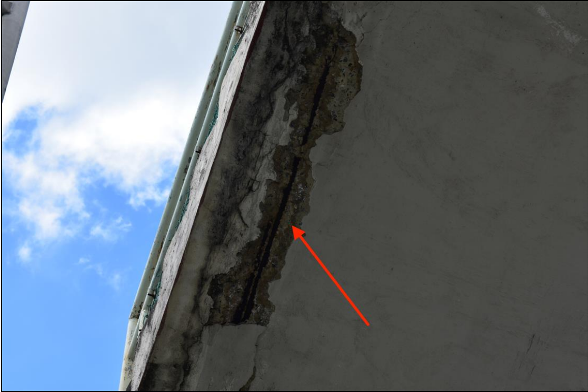
Figure 6.30: Exposed rebar on PB 2087
