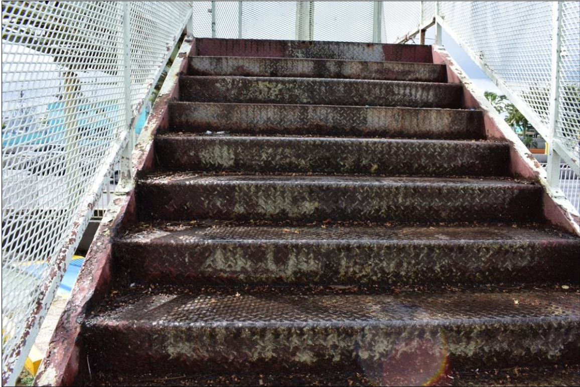
Figure 5.61: Corrosion on stairway
