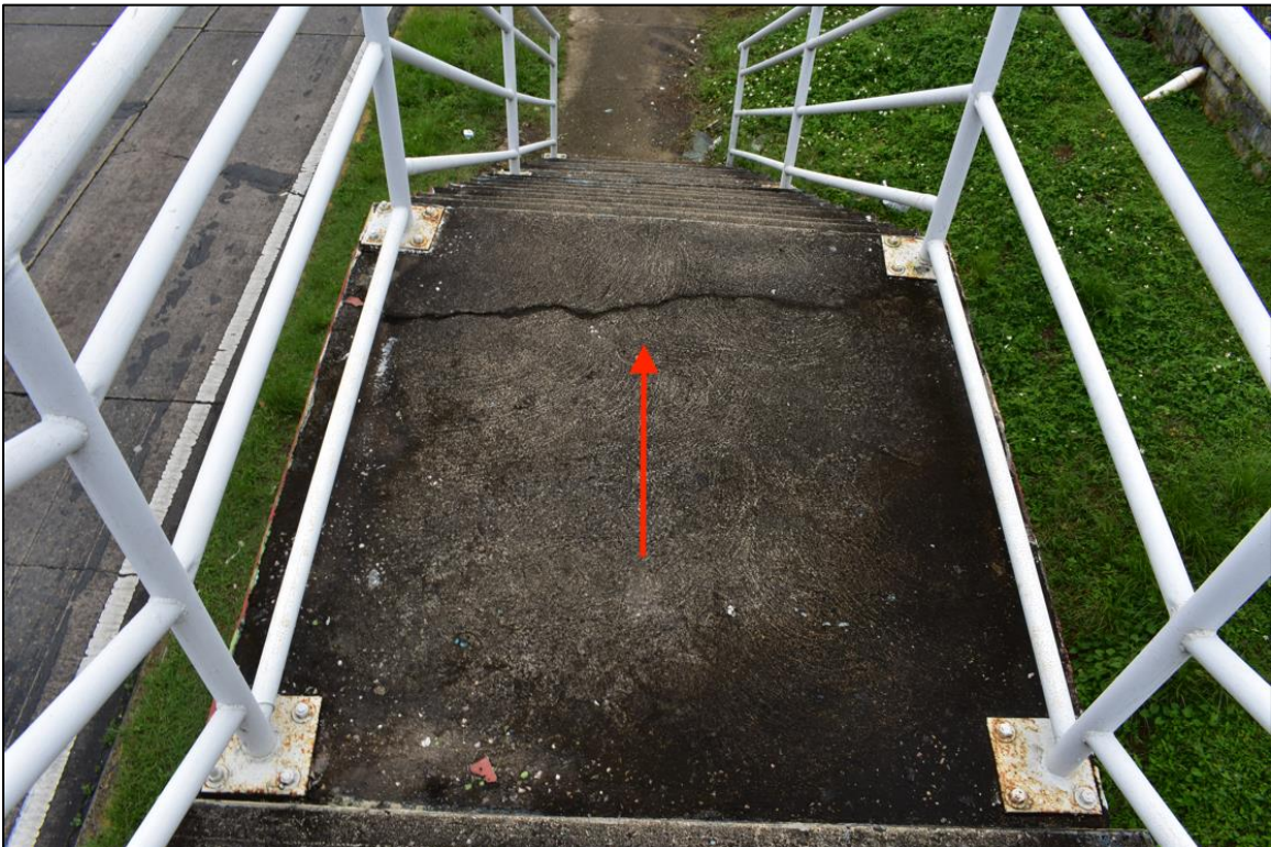
Figure 6.24: Crack on stairway of PB 1736
