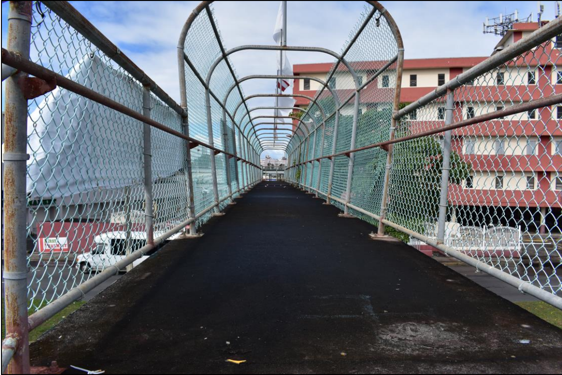
Figure 6.10: Mold and silt on PB 1095
