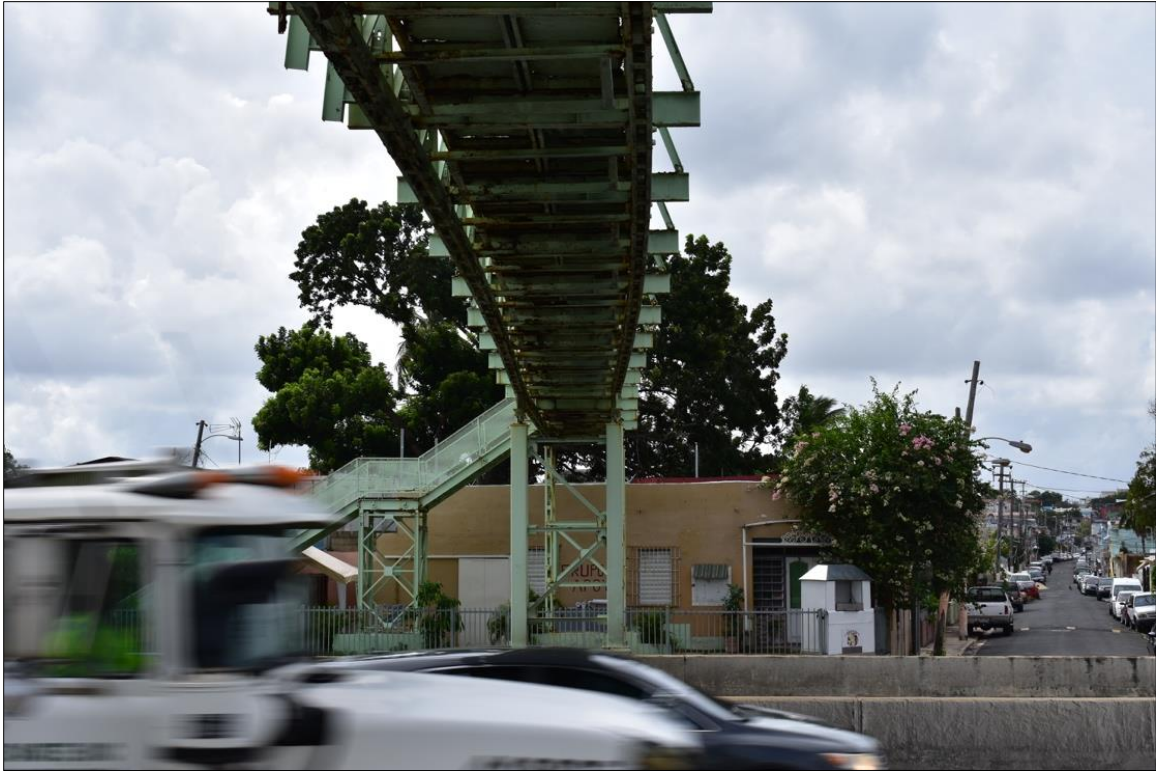
Figure 5.42: Underside view of lateral deflection
