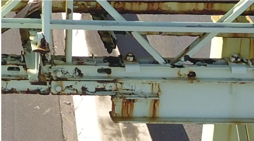
Figure 5.11: Corrosion in Truss Element (Example 2)
