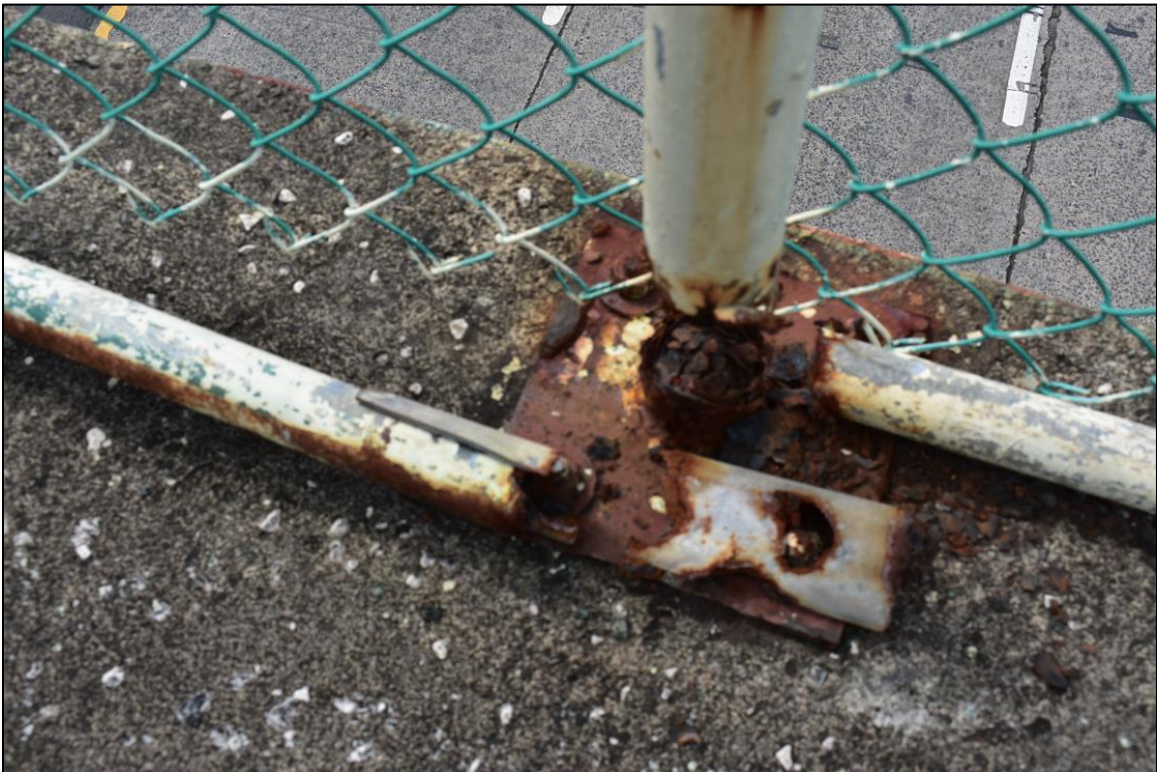
Figure 6.33: Corrosion of security fencing on PB 2087
