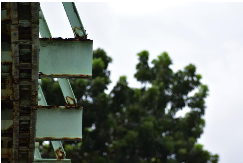
Figure 5.13: Corrosion in Floor Beams (Example 1)
