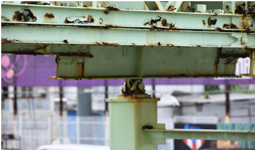
Figure 5.12: Corrosion in Truss Element (Example 3)
