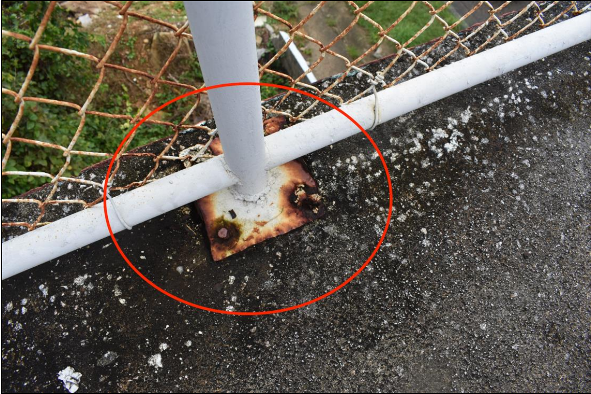
Figure 6.23: Corrosion of security fencing on PB 1736
