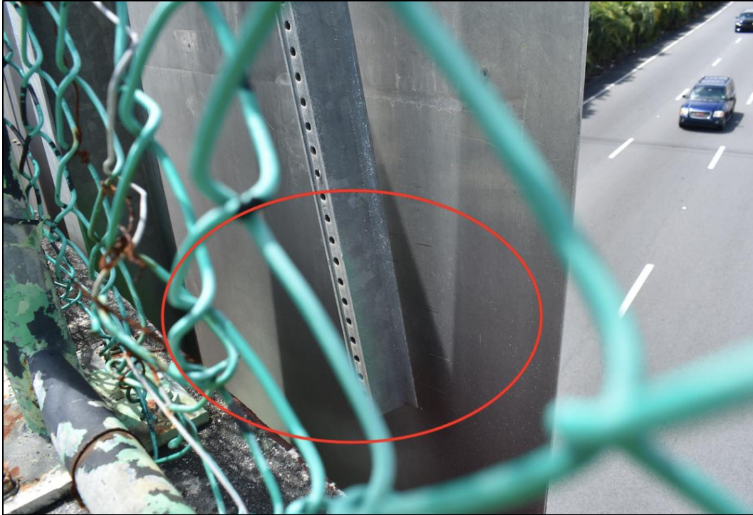
Figure 5.74: Transit sign detached from mounting assembly
