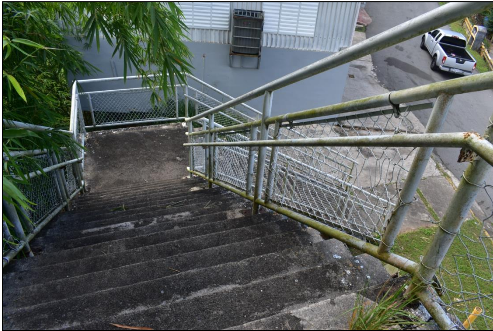
Figure 6.20: Mold and silt on PB 1513
