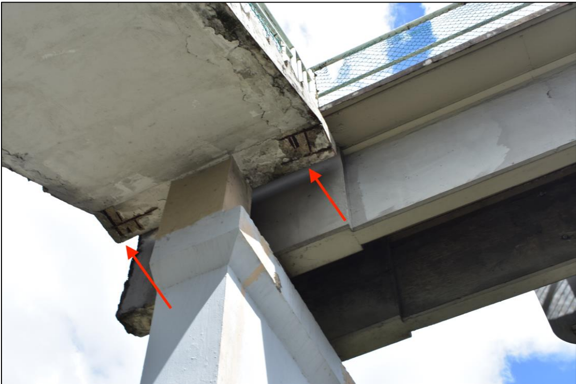
Figure 6.31: Exposed rebars on PB 2087
