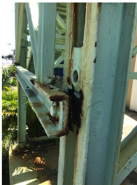
Figure 5.15: Loose Connection at Column Tower
