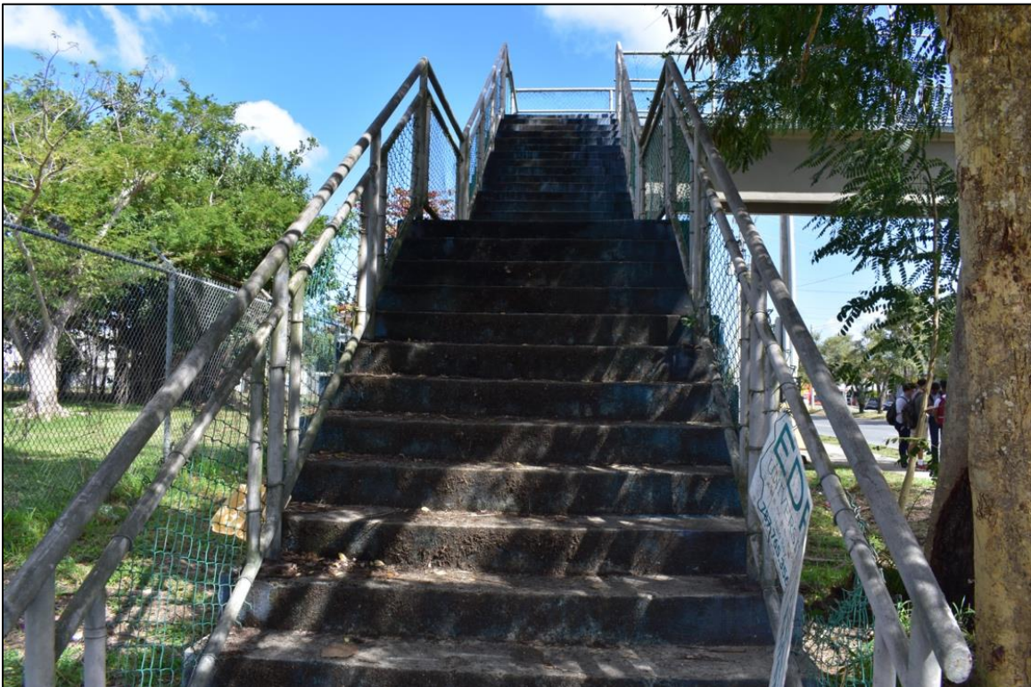
Figure 6.12: Mold on stairways of PB 1418
