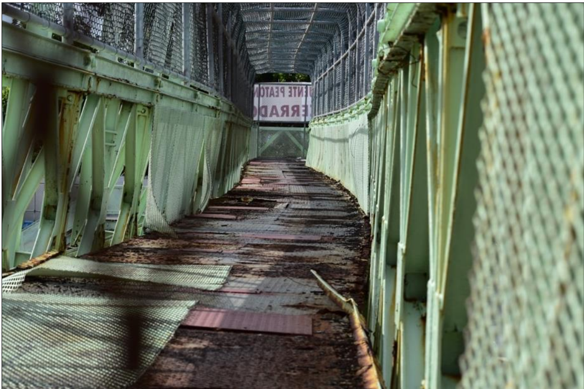
Figure 5.41: Curvature in deck
