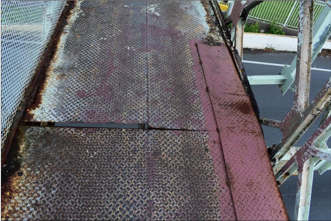
Figure 5.63: Detached plates
