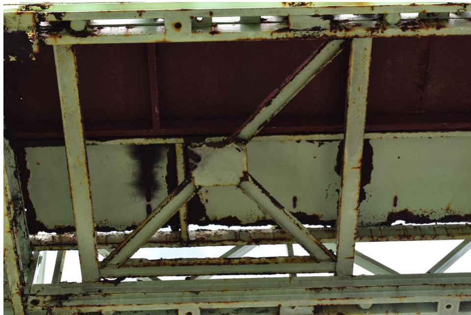
Figure 5.9: Missing Bracing Elements
