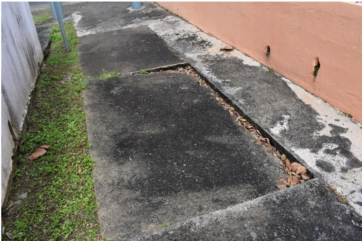
Figure 5.13: Sunk section of sidewalk
