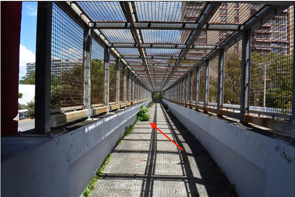
Figure 6.36: Vegetation covered drains on PB 2566
