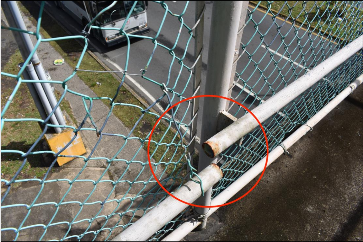
Figure 6.15: Broken railings on PB 1418
