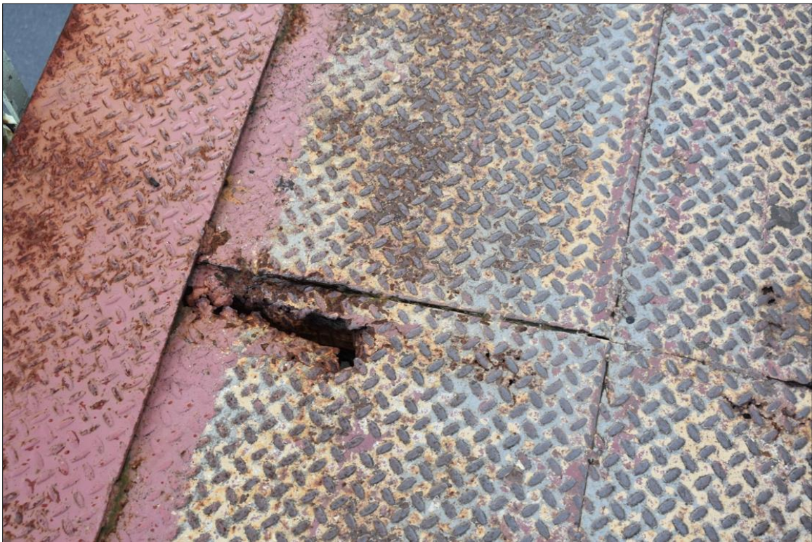
Figure 5.64: Hole in plates
