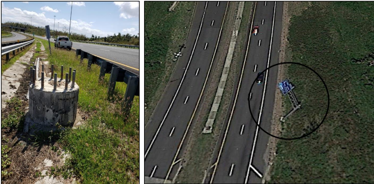
Figure 6-20: Cylindrical Precast Concrete Base that Experienced Torsional Rotation. The post was Removed. PR 66 in Canóvanas
