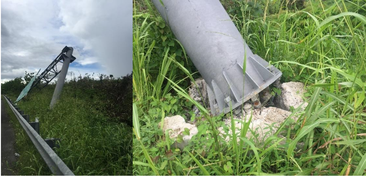
Figure 5-34: Photo of Cantilever Sign Foundation Structural Failures on the Pedestal at P-106
