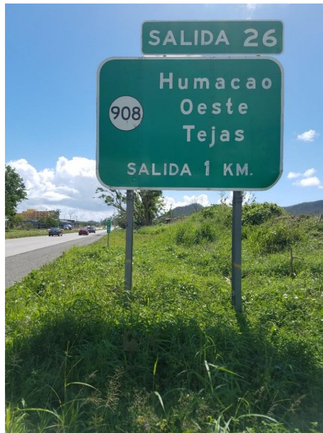
Figure 1.5: Guide sign with breakaway I-beams
