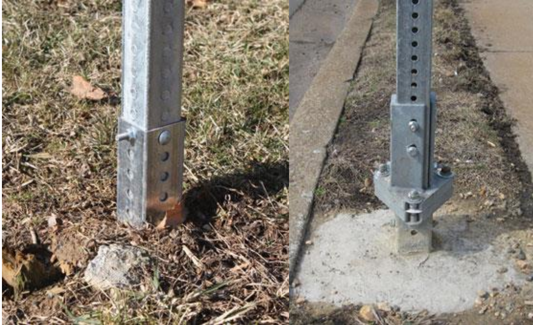
Figure 2.10: Breakaway designs for square tube posts (McGee, 2010)
