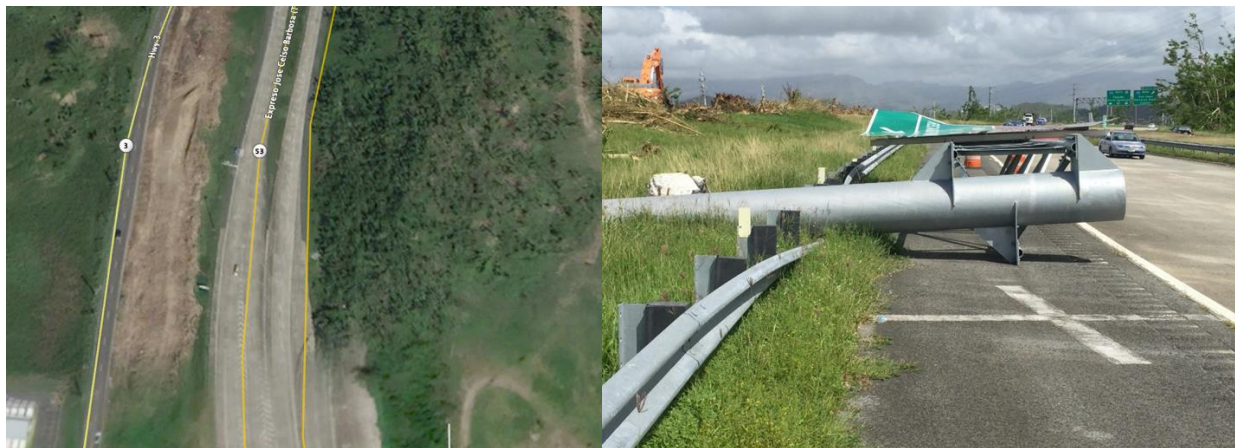
Figure 5-44: Photo of Cantilever Sign Structural Failures on the Pedestal at P-100 Location: 18°7'7.11"N; 65°49'16.812"W
