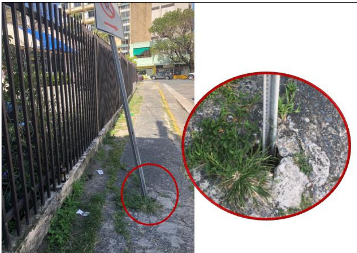
Figure 4.8: Example of Backfill concrete failure
