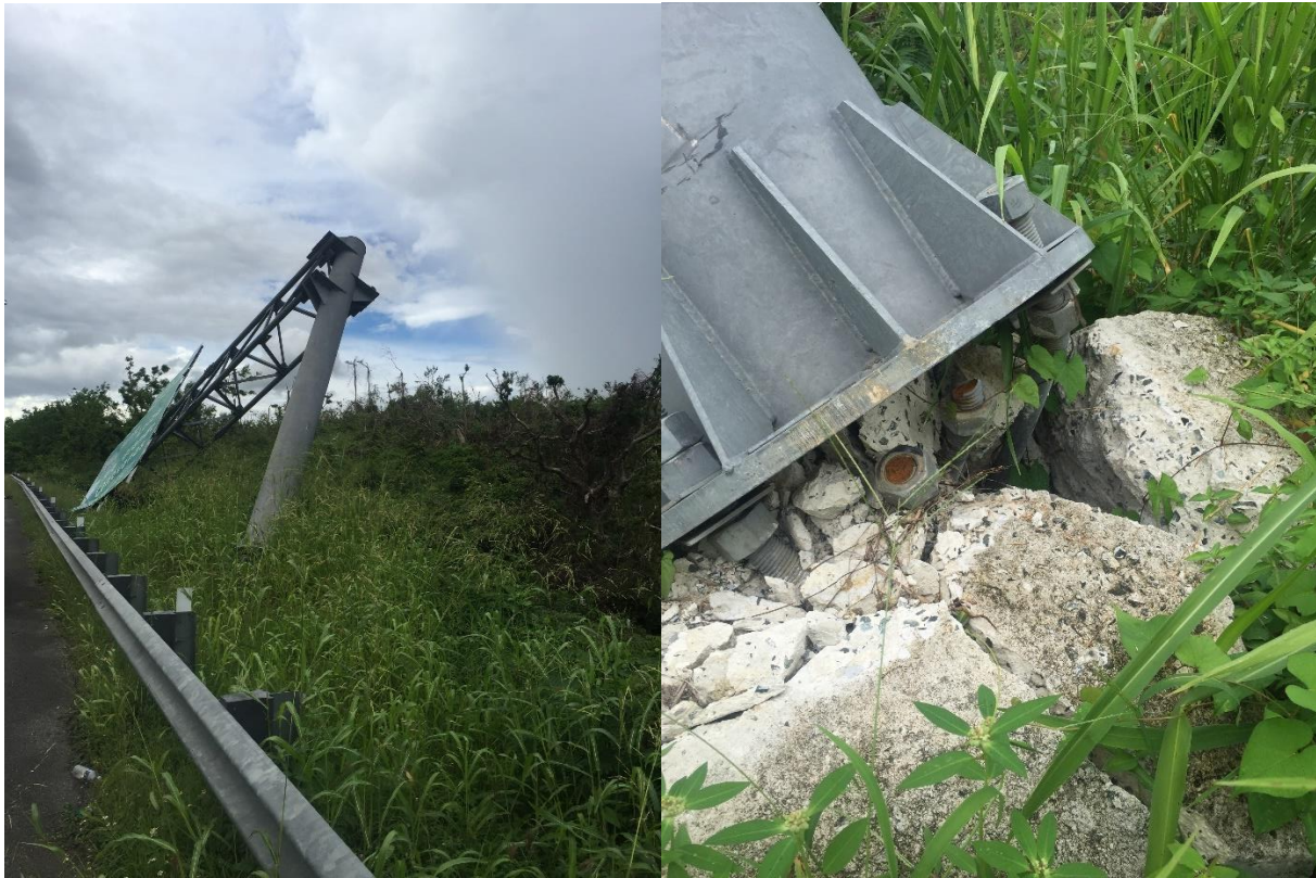
Figure 4-3: Total Collapse of a Cantilever Sign Located in PR-66 Highway
