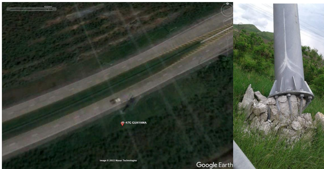
Figure 5-39: Photo of Cantilever Sign Foundation Structural Failures on the Pedestal and Sign Position (Partial Collapse) at P-47. Location: 17.9868529°N, -66.1425048°W
