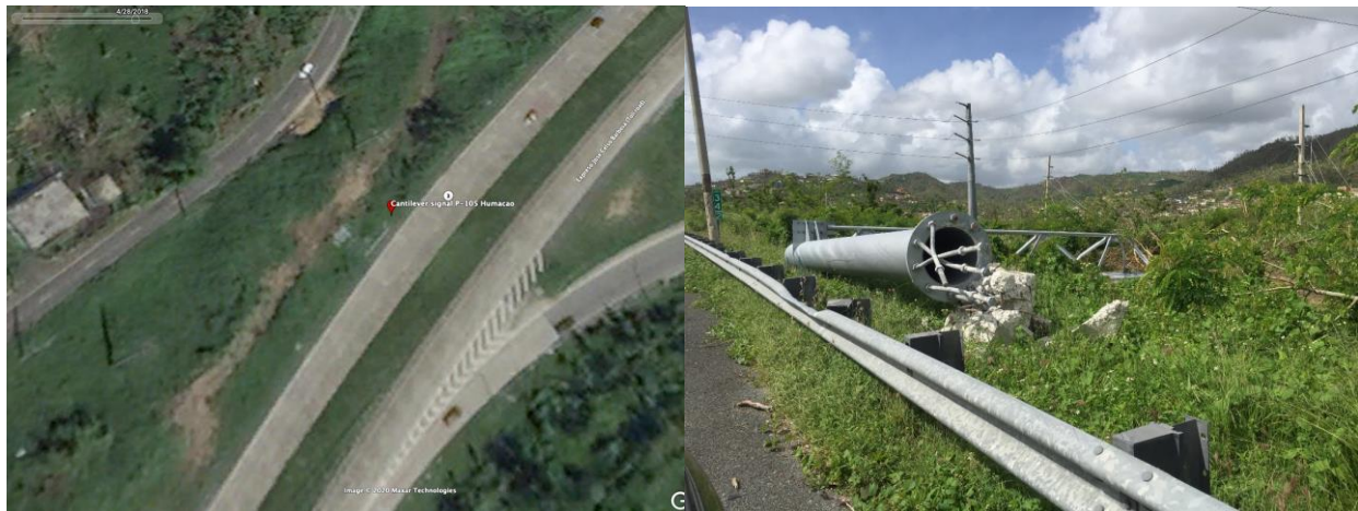
Figure 5-46: Photo of Cantilever Sign Structural Failures on the Pedestal at P-105 Location: 18° 7'20.00"N; 65° 49'12.23"W
