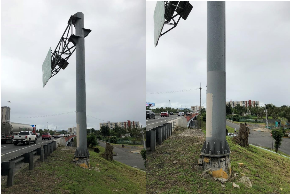
Figure 4-4: Partial Collapse and Damages on a Cantilever Traffic Sign Located on PR-18 Highway
