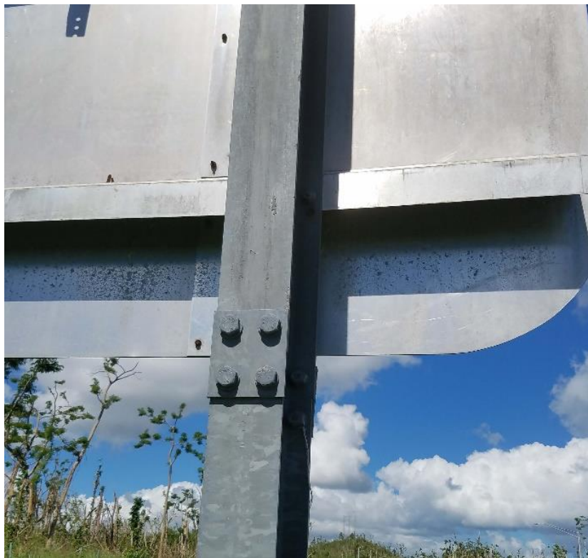
Figure 2.10: Hinge plate
