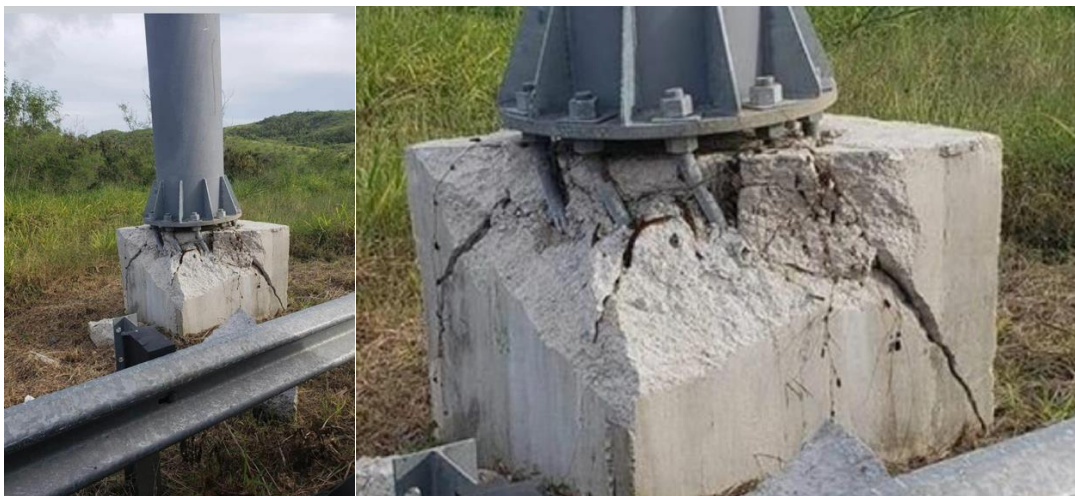
Figure 5-67: Photo of Cantilever Sign Foundation Structural Failure at P-15; Partial Collapse; the Post Presented Large Deflections and Double Bending in the Plastic Range of the Anchoring Elements
