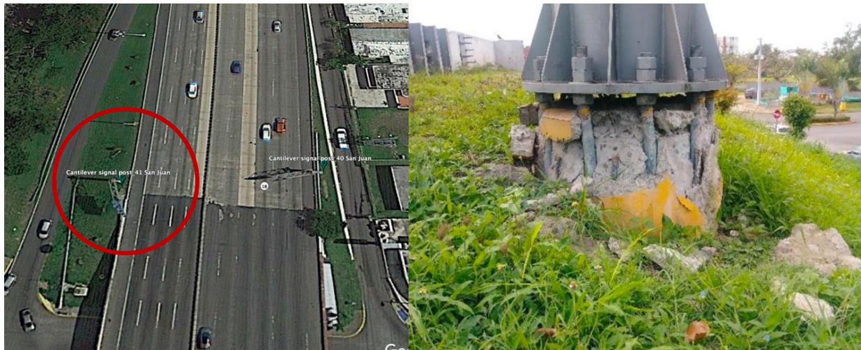
Figure 5-72: Photo of Cantilever Sign Soil Foundation Failure (Torsional Rotation) with Damages to the Pedestal at P- 41 Photo Location: 18°24'47.01"N; 66° 4'13.07"W
