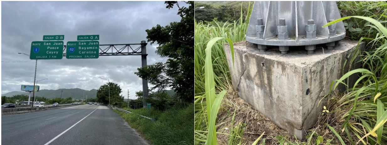
Figure 5-30: Photos of Cantilever Traffic Sign Location and Anchor Bolts Lateral Movement Producing Cracks on the RC Base at P-58. Location: 18.25564167N; -66.02865278W
