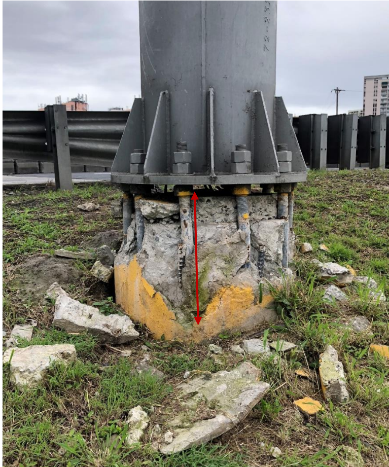
Figure 6-5: More Advance Stage of Concrete Cracks and Spalls due to Lateral Deflections of Anchor Bolts with Large Unconfined Length (Sign P-41)
