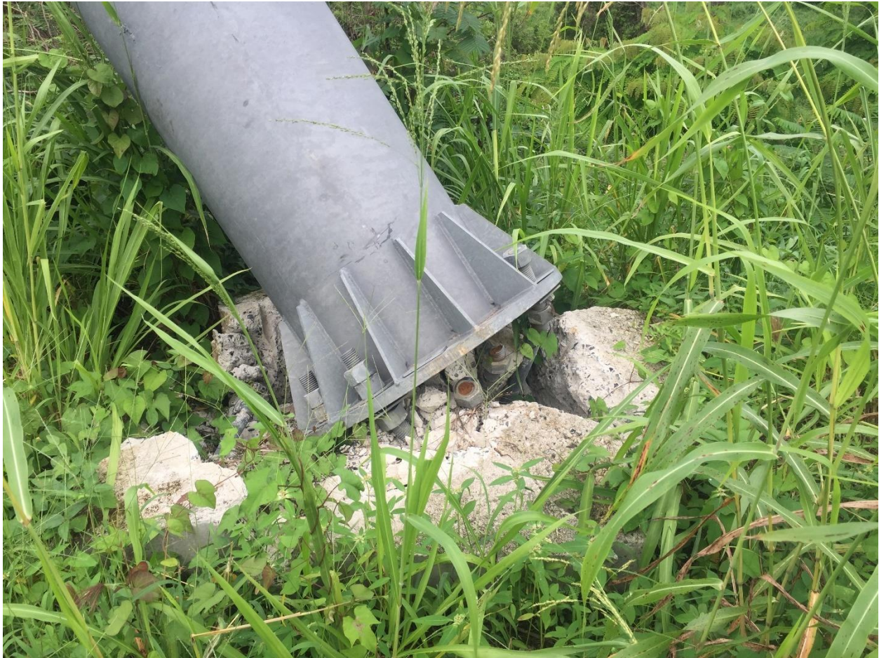
Figure 6-11: Large Deflections of Anchor Bolts due to Lack of Lateral Confinement (Sign P-106)
