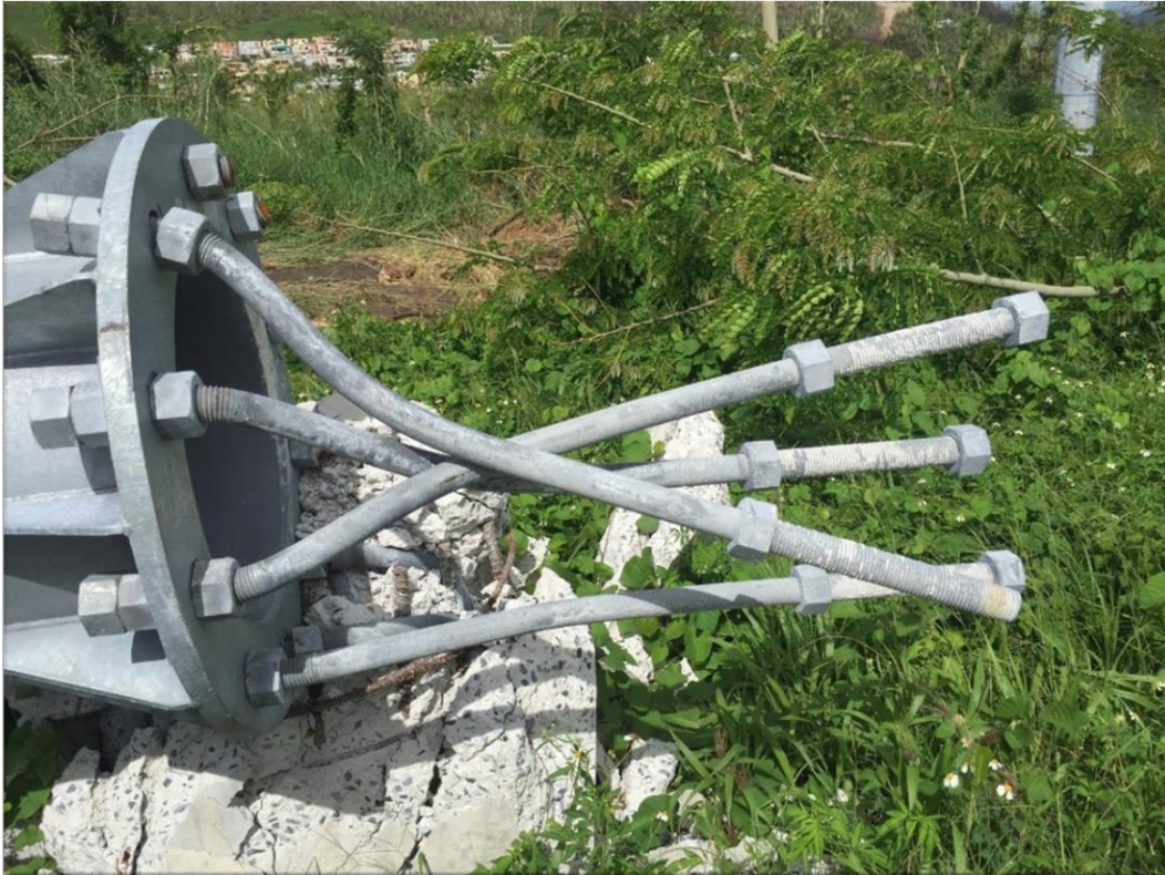
Figure 6-16: Anchor Bolts Pullout (Sign P-105)
