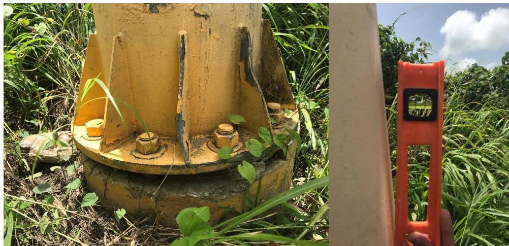
Figure 5-6: Photos of Cantilever Traffic Sign Pedestal Failures and Post Inclination at P-76
