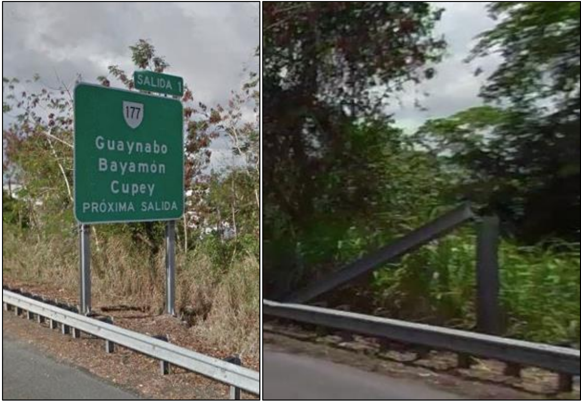
Figure 4.11: Sign 11 before and after failure (Source: Google Maps)
