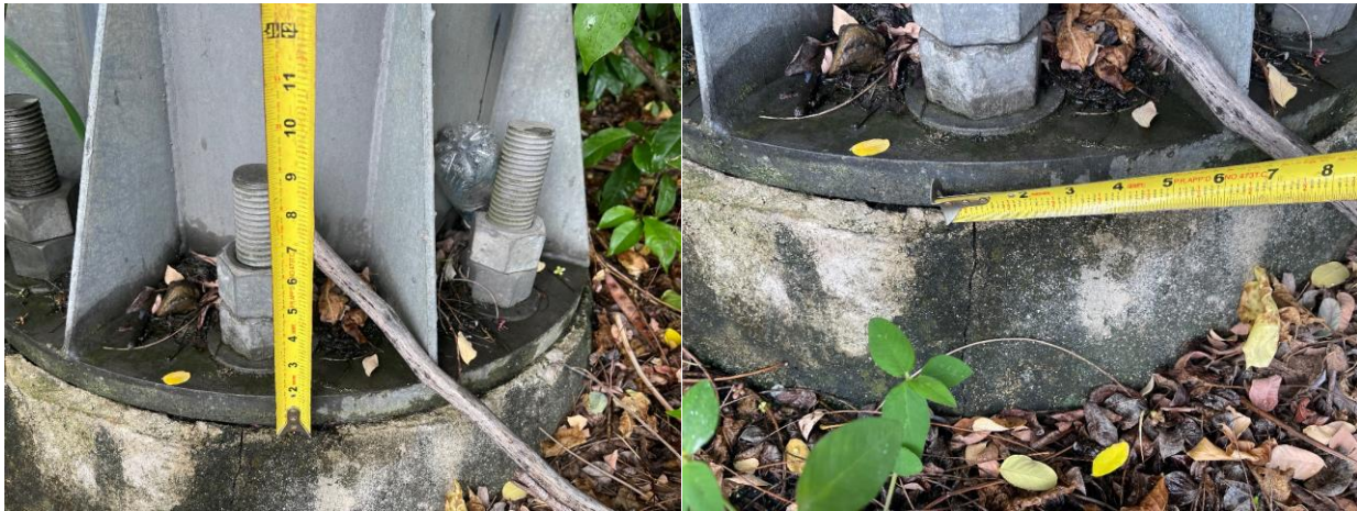
Figure 5-25: Photos of Cantilever Traffic Sign Base Condition at P-16. Location: 18.22014722 N; -66.04703611 W.
