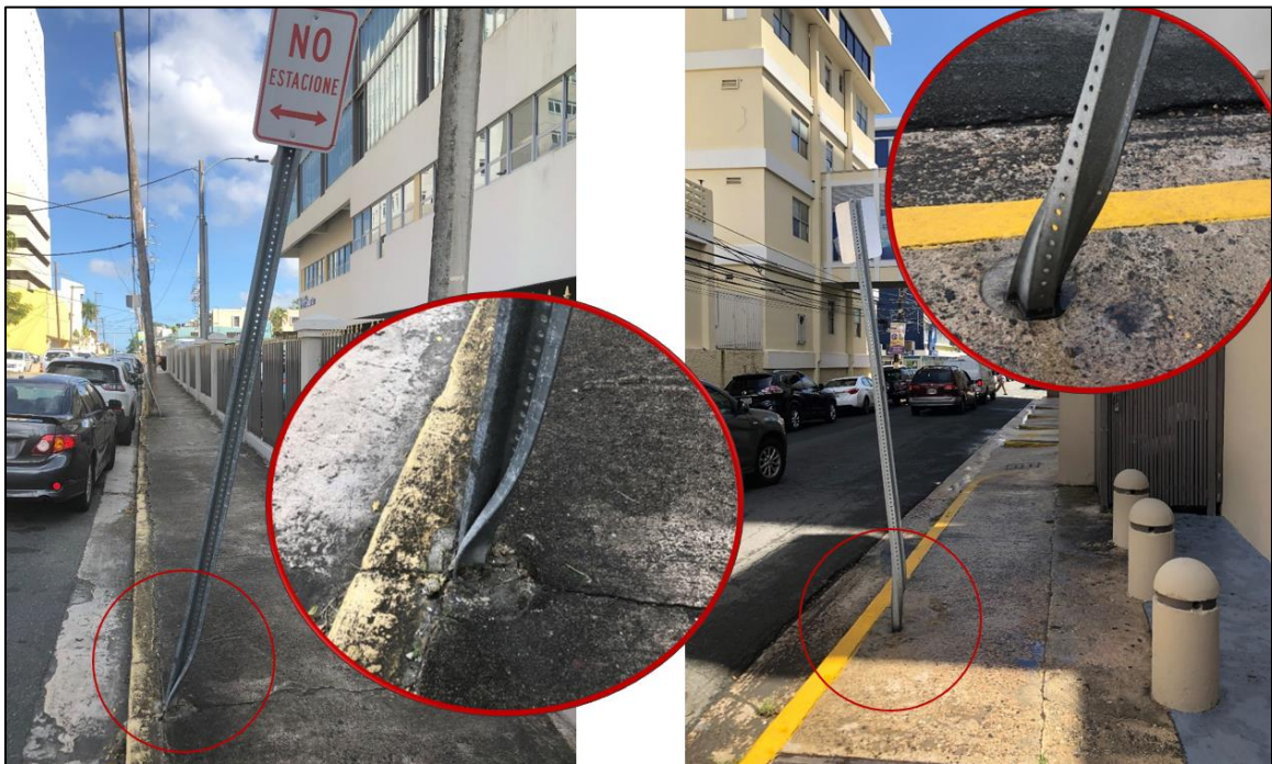
Figure 4.10: Examples of permanent twisting deformation
