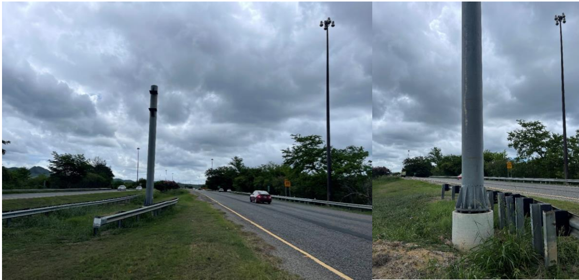
Figure 5-49: Photo of Cantilever Sign Missing Truss and Sign at P-6 Location: 18.03189444°N; 66.45465278°W
