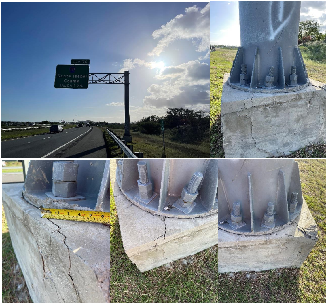
Figure 5-82: Photo of Cantilever Sign Location and Pedestal Cracks at P-10 Photo Location: 18.01423056°N; 66.36989167°W
