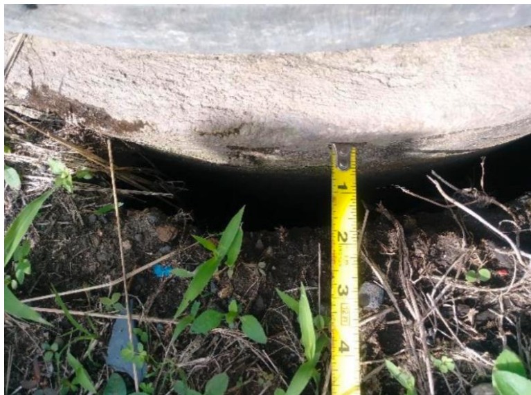
Figure 5-78: Gap Around the Circumference of the Drilled Shaft
