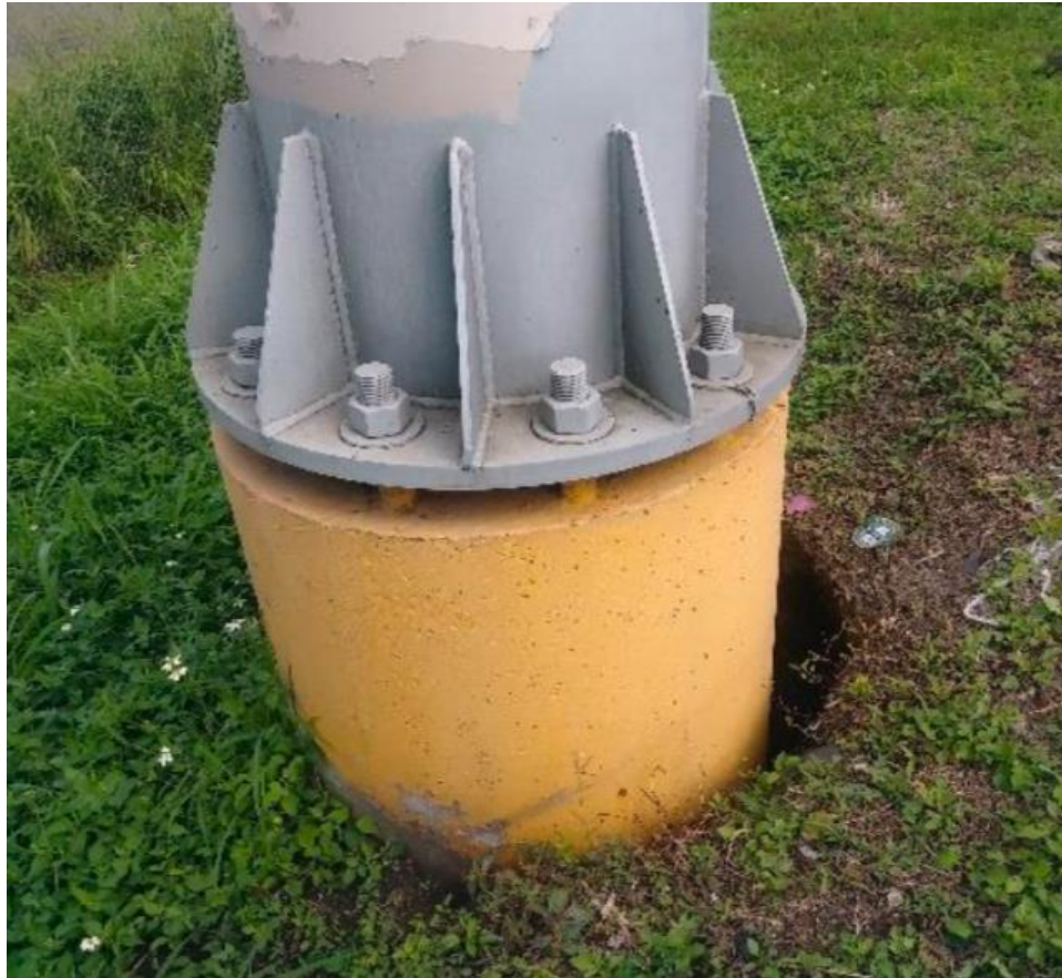
Figure 6-22: Gap Between the Soil and the Cylindrical Precast Concrete Base that Experienced Torsional Rotation. PR 18 in San Juan.
