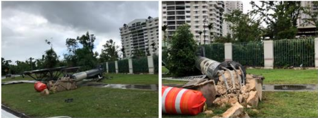
Figure 5-79: Photo of a Collapsed Cantilever Sign Foundation due to Structural Failures on the Pedestal at P-98 Location: 18°24'27.38"N; 66° 4'3.00"W
