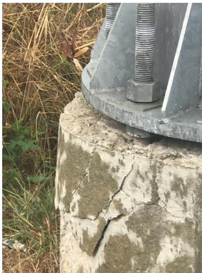
Figure 6-2: Initial Stages of Concrete Cracks and Spalls due to Lateral Deflections of Anchor Bolts (Sign P-3)
