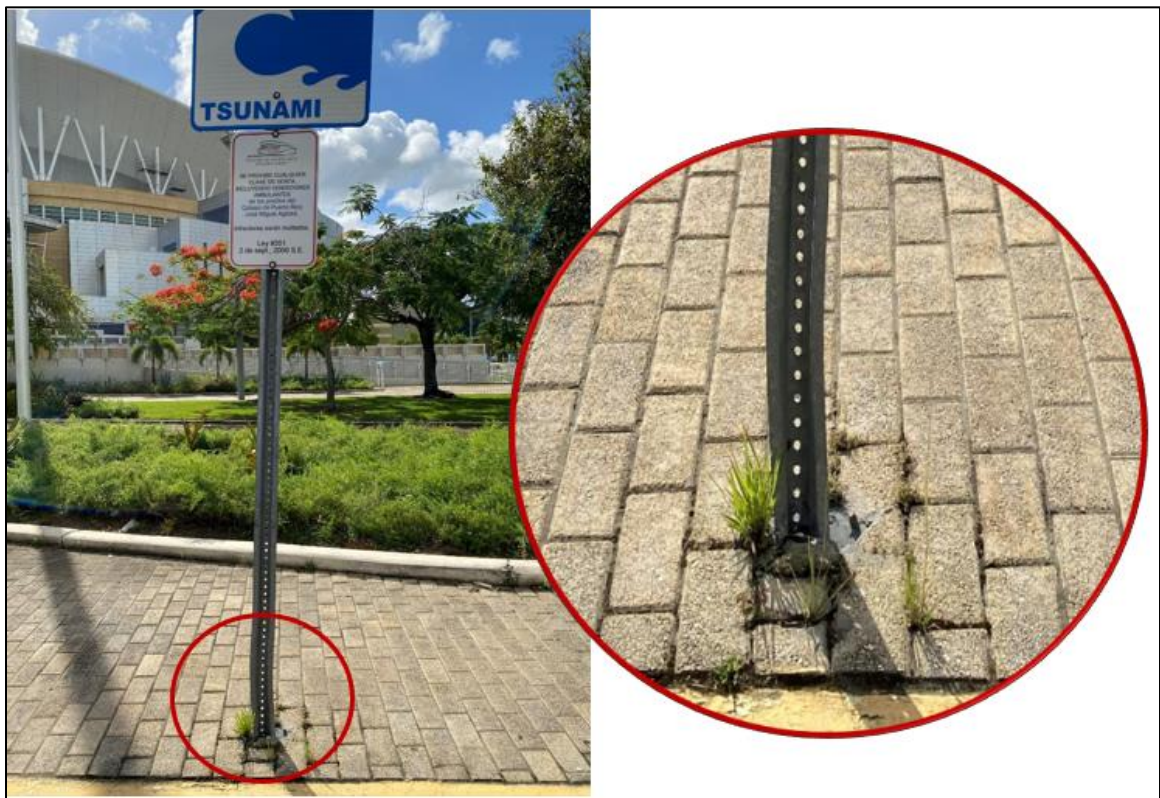
Figure 4.17: U-channel top post without a visible base post
