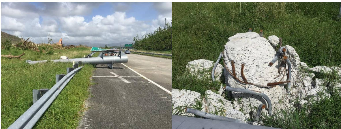
Figure 4-2: Collapsed Cantilever Sign in PR-30 Highway
