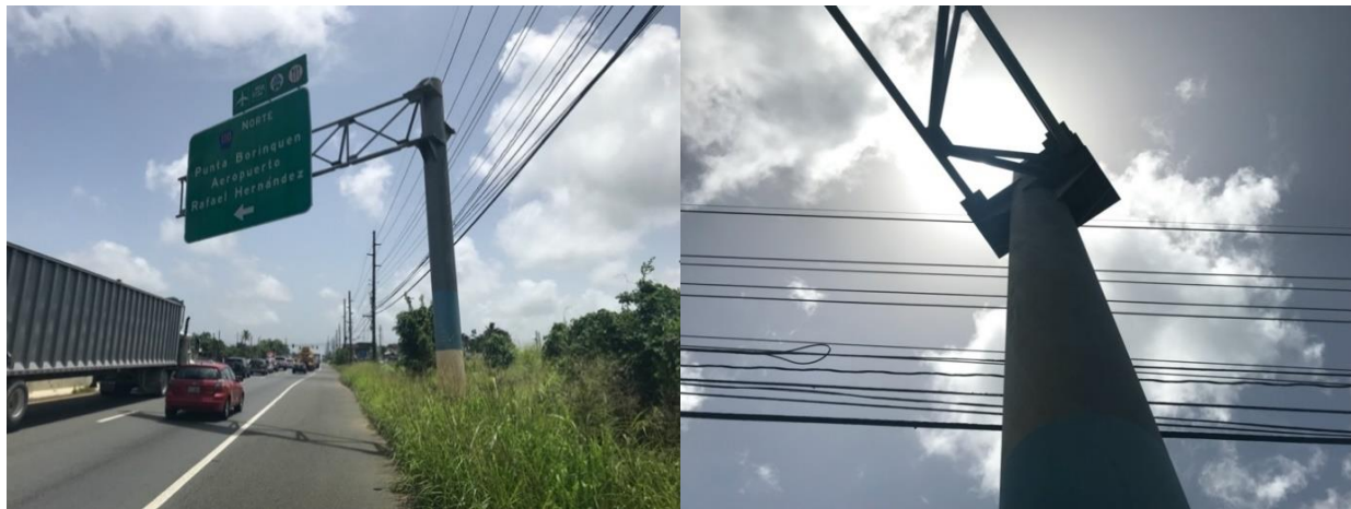
Figure 5-5: Photos Showing the Rotation of the Traffic Sign at P-76 Location: 18°27'8.10"N; 67° 5'38.06"W
