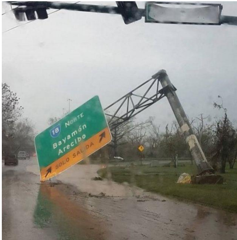
Figure 4-6: Overhead Cantilever Traffic Sign Collapse on PR-17 (Lima, 2017)
