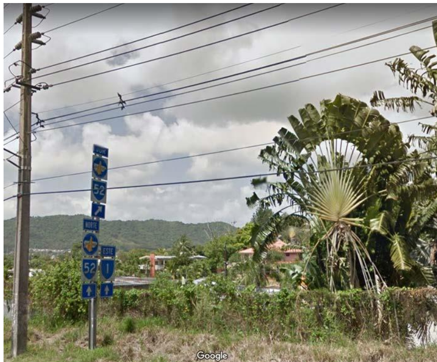
Figure 2.7: Single post ground-mounted breakaway sign (Source: Google Maps)
