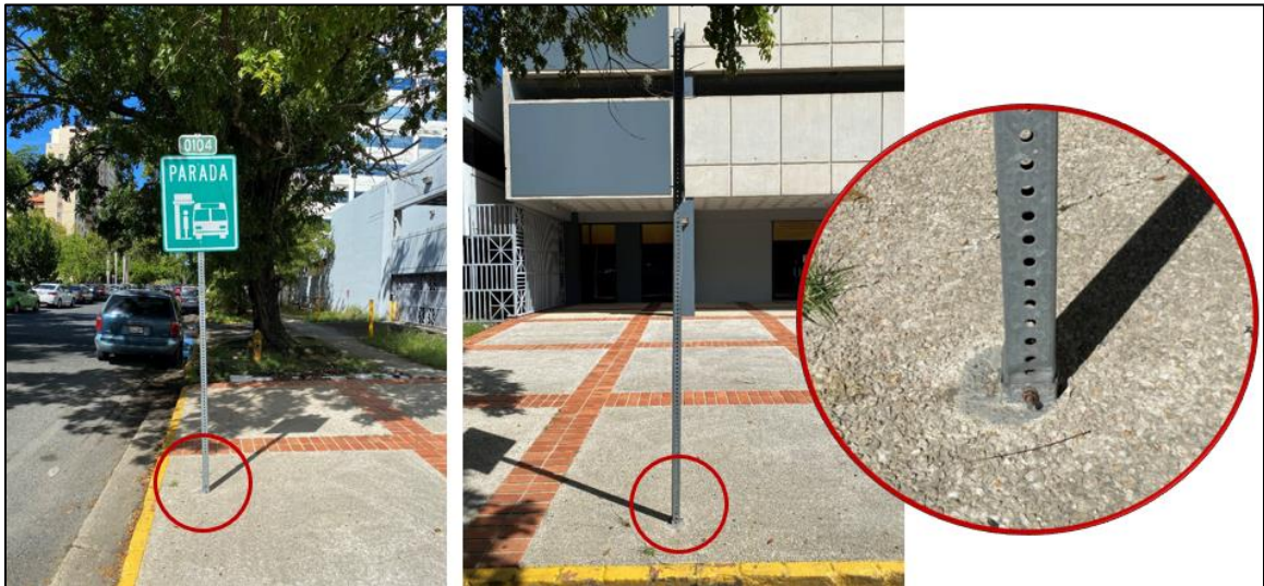
Figure 4.3: Square exhibiting plasticization at the base
