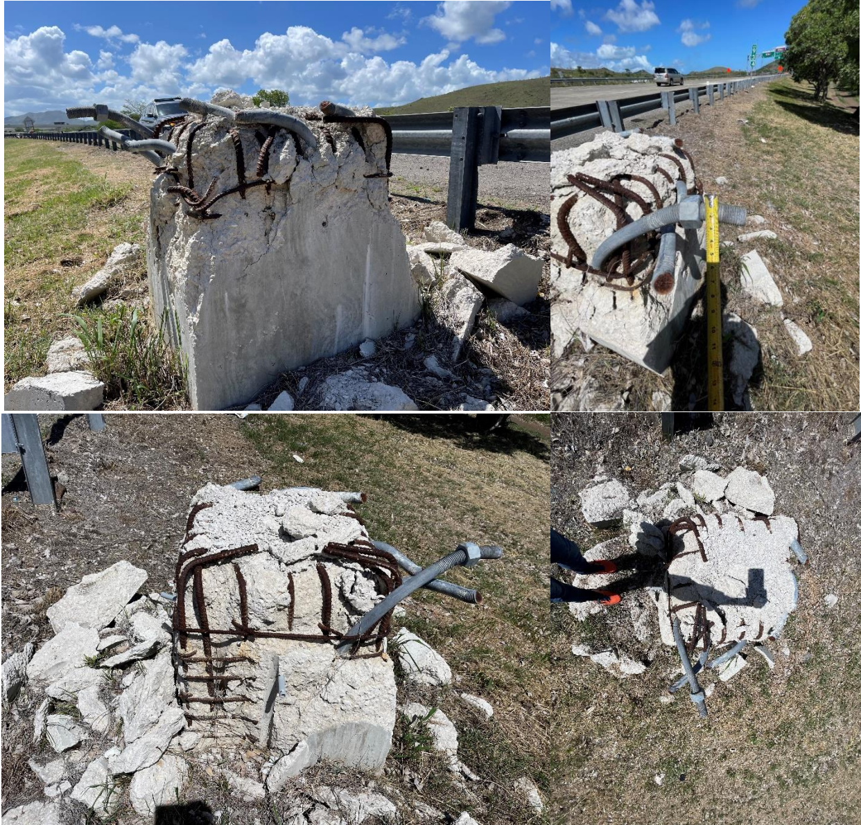
Figure 5-65: Photo of Cantilever Sign Structural Foundation Failure at P-12; Collapsed Post Presented Torsional Pattern and Large Deflections of the Anchoring Elements, which also Exhibit Shear Fracture
