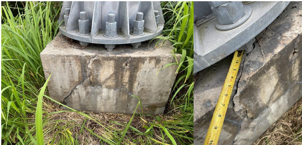
Figure 5-31: Additional Details of RC Base Damages due to Anchor Bolts Lateral Displacements at P-58
