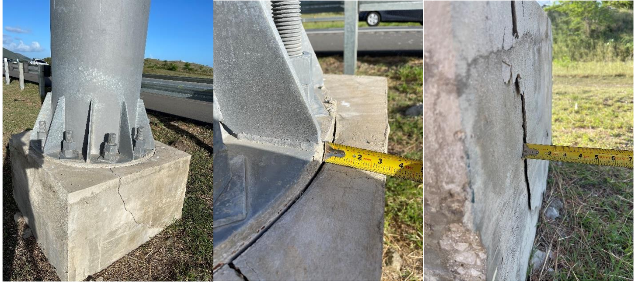
Figure 5-83: Photo of Cantilever Sign Location Pedestal Cracks at P-10
