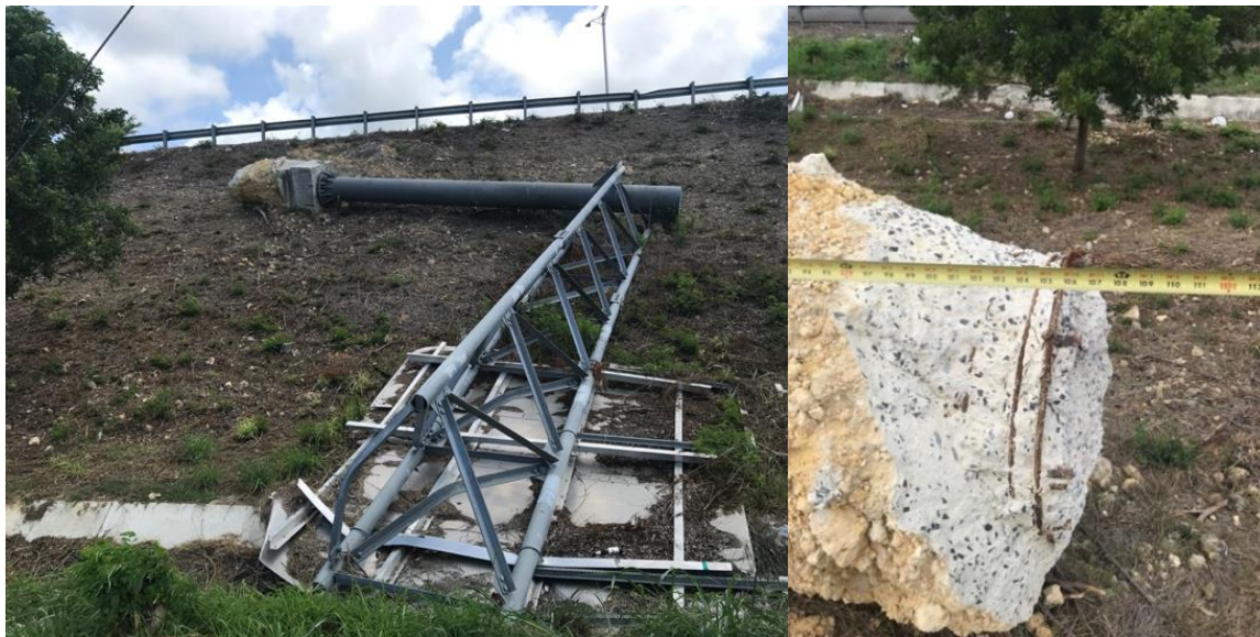
Figure 5-60: Photo of Cantilever Sign Foundation Soil and Structural Failure at P-59. Location: 17°59'21.23"N; 66°38'46.49"W
