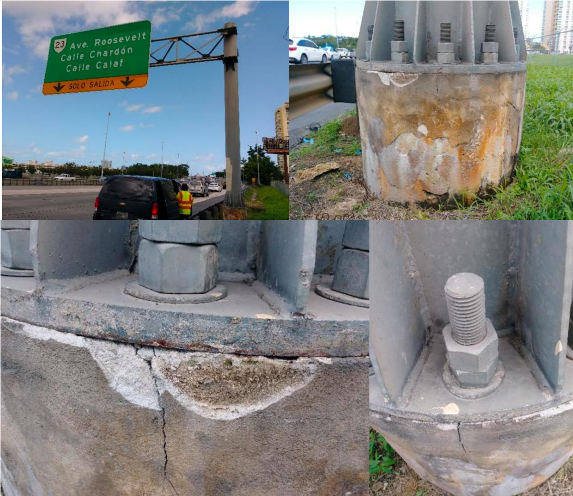
Figure 5-76: Photo of Cantilever Sign Foundation Failure (Torsional Rotation), Damages to the Concrete Pedestal, and Small Gap Between Soil and Shaft at P- 43 Photo Location: 18.41561389°N; 66.06995°W
