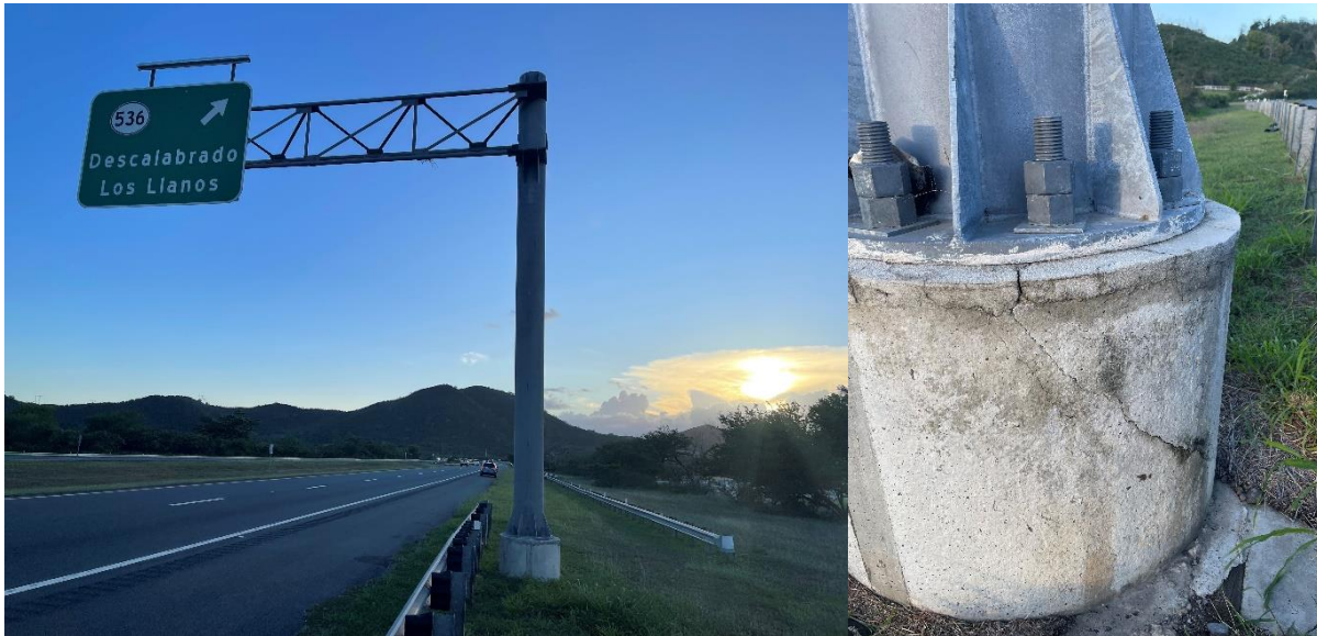
Figure 5-85: Photo of Cantilever Sign Location and Pedestal Cracks at P-70 Photo Location: 18.0284609°N; 66.4165331°W
