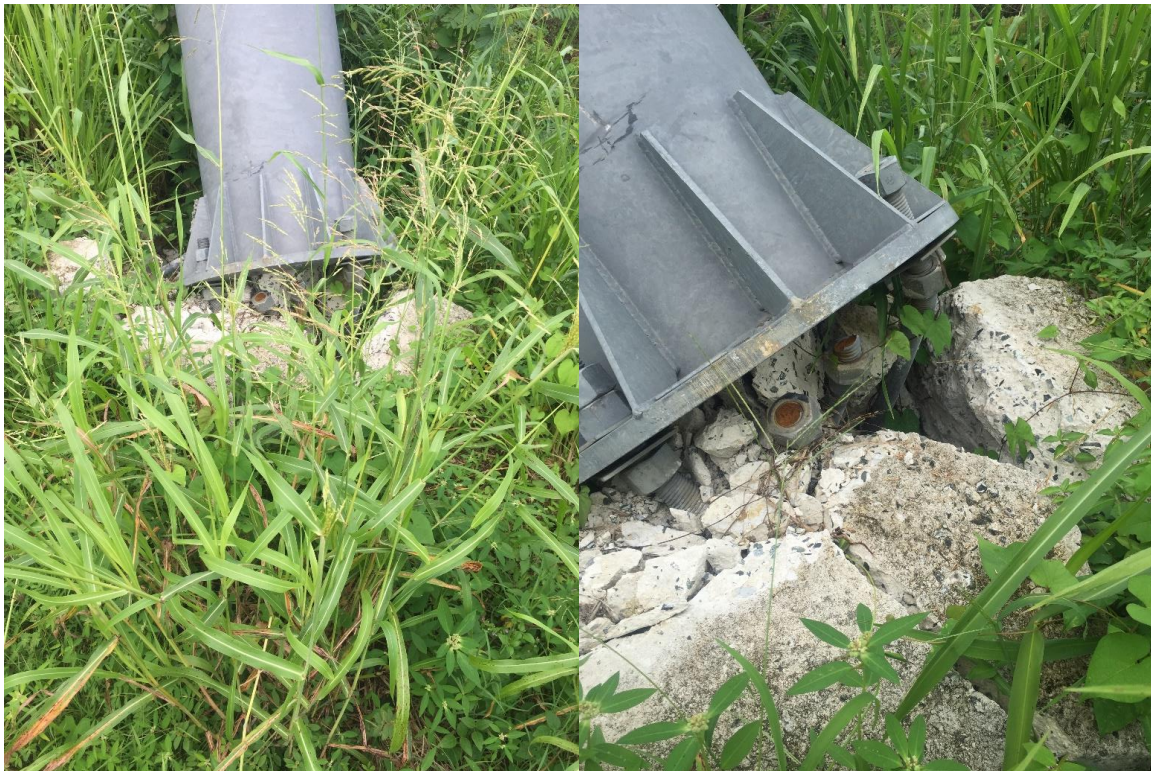
Figure 5-35: Photo of Cantilever Sign Foundation Structural Failures on the Pedestal at P-106
