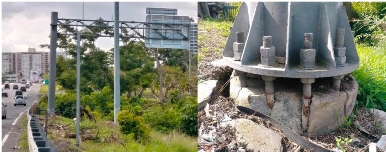
Figure 5-70: Photo of Cantilever Sign Soil Foundation Failure (Torsional Rotation) with Damages to the Pedestal at P- 38 Photo Location: 18°24'5.58"N; 66° 4'16.57"W
