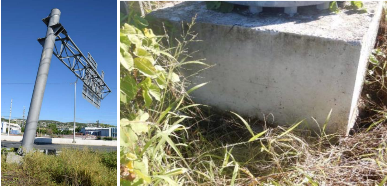
Figure 5-62: Photo Showing the Rotation of The Traffic Sign and the Foundation Pedestal at P-94
