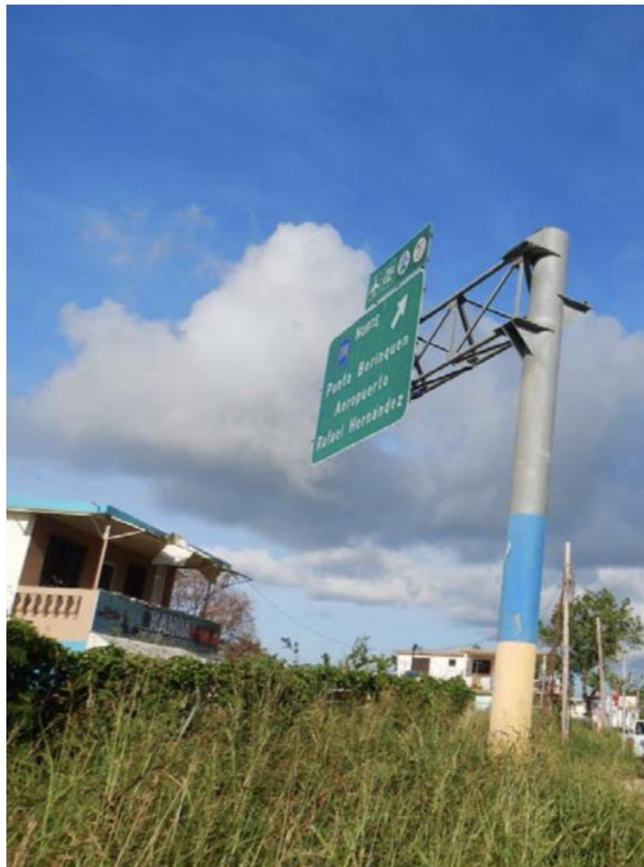
Figure 5-7: Photo of Cantilever Sign Foundation Failure at P-77 with Location: 18°27'13.01"N; 67° 5'20.87"W
