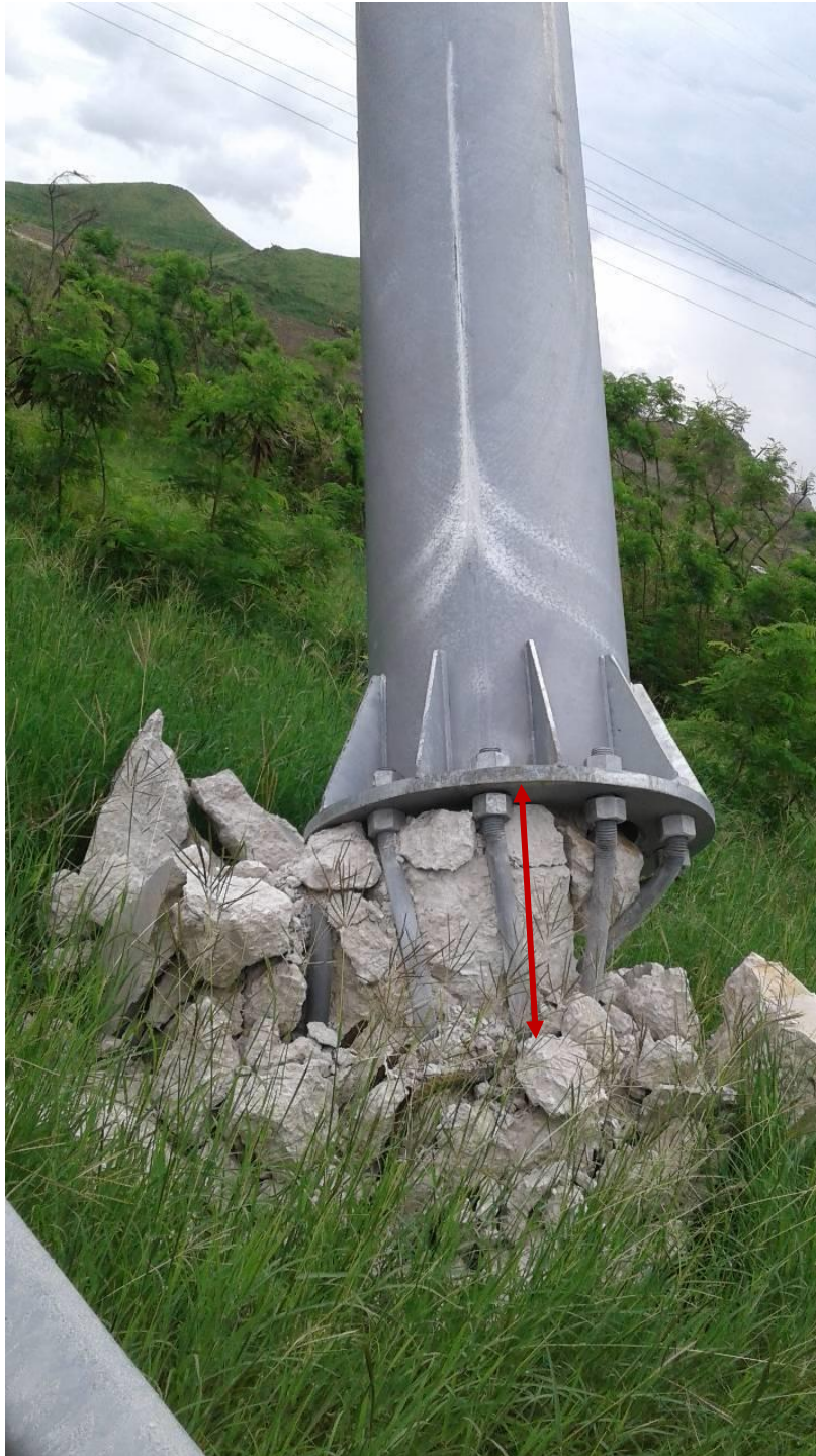
Figure 6-8: Large Deflections of Anchor Bolts due to Lack of Lateral Confinement
