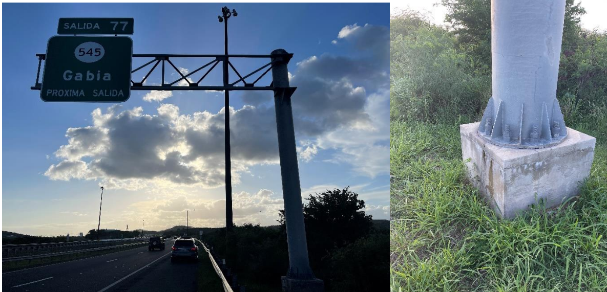
Figure 5-84: Photo of Cantilever Sign Location and Pedestal Cracks, Efflorescence, Water Marks and Leakage at P-36 Photo Location: 18.01324444°N; 66.38875°W
