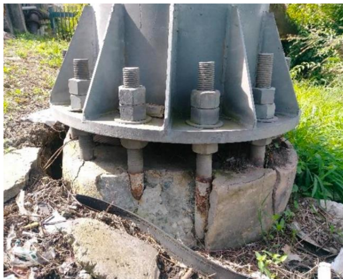
Figure 6-4: More Advance Stage of Concrete Cracks and Spalls due to Lateral Deflections of Anchor Bolts with Large Unconfined Length (Sign P-38)
