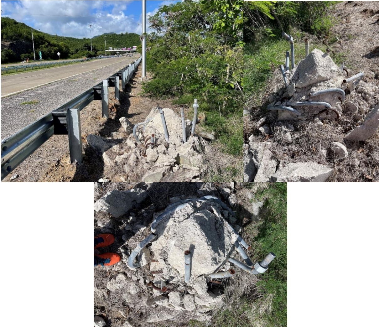
Figure 5-40: Photos of Cantilever Traffic Sign Foundation Structural Failure to the Pedestal at P-47; with Large Deflections and Bending on the Plastic Range and Shear Fracture of the Anchor Elements, and Fractures, Detachments and Crushing of the Concrete. Bolts outside the confinement of Stirrups
