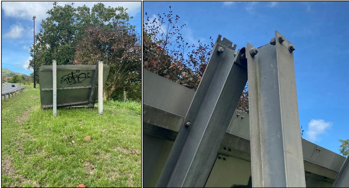
Figure 4.4: Slotted fuse plate slippage failure of Sign 9
