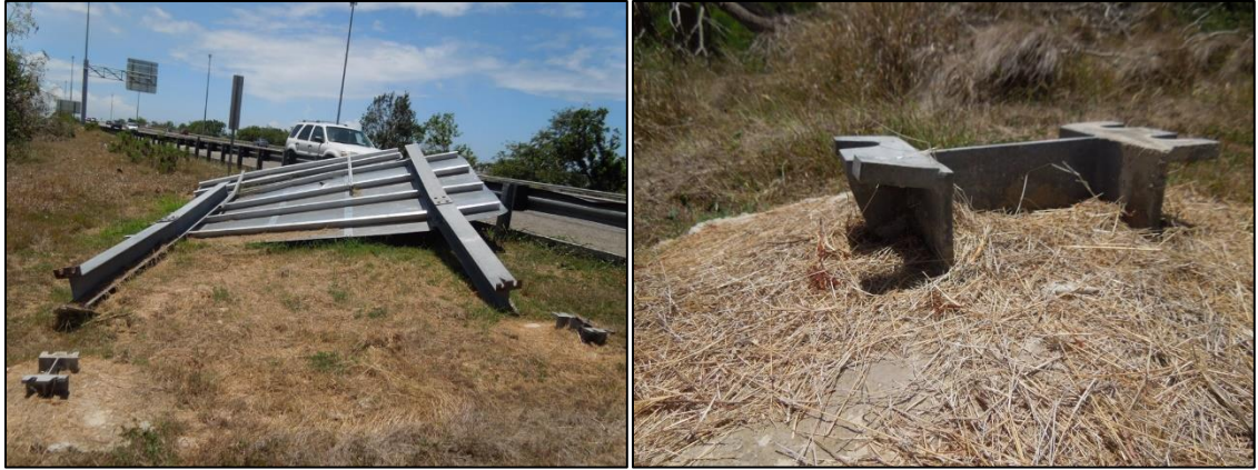
Figure 4.7: Slippage failure at the base of Sign 4
