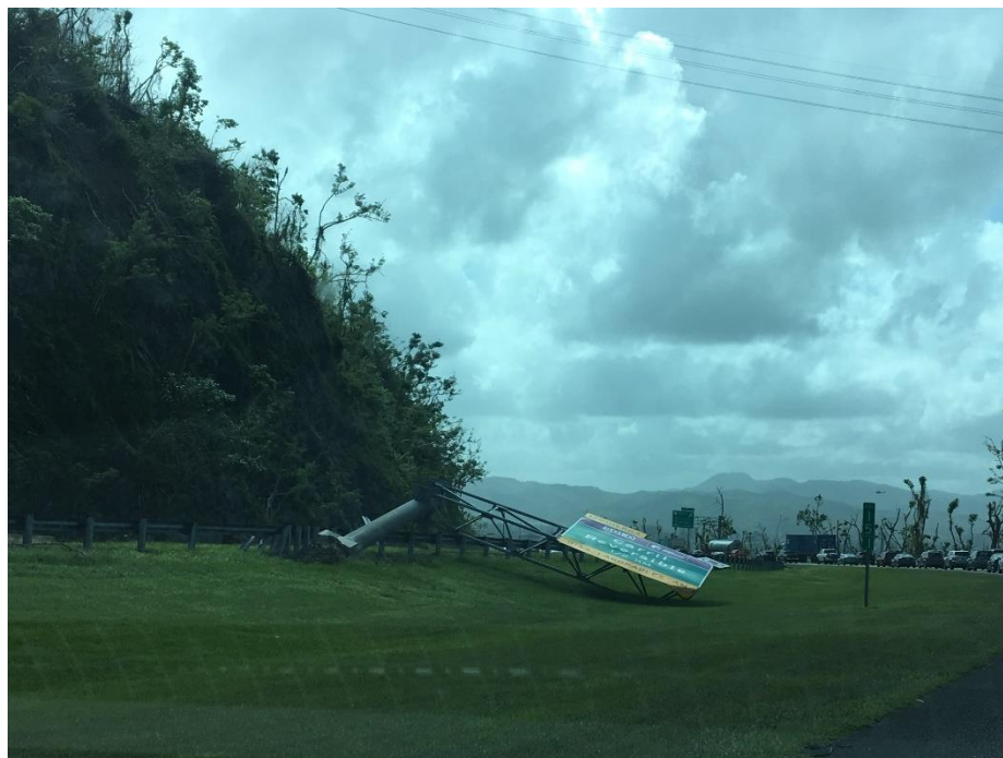
Figure 1-5: Example of Overhead Cantilever Sign Failure due to Hurricane Maria
