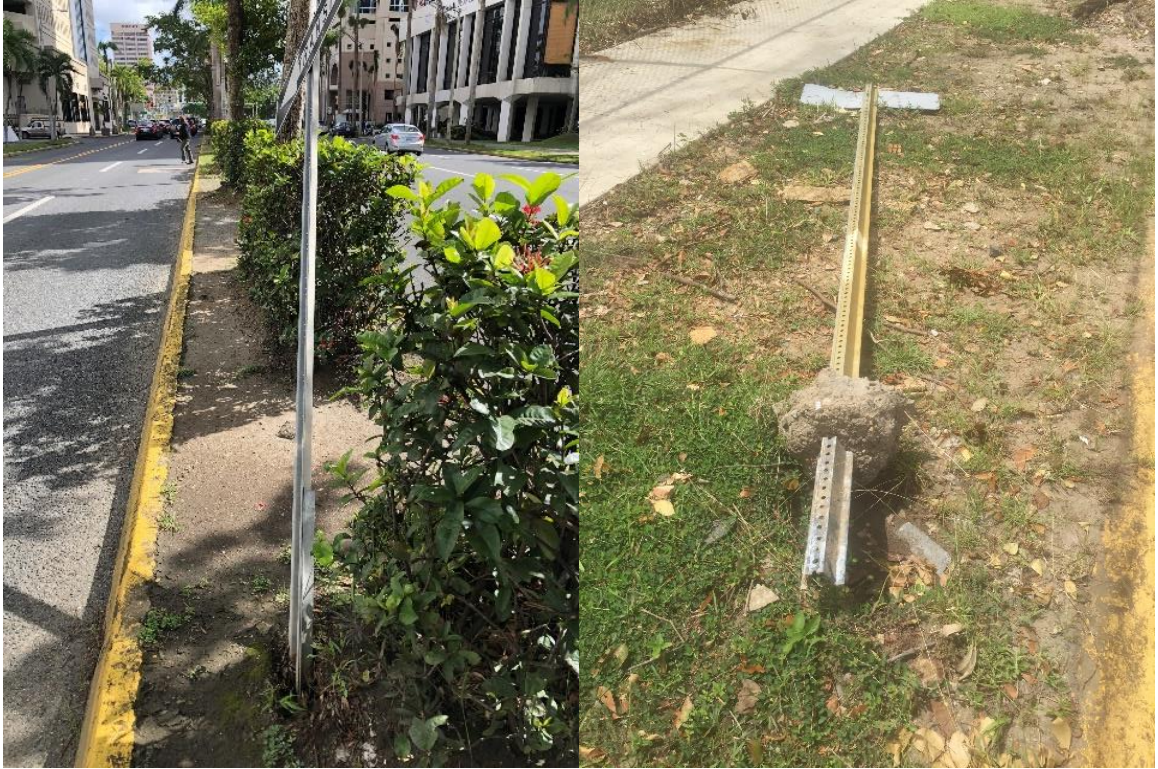
Figure 4.7: Examples of foundation on soil failure
