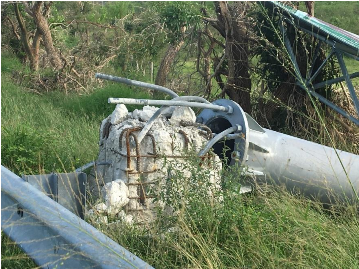
Figure 6-15: Anchor Bolts Pullout
