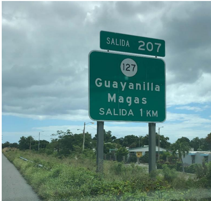
Figure 2.6: Dual post ground-mounted breakaway sign
