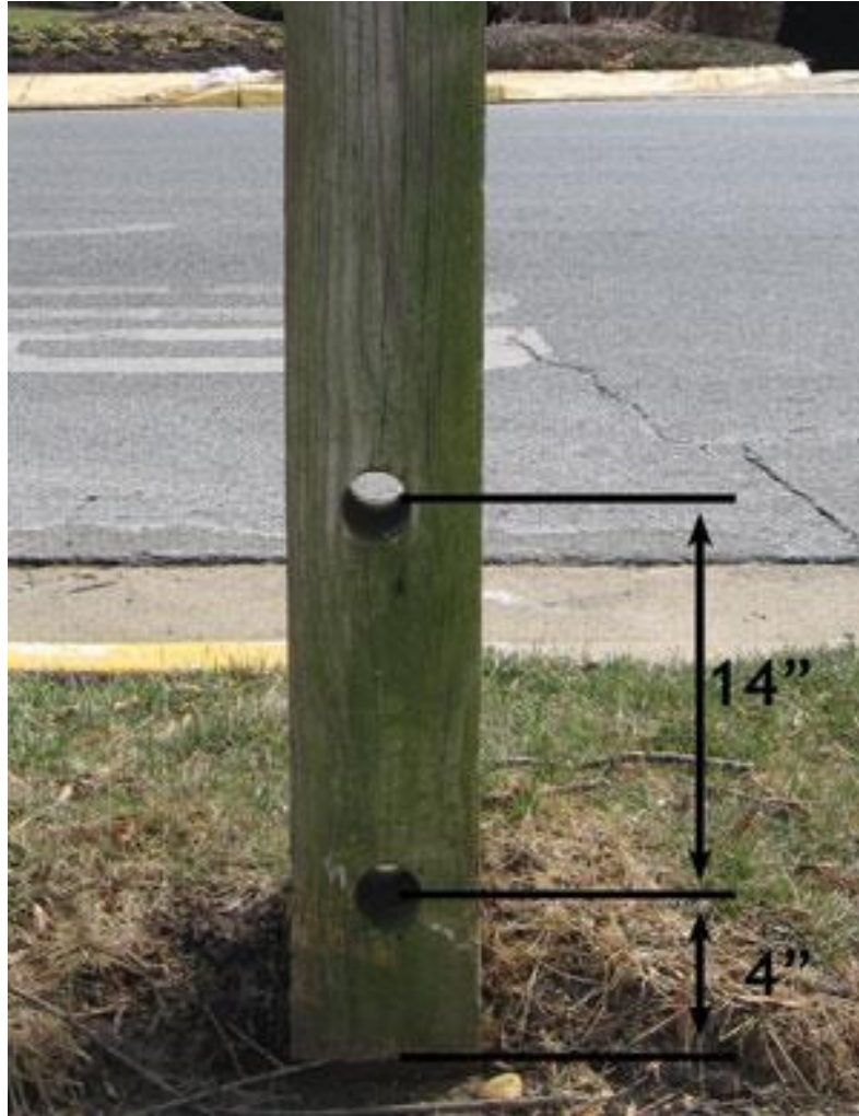
Figure 2.6: Holes to provide breakaway capability (McGee, 2010)
