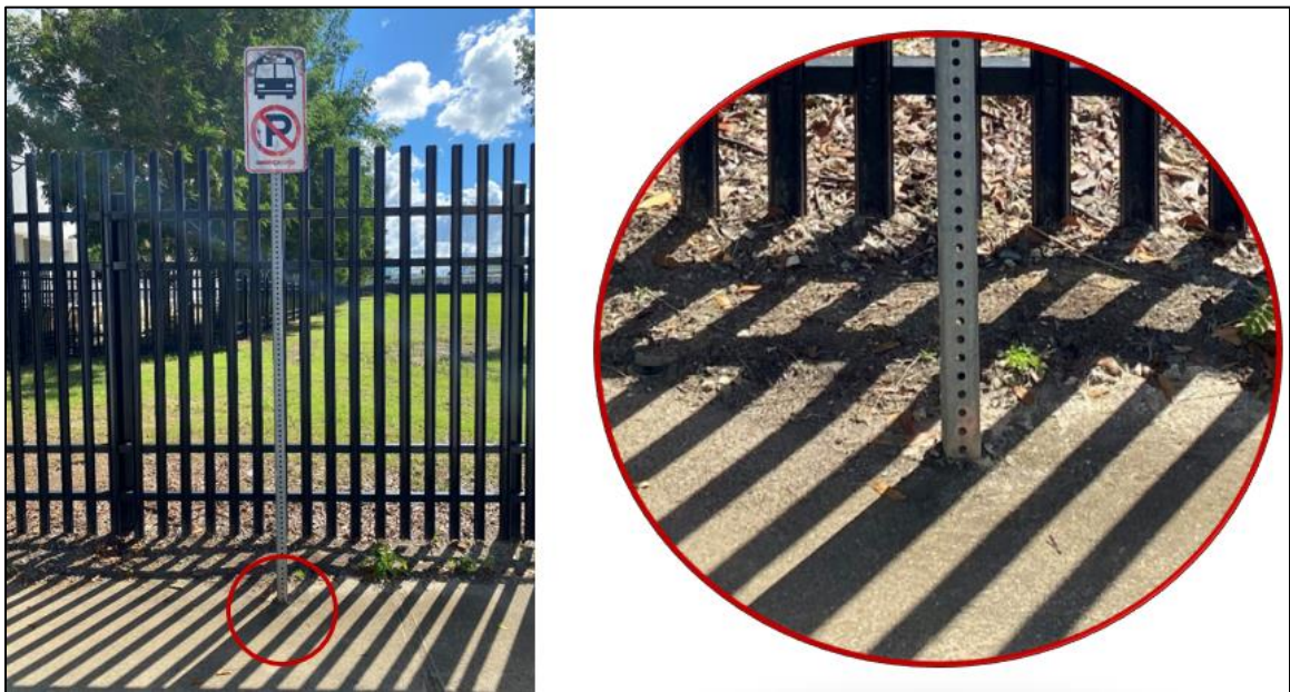
Figure 4.5: Top post without a visible base post
