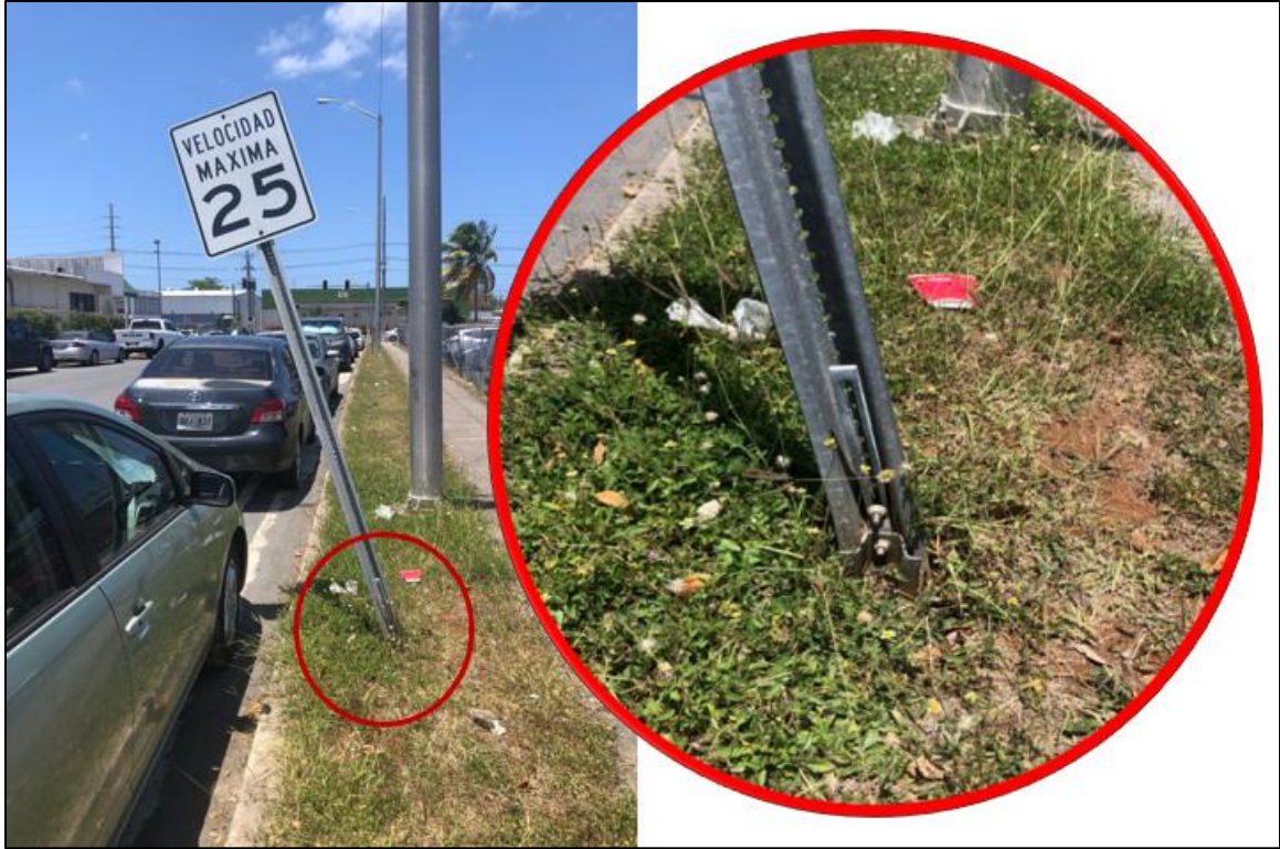
Figure 4.9: Example of retainer strap deformation
