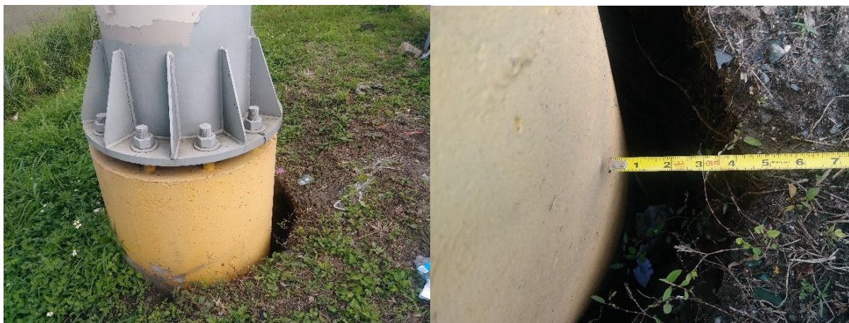
Figure 5-74: Gap Around the Circumference of the Drilled Shaft, and Soil Movement Downhill
