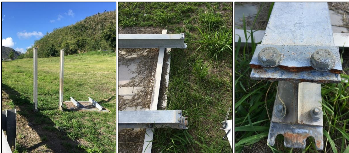
Figure 4.5: Slotted fuse plate slippage failure of Sign 7
