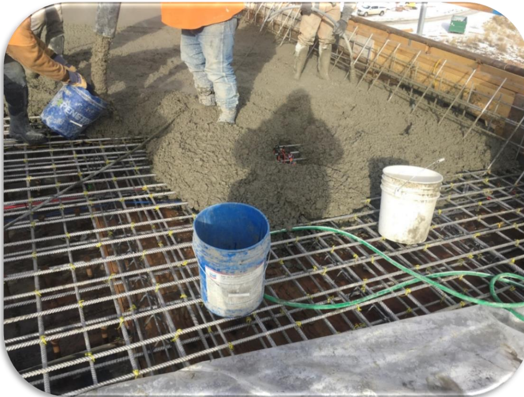
Figure 75. Concrete being deposited around WJE sensor location and sampling.
