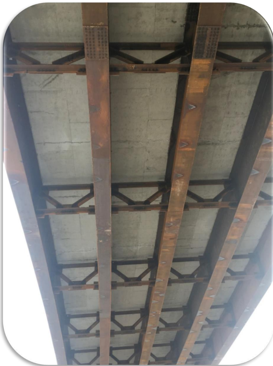
Figure 42. Underside of Rarus Structures - Silver Bow Creek - Bridge C - 2019 inspection.
