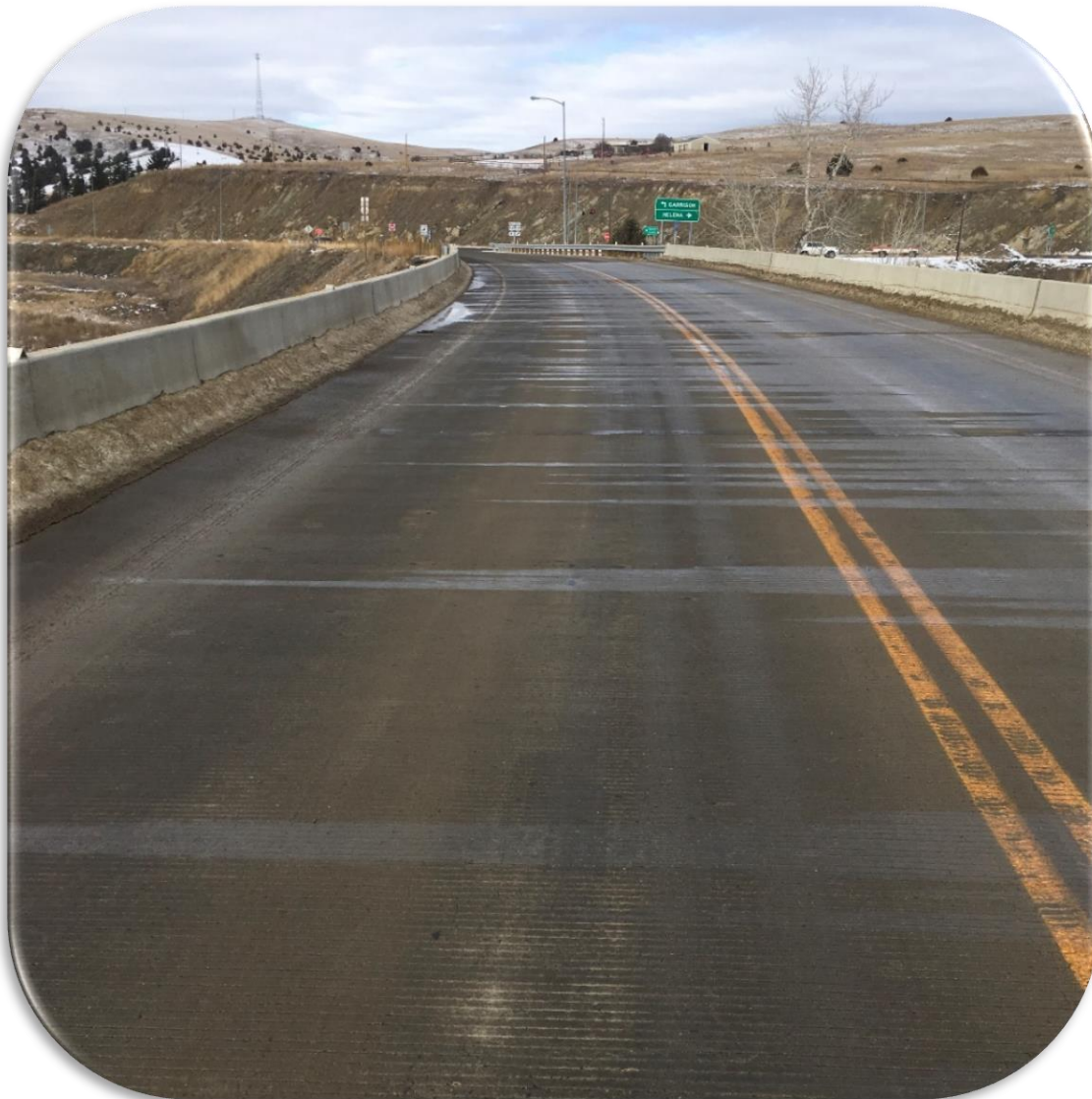
Figure 13. Garrison Bridge - 2019 inspection - Typical deck topside condition.
