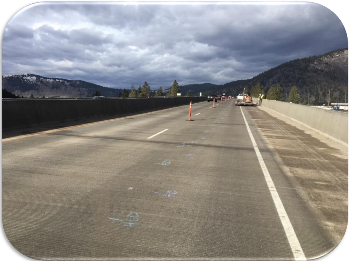
Figure 35. Bonner Bridge Phase II (WB)- Typical deck topside condition, placement 1.
