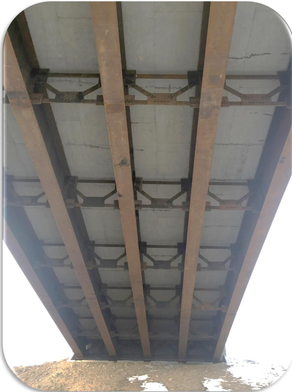
Figure 43. Underside of Rarus Structures - Silver Bow Creek - Bridge C - 2019 inspection.
