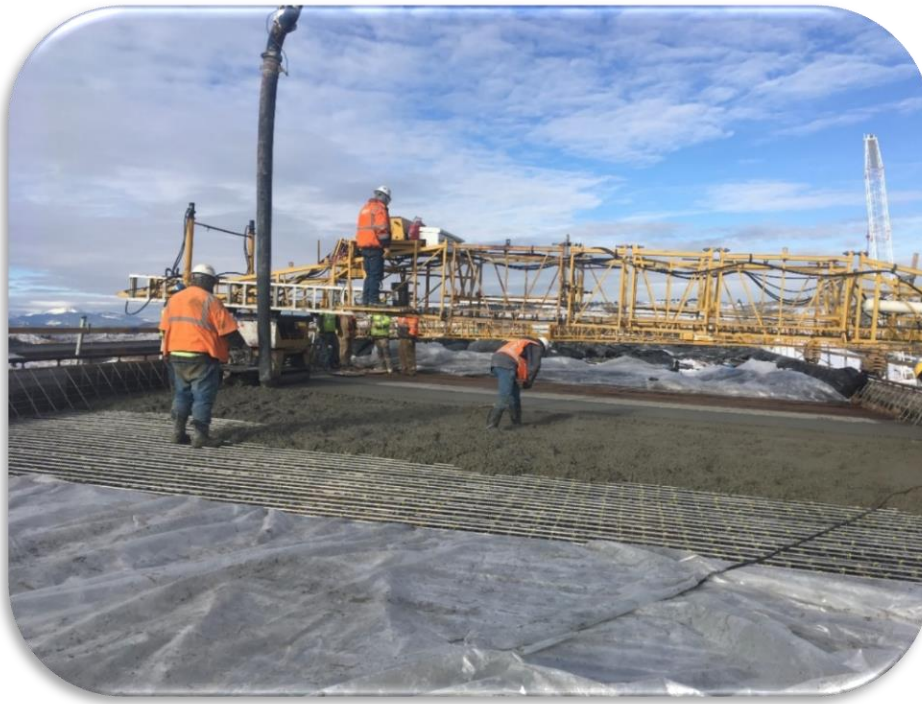
Figure 76. Concrete placement, finishing, and curing procedures.
