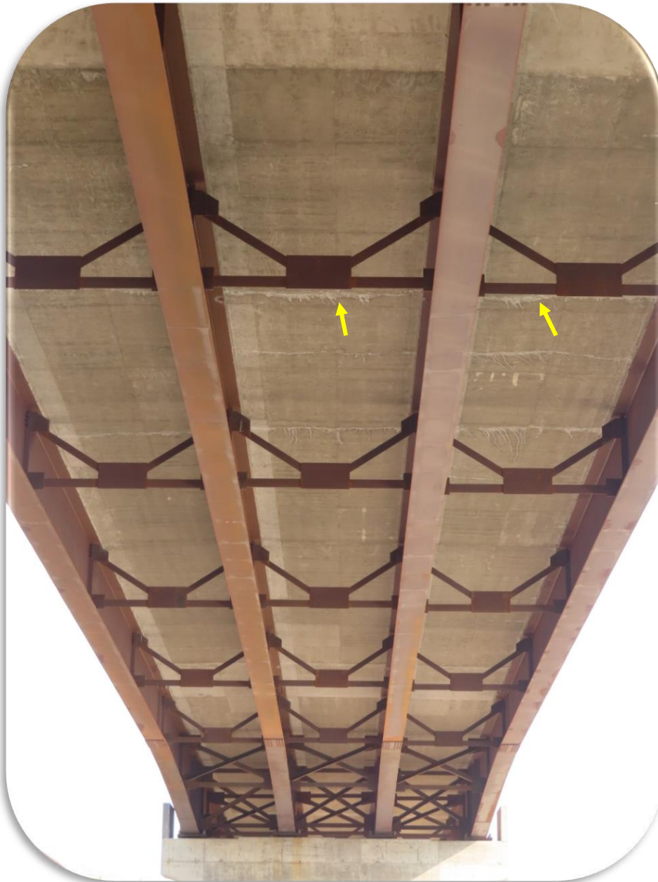
Figure 34. Bonner Bridge Phase I (EB) - 2020 inspection - Typical deck underside condition, placement 3.
