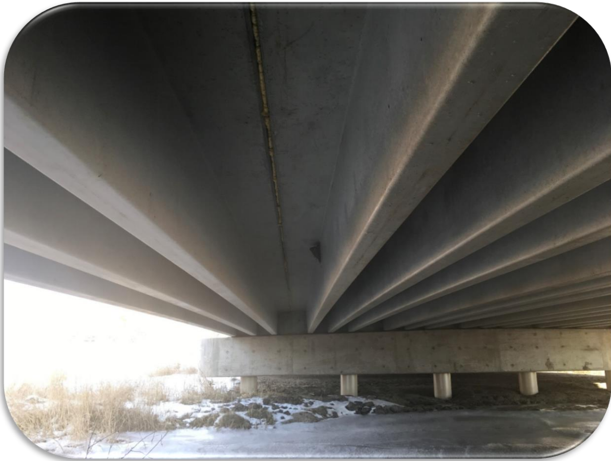
Figure 19. Whitehall Bridge - 2019 inspection - Typical deck underside condition.
