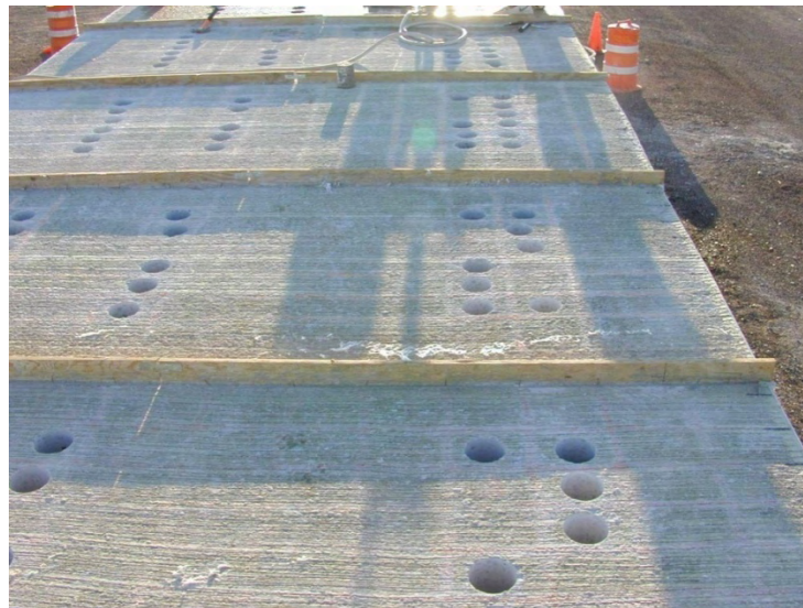
Figure 1.1 Coring of Bridge Deck Concrete for Permeability Test - El Paso Site
