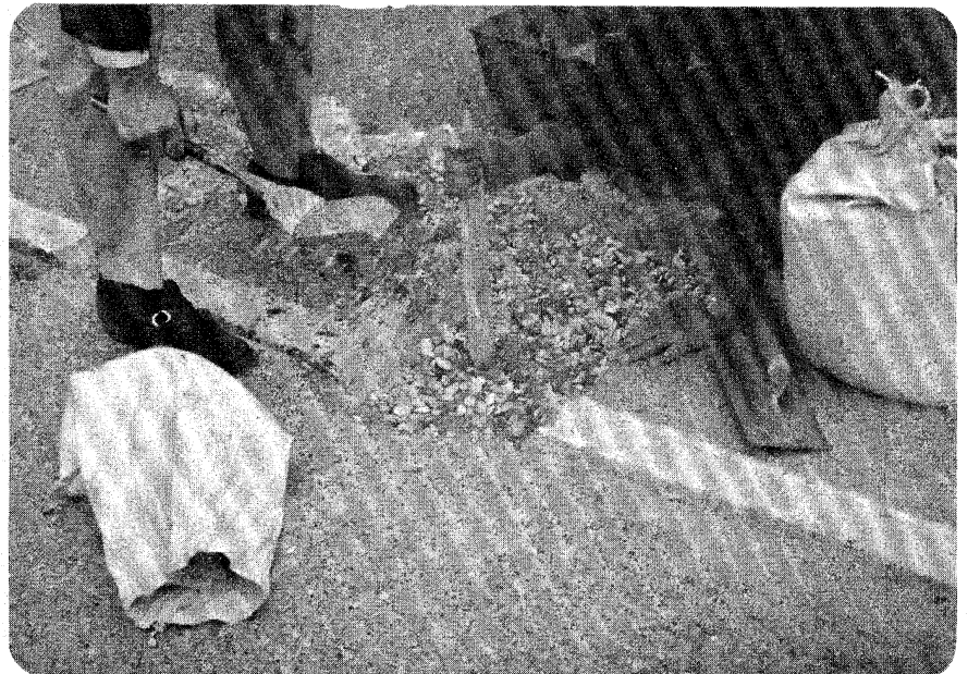
Figure 40. Placing fine aggregate.
