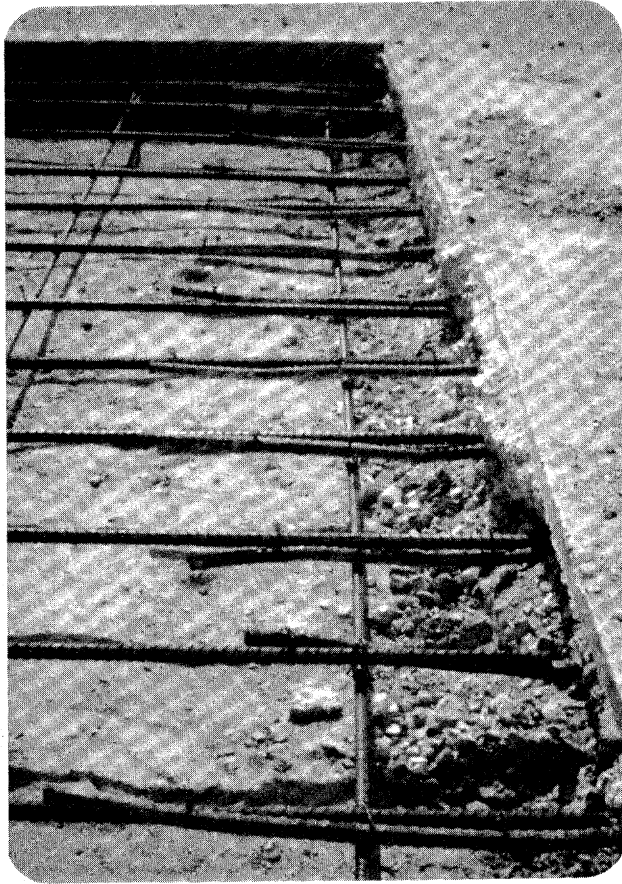
Figure 19. Typical tied steel splice.
