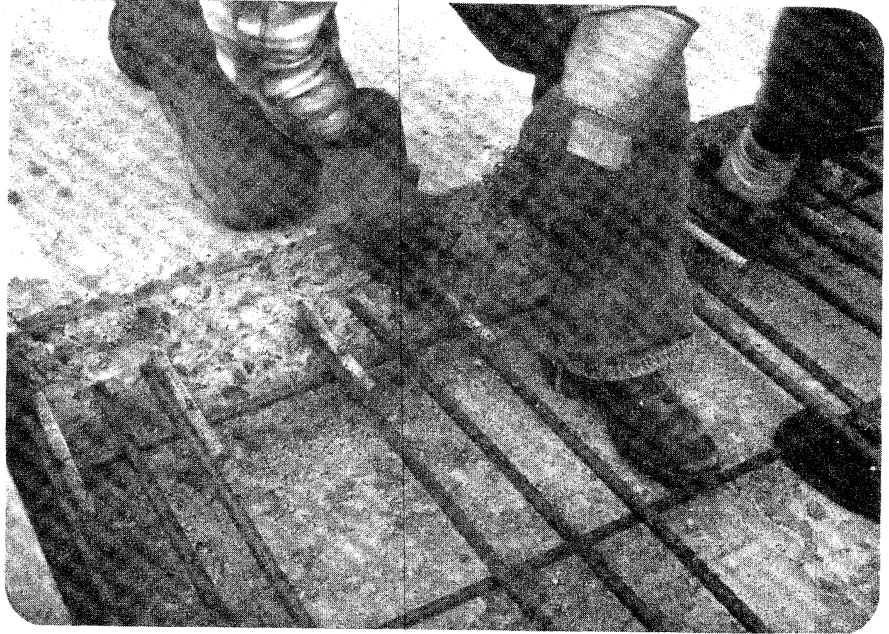
Figure 17. Tying steel for welding.
