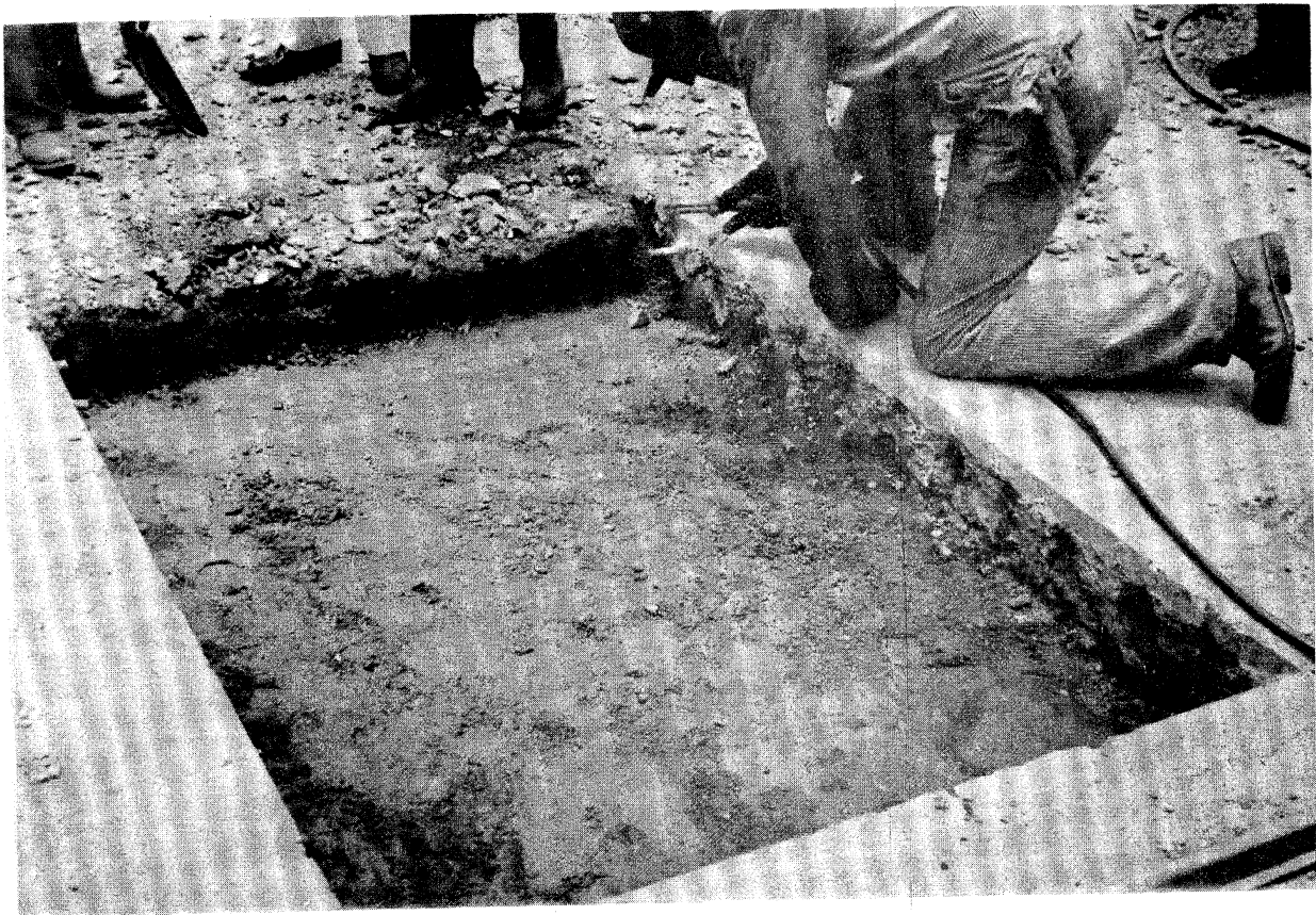
Figure 30. Preparing hole for precast patch.
