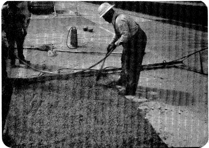
Figure 27. Vibrating the concrete.
