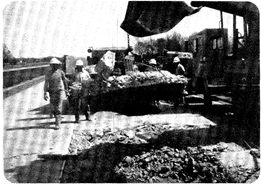
Figure 12. Lifting the slab.
