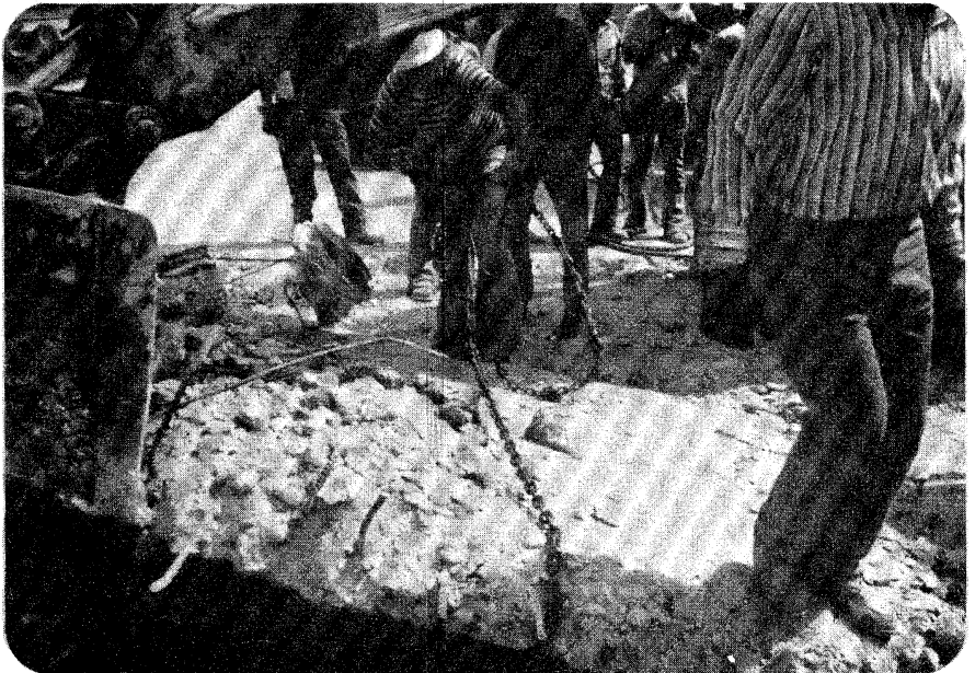
Figure 11. Putting a chain around the slab.
