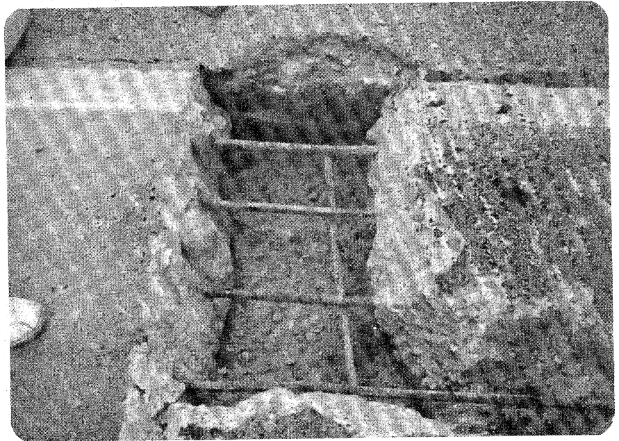
Figure 38. Hole prepared for polymer patch.
