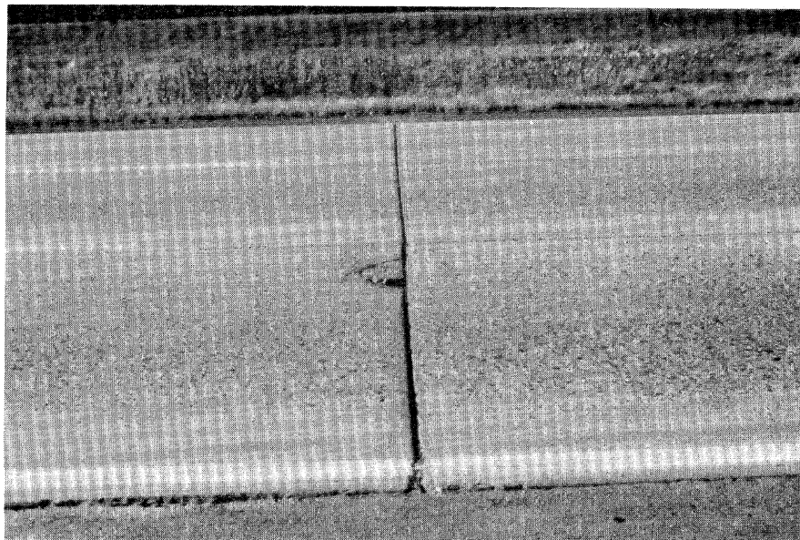
Figure 4.43. Low Severity Spalling.
