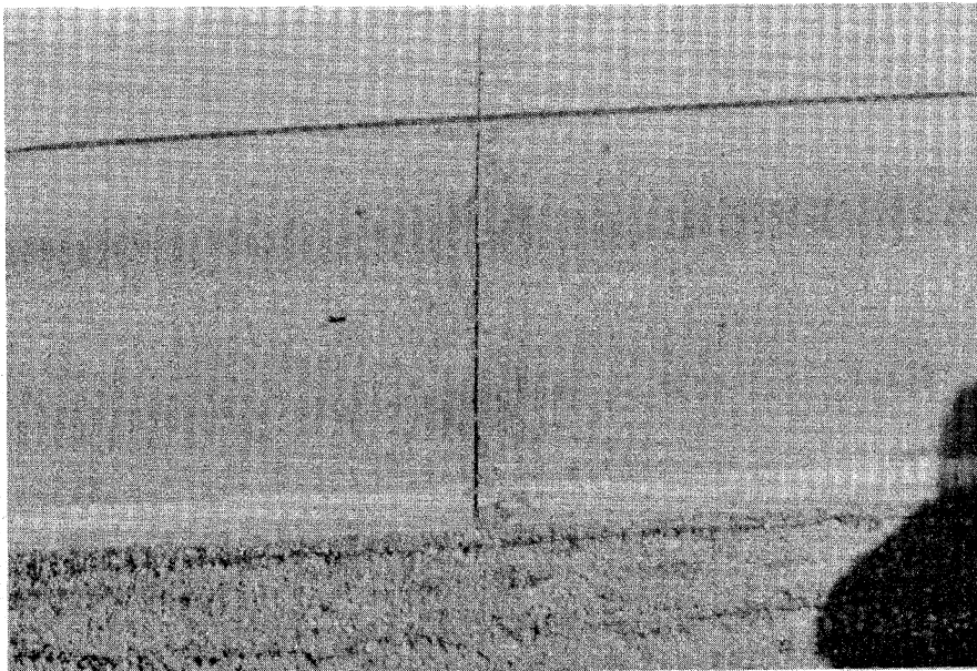
Figure 3.4. Low Severity "D" Cracking.
