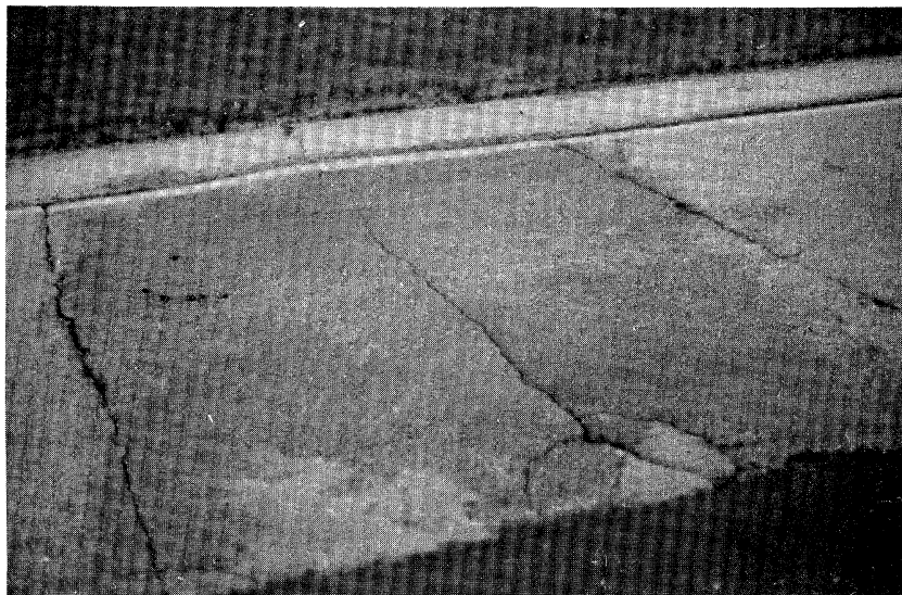
Figure 2.76. Medium Severity Swell Occurring at a Patch Due to Buckling of Concrete Slab Beneath Asphalt Surface.
