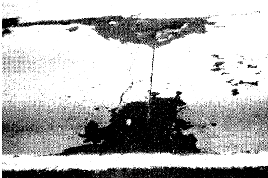
Figure 4.13. Medium Severity Joint Load Transfer System Associated Deterioration.
