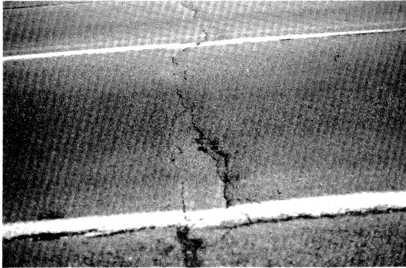
Figure 2.41. High Severity Transverse Cracking.
