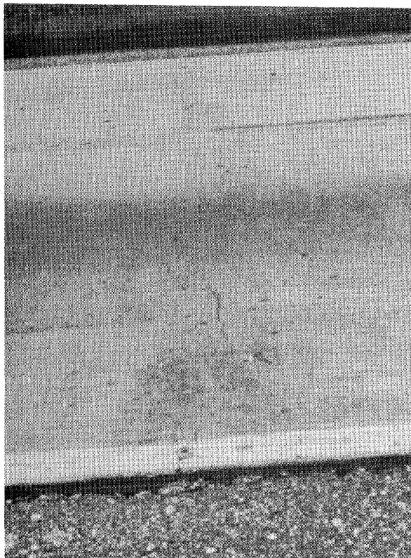
Figure 5.13. Low Severity "D" Cracking.
