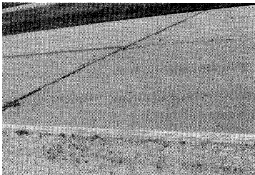
Figure 3.18. Gravel Shoulder Recorded as High Severity Lane/ Shoulder Separation.
