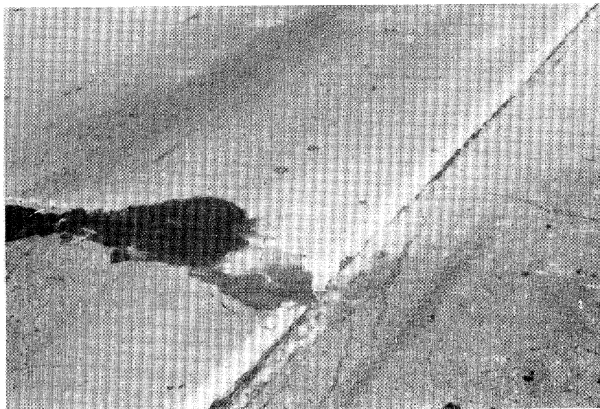
Figure 4.37. Medium Severity Pumping (pumped material like this occurs only at a few of the joints and cracks).
