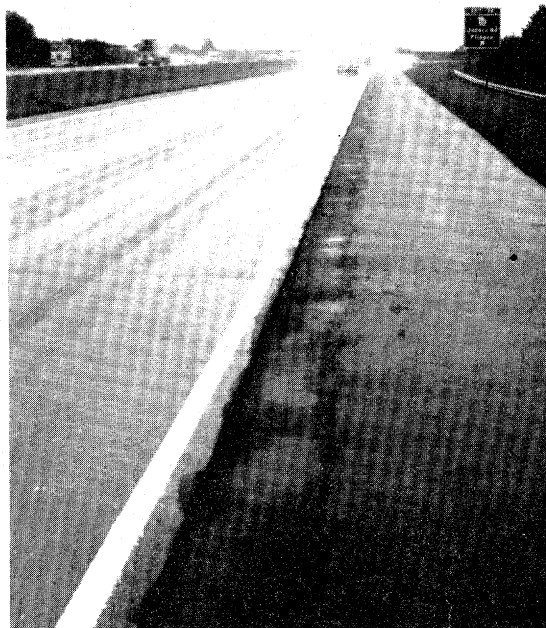
Figure 2.47. Low Severity Patch Along Shoulder Joint.
