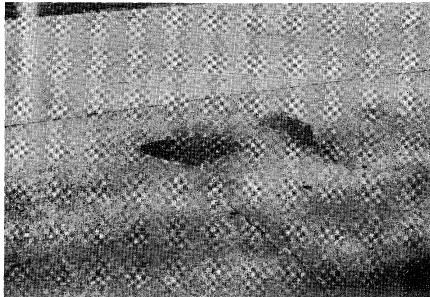
Figure 5.26. Medium Severity Localized Distress.
