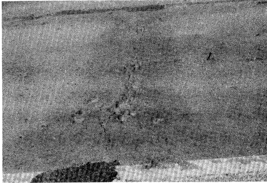
Figure 4.7. Medium Severity "D" Cracking.
