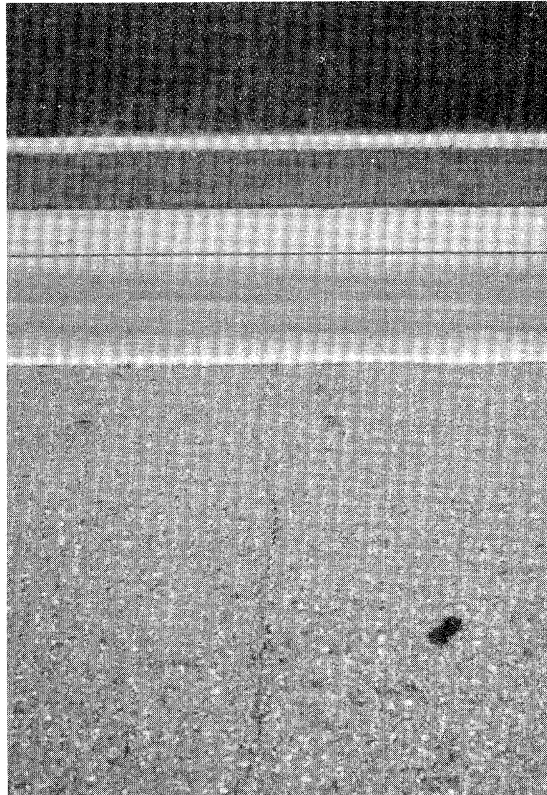
Figure 2.35. Low Severity Transverse Cracking Across Shoulder.
