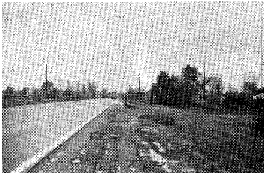
Figure 2.69. High Severity Raveling and Weathering.
