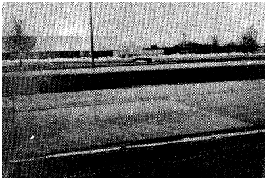
Figure 3.22. Low Severity PCC Patch Deterioration.
