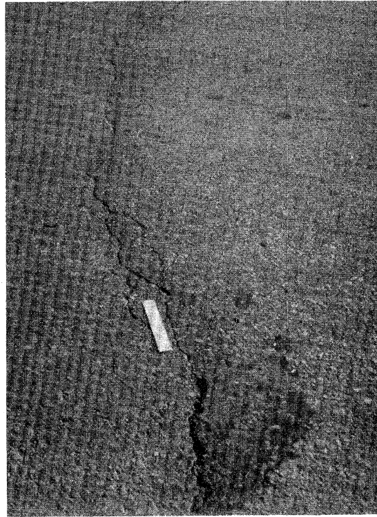
Figure 2.39. Medium Severity Transverse Cracking.
