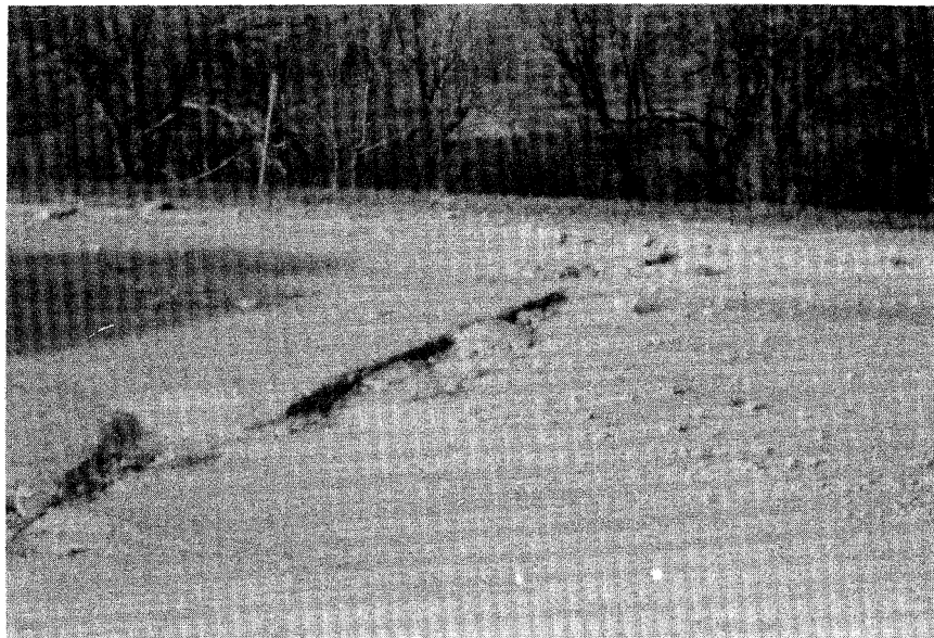
Figure 4.2. High Severity Shattering Type Blow-up.
