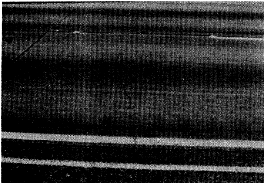
Figure 3.48. Low Severity Transverse Crack.
