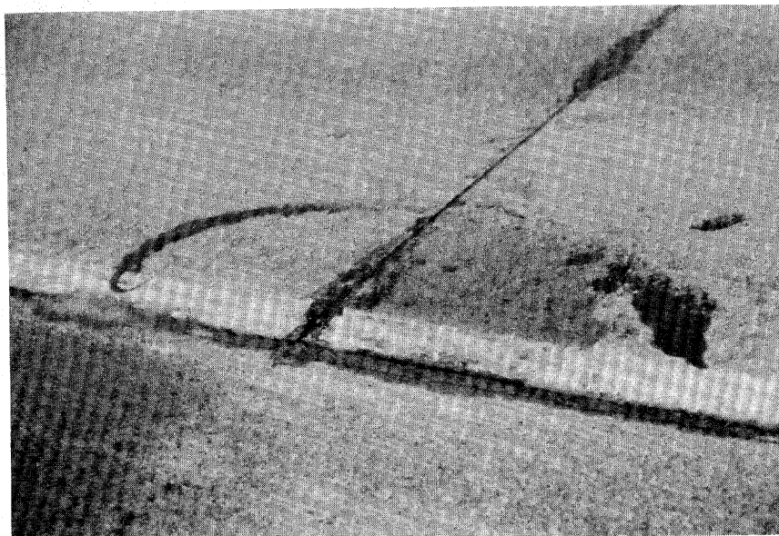
Figure 4.3. Low Severity Corner Break.
