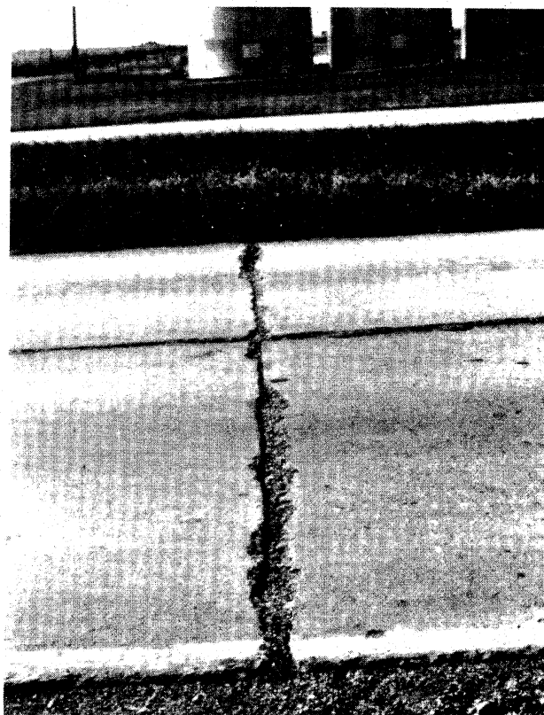
Figure 3.40. Medium Severity Spalling (Transverse Joint).
