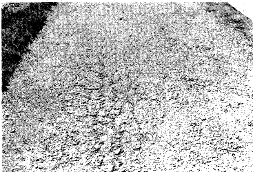
Figure 2.66. Medium Severity Raveling and Weathering.
