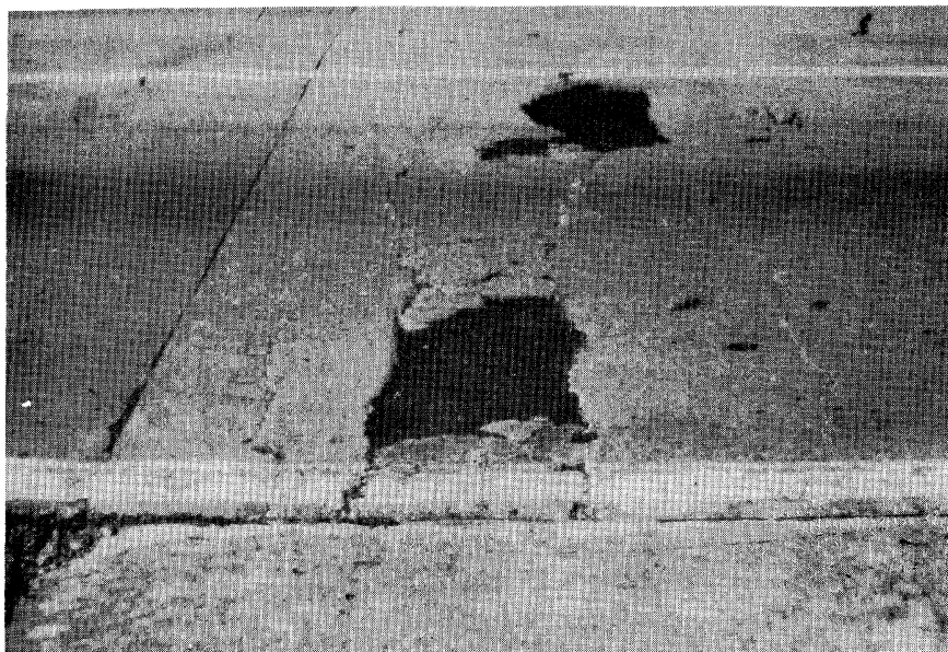
Figure 5.10. High Severity Construction Joint Deterioration.
