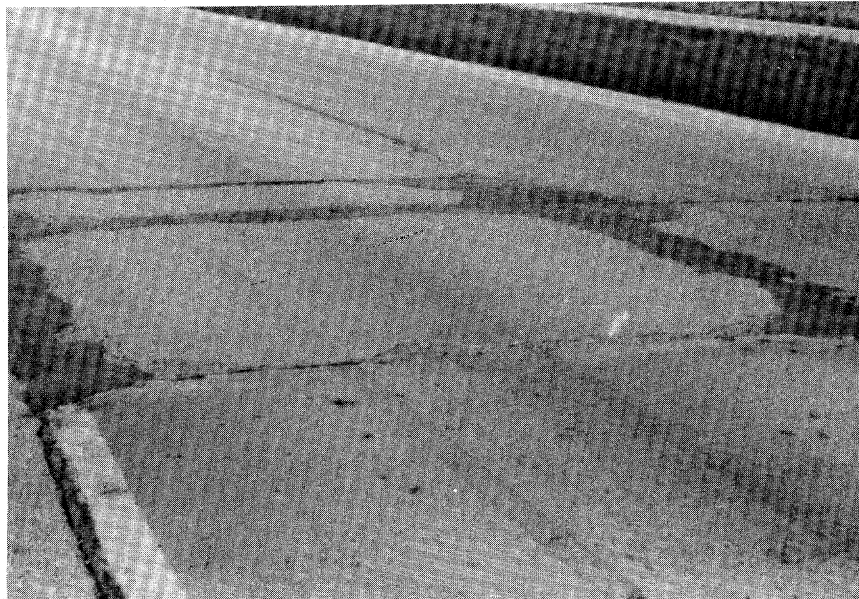
Figure 4.30 Medium Severity Concrete Patch Deterioration.
