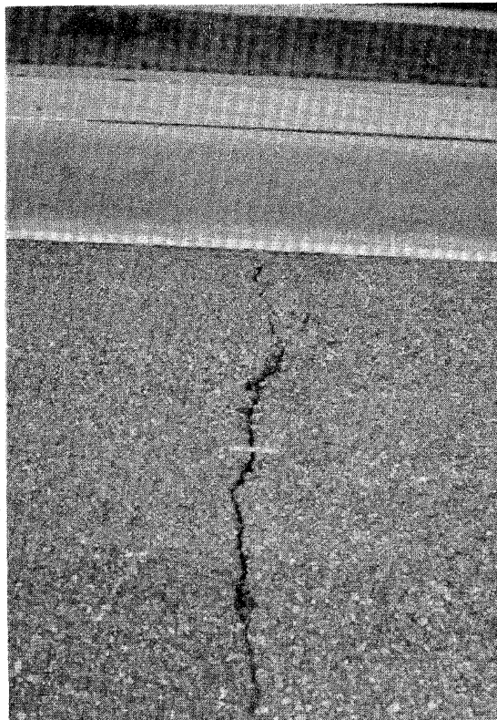
Figure 2.40. Medium Severity Transverse Cracking Across Shoulder.
