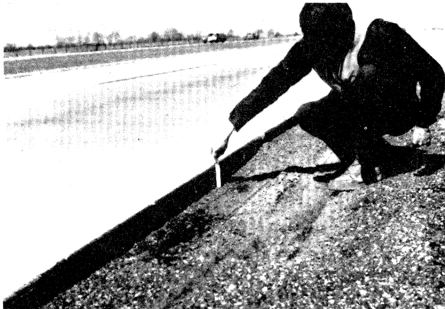
Figure 5.22. High Severity Lane/Shoulder Dropoff.
