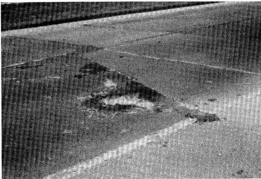
Figure 4.34. Patch Adjacent Slab Deterioration (second patch, spalling, "D" cracking and temporary patching).
