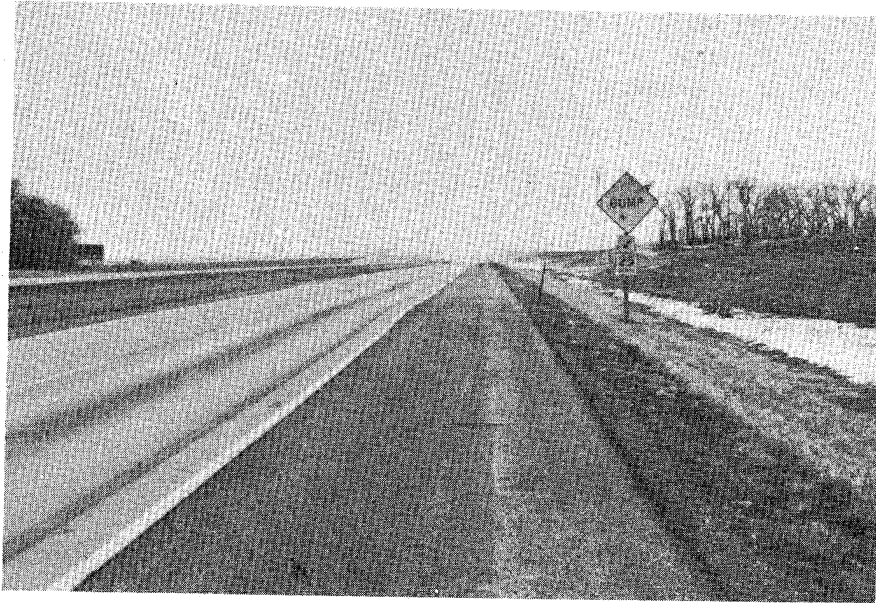
Figure 5.54. Swell Caused by Frost Heave.
